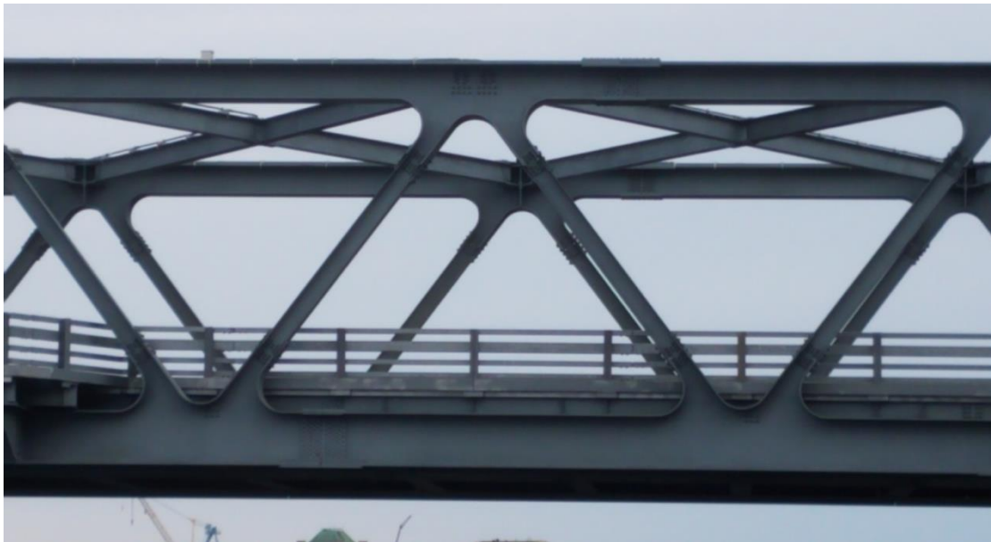
Figure 1 - Gusset-less Connections at the Memorial Bridge, Portsmouth NH
