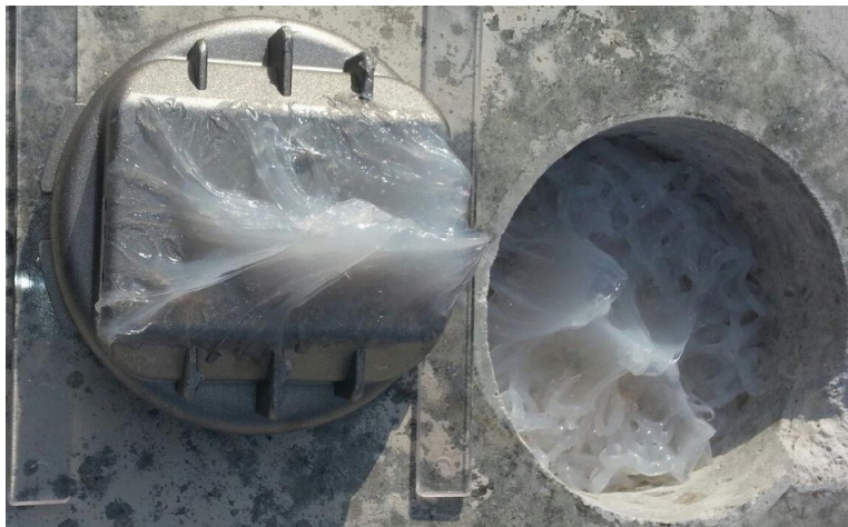
Example of Solar Delineator Installation
