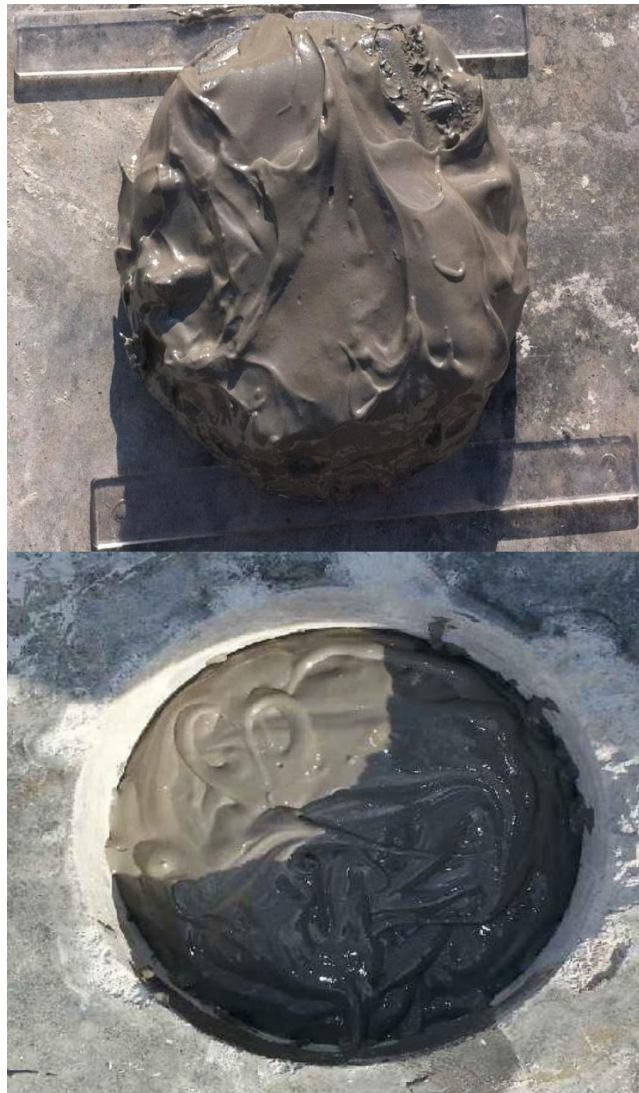
Figure A.3: Picture of Full Depth Epoxy Coverage of Delineator
