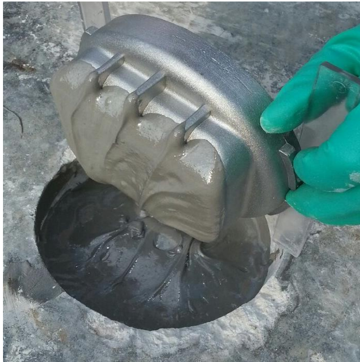
Figure A.2: Method 2 Picture of Epoxy Base Coverage
