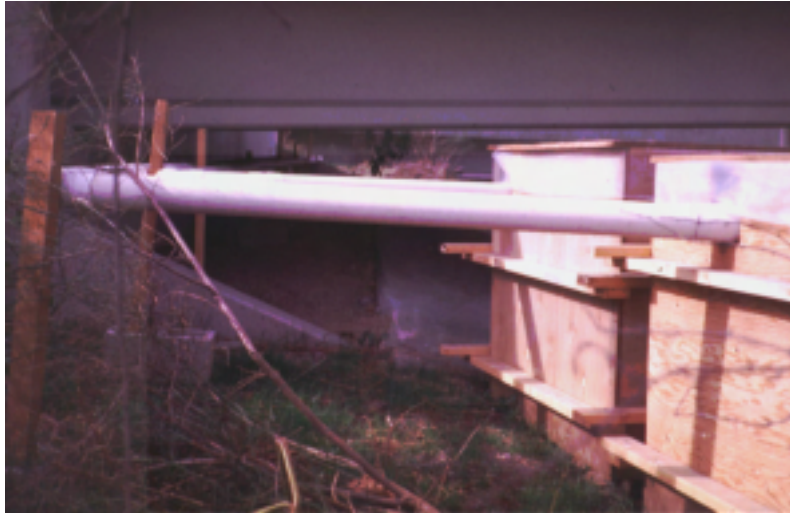
Figure 3.7 Storm water conveyance lines and collection tanks
