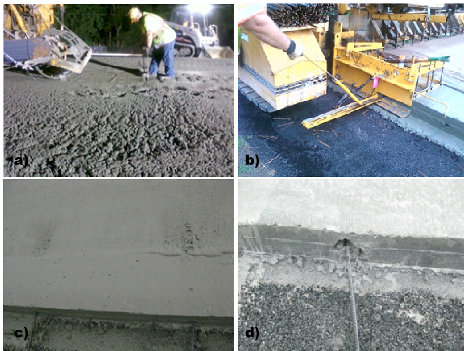
Figure 14. Tie Bar Placement in Unbonded Section: a) insertion in middle of lanes; b) insertion at edges; c) surface disturbance; d) hole at edge
