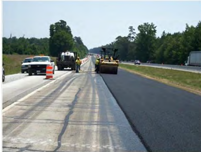
Figure 10. Porous Friction Course As Separation Layer for Unbonded Section
