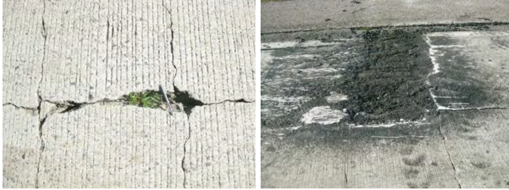
Figure 2. Visual Distress Observed on Unbonded Section Before Construction
