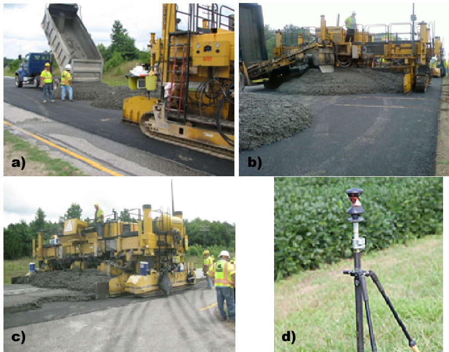
Figure 13. Paving Operation: a) trucks dumping concrete in front of spreader; b) side discharge; c) two-track paver; d) GPS-enabled laser guidance system
