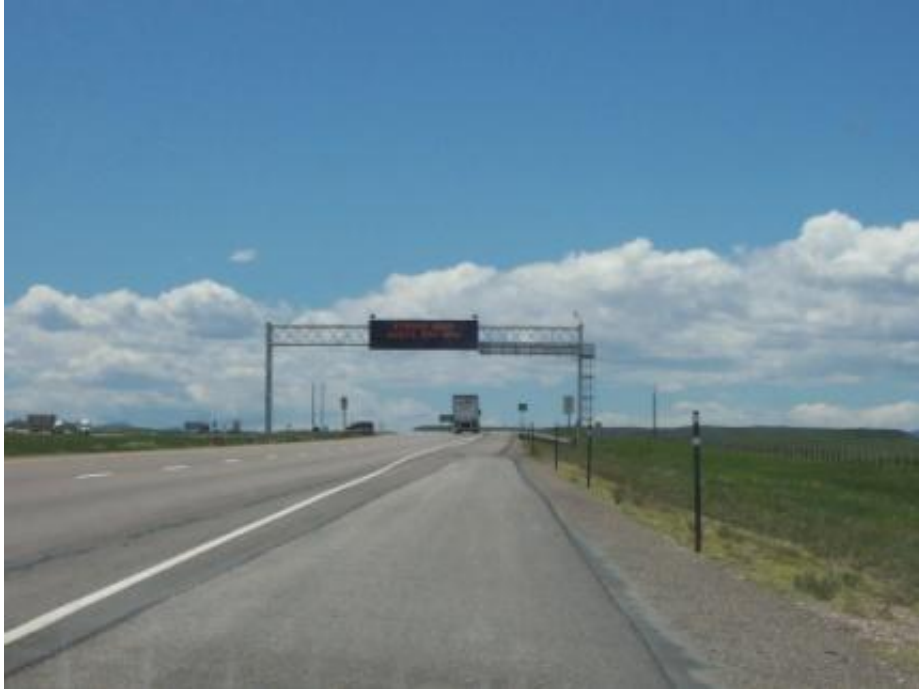
Figure 3.6 Three Line, Overhead Mounted DMS on I-80
