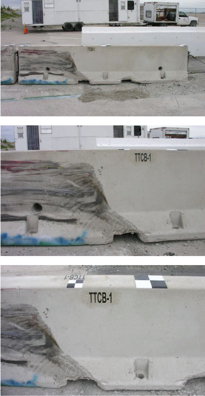
Figure 34. System Damage - Barrier No. 1, Test No. TTCB-1
