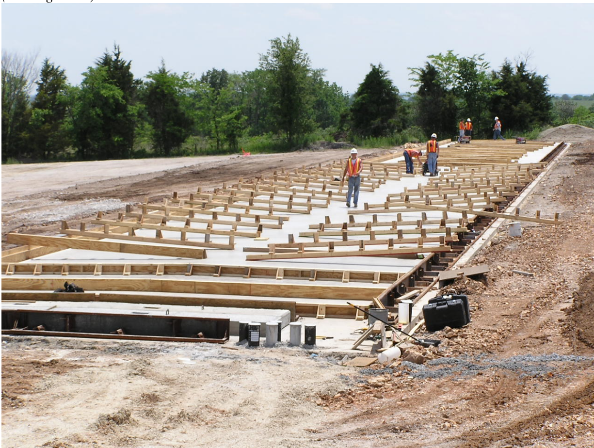
Figure 2: Casting bed – laying out forms for 10 ft. sections.
