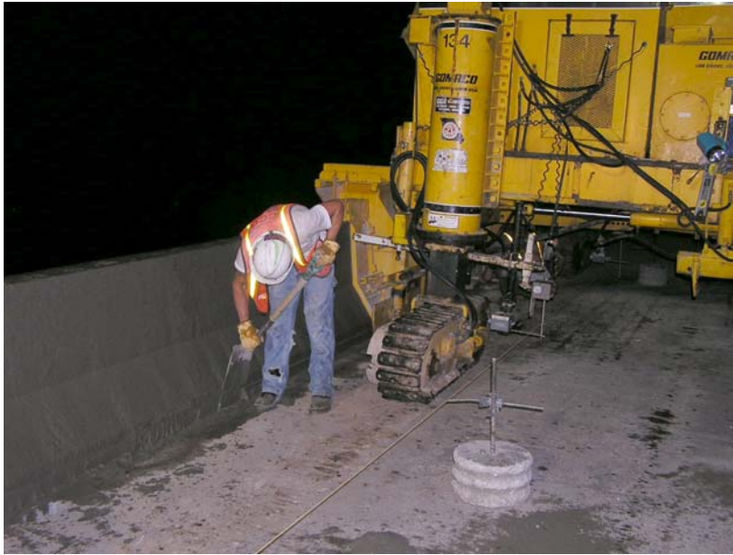
Figure 17: Placing barrier curb by slipform method.
