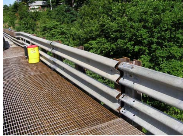
Figure 10: (In background) Temporary guardrail transition to existing guardrail.
