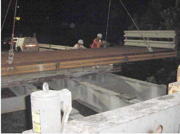
Figure 9: Installing temporary deck panels.
