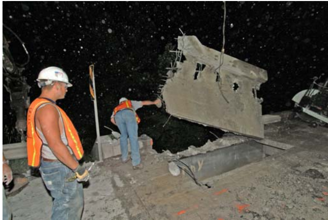
Figure 7: Removing first section of old concrete deck.
