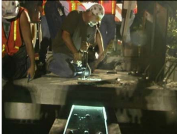
Figure 12: Welding new shear studs to steel girder through blockout.
