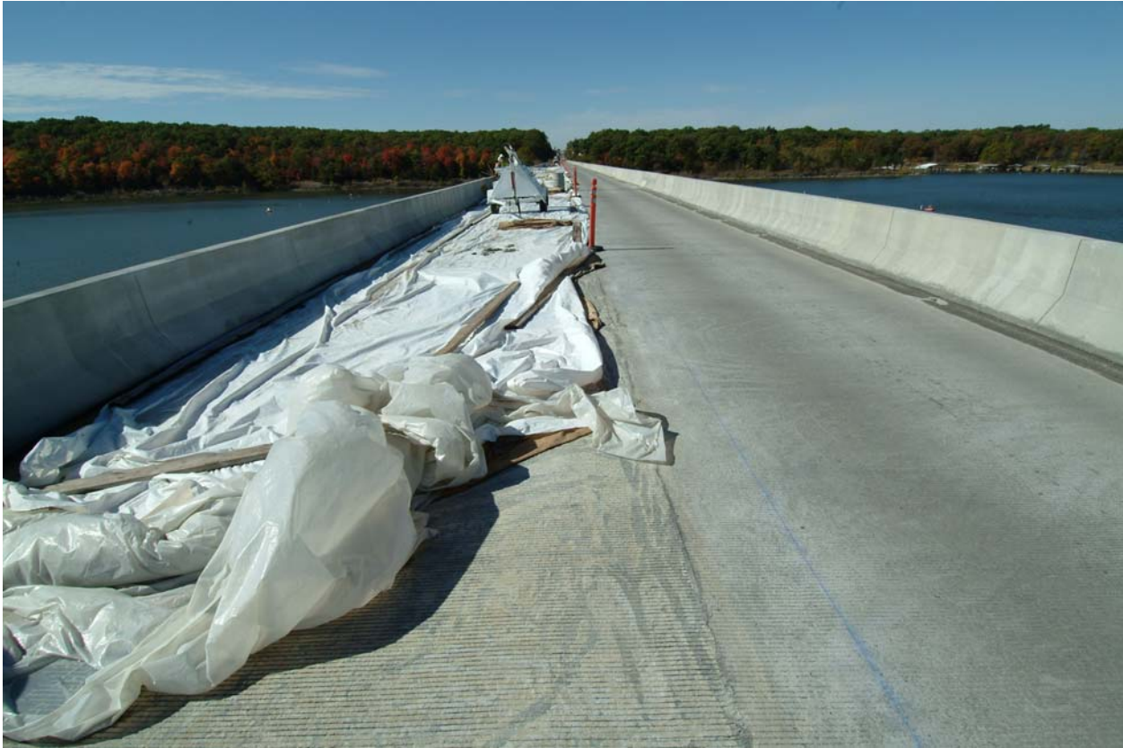
Figure 18: Uncovering the last of silica fume overlay placements.
