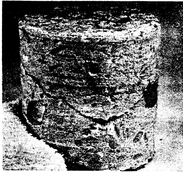
Figure 20. Core taken from a mediumly delaminated spot in square 2-6 of Figure 12. shows no corrosion at one end of the steel
