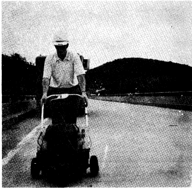
Figure 7. Delamination detector in operation.
