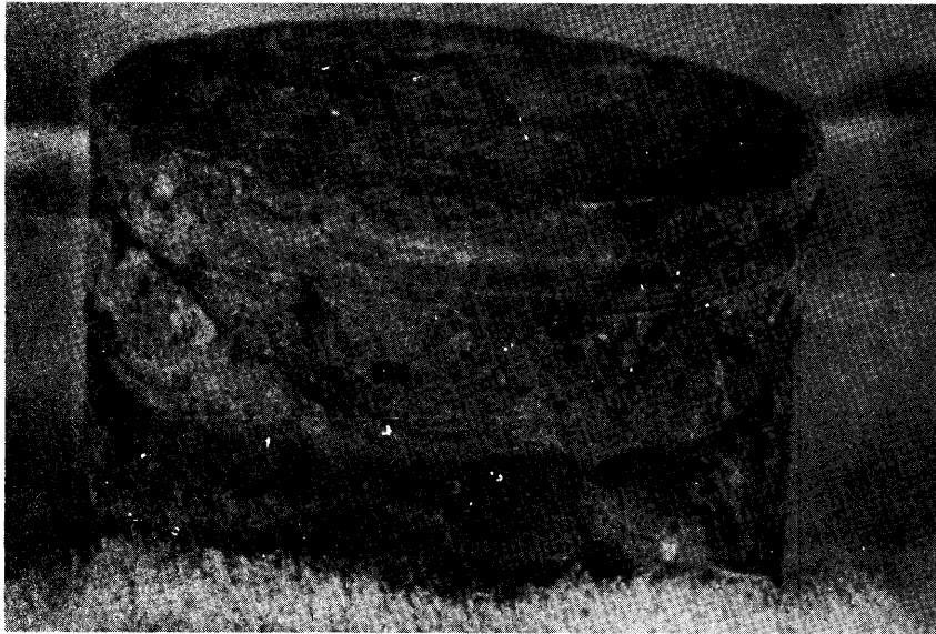
Figure 26. A core from a delaminated spot in square 3-8 in Figure 13.
