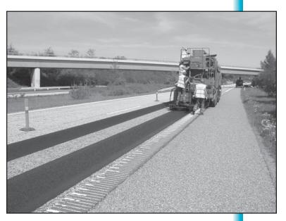
Figure 4. Replacing hot-mix asphalt in wheel paths in Denmark. (Photo source: Danish Road Institute, Denmark)
