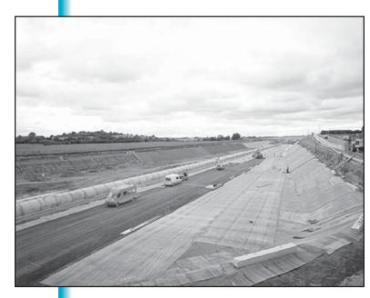
Figure 5. Demonstration of bituminous membrane application in Denmark. (Photo source: Colas Danmark A/S, Denmark)
