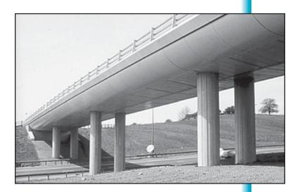
Figure 31. External enclosure of bridges in the United Kingdom. (Photo Source: Highways Agency, UK)
