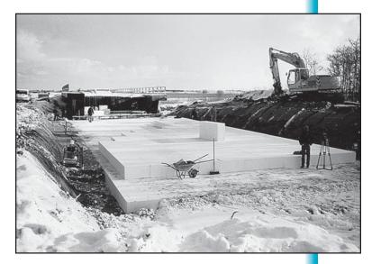
Figure 9. Geofoam application in Germany. (Photo Source: BASt, Germany)
