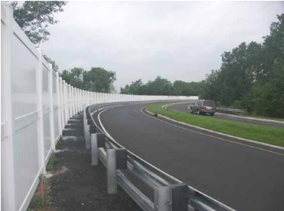
Figure 13 8ft High Privacy Fence for Route 138 & 18 Intersection
