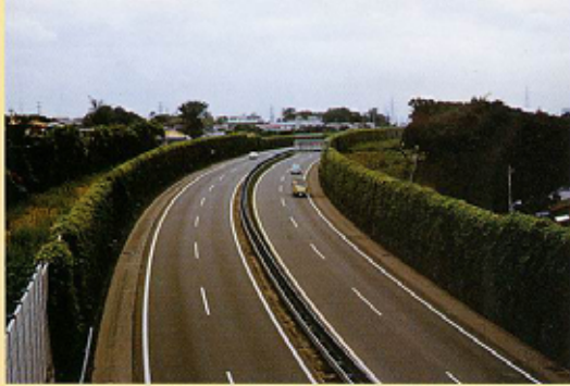
Photo 1 The road landscape is much improved by noise barriers covered with ivy. It also reduces the sense of discomfort given to the surrounding area.(Chuo Expressway)
