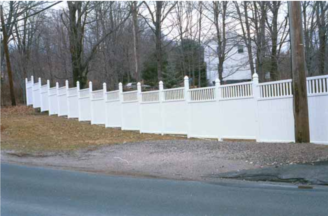
Figure 1 Six Foot PVC Privacy Fence
