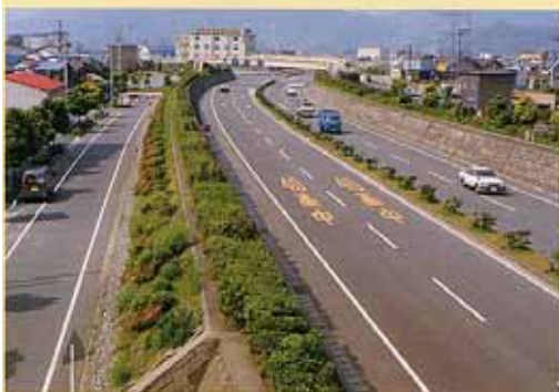
Photo 6 A comfortable roadside environment and driving environment are possible by building embankments if there is a sufficient width for buffer zones. (Seishin Bypass, National Highway No.1)
