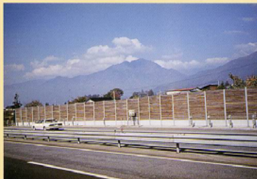
Photo 4 Use of wooden noise barriers in harmony with the surrounding landscape is peaceful for drivers.(Chuo Expressway)
