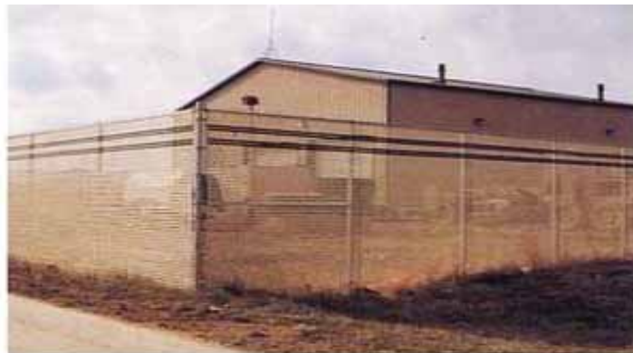
Horizontally installed DuraSlatt fillerstrips with contrasting feature strips
