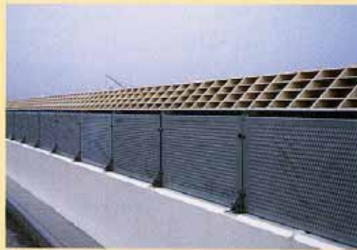
Photo 8 Phase difference is created by separating the sound wave to get a noise reducing effect by interference. Installation of the interference type special noise barrier protects sunshine against deterioration and reduces the sense of discomfort. (Kanagawa NO.3, Metropolitan Expressway)
