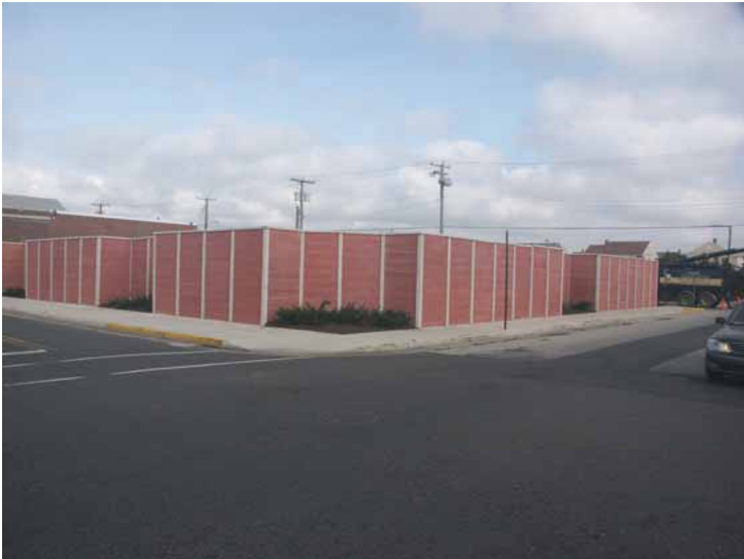
Figure 17 Concrete Privacy Fence
