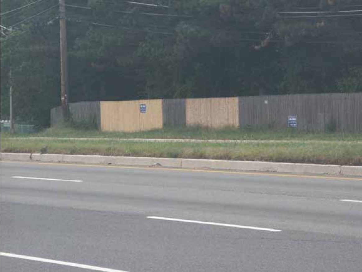
Figure 4 Repaired Sections Privacy Fence Along Route 9, Manalapan Twp.
