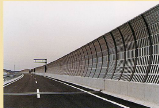
Photo 3 Use of curved noise barriers reduces the influence of reflected noise and gives a soft image to the structures.(New Shonan Bypass, National Highway NO.1)
