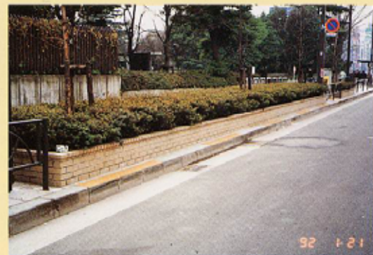
Photo 5 Noise barriers often cannot be installed in an area where roadsides are used for other purposes. In such places, planting tubs serve as noise barriers to some extent.
