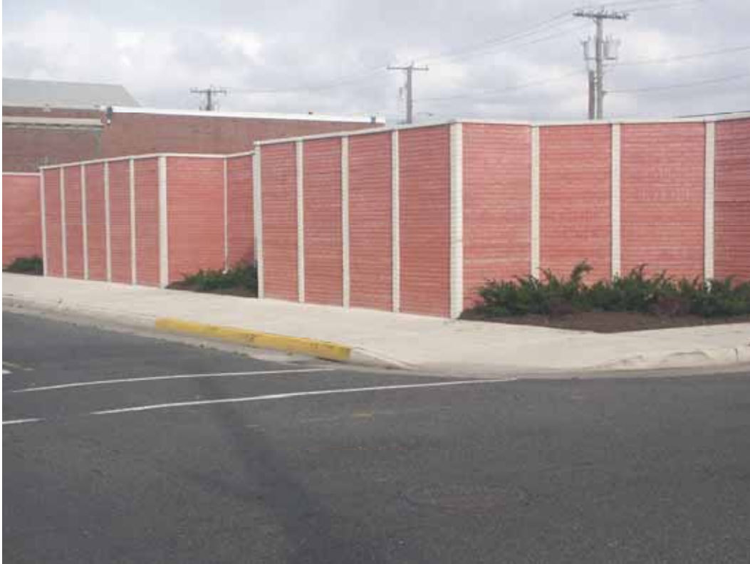
Figure 18 Concrete Privacy Fence
