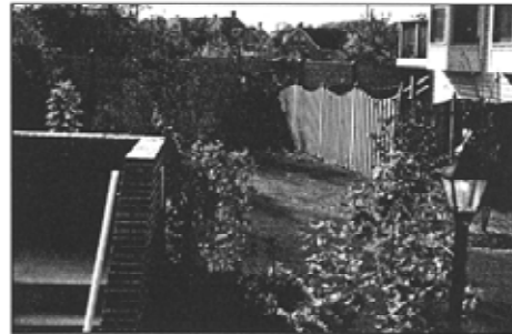
This bottling plant had received noise complaints from nearby homes. The complaints stopped after installation of this 15-foot high PLYWALL barrier
