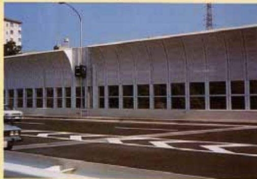
Photo 10 The translucent plate is provided at the height of the drivers' eyes to protect the landscape. The upper part overhangs to protect against reflected noise. (Kanagawa NO.3, Metropolitan Expressway)
