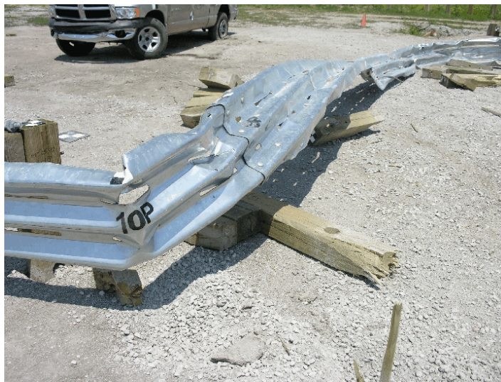
Figure 45. System Damage, Test SR-7
