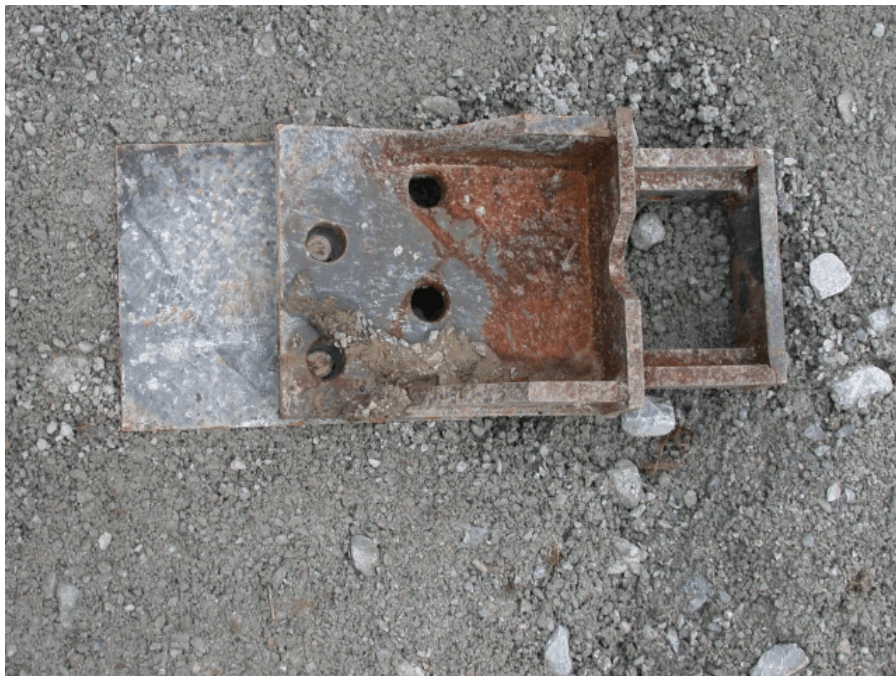
Figure 55. Cable Anchor Damage, Test SR-5
