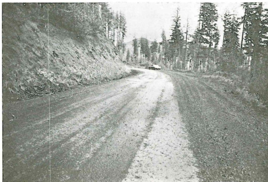
Figure 21. Bald Mountain Access Road, October 1973.
