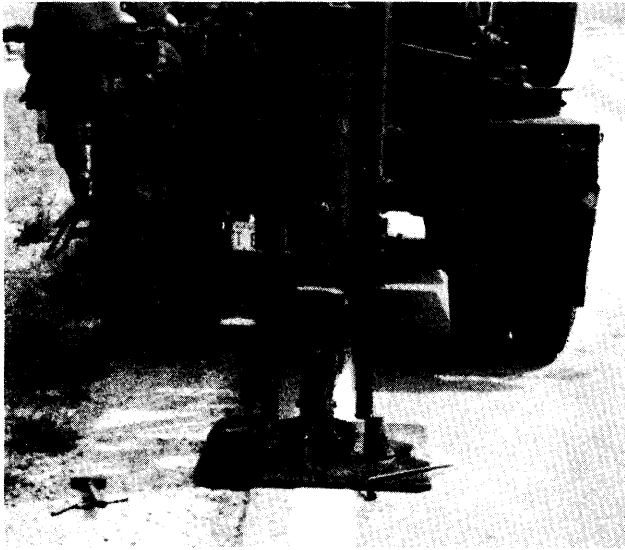
Figure 22. Equipment used to punch holes for light installation and the hole punched.
