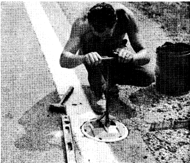
Figure 23. Pavement light being set and being aimed with a stringline.
