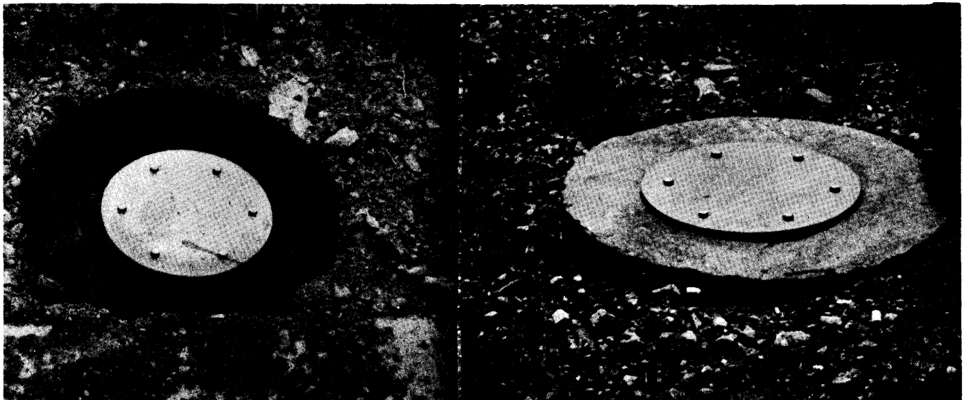
Figure 13. Transformer housing before and after concrete was poured.
