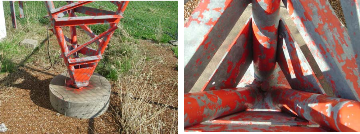
Figure 2.13. Details of Ashland foundation and shear pin.
