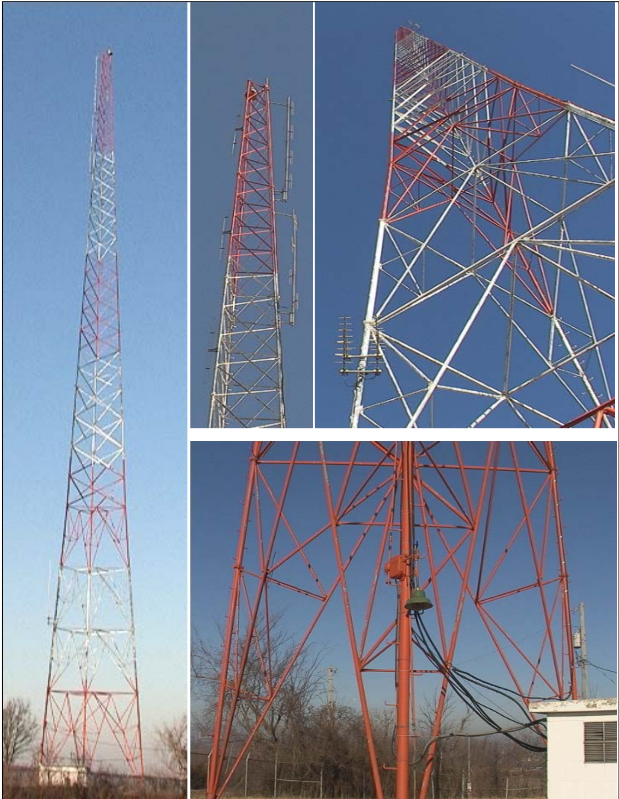
Figure 3.40. (a) Select Photographs of Kansas City Tower
