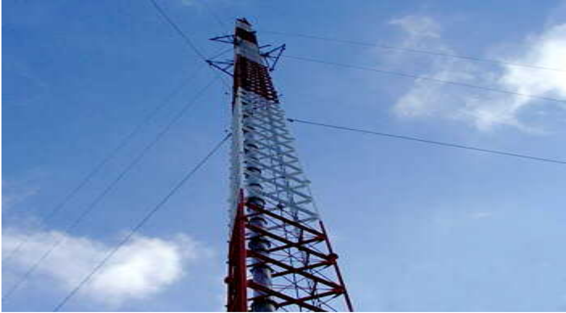
Figure 3.2. Example of a typical guyed mast tower.
