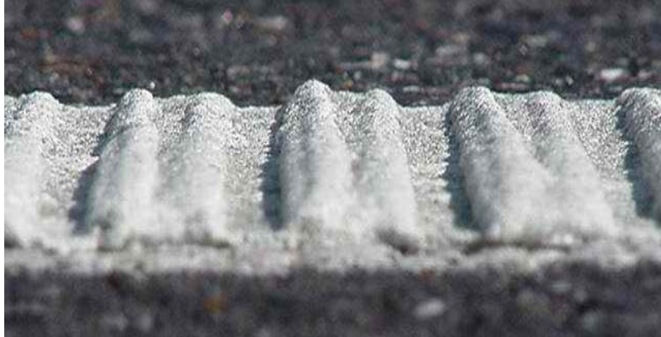
Figure 3-3. Profiled pavement marking
