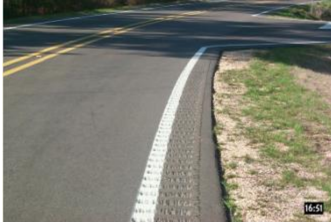
Figure 9-1. Rumble stripe on SR 589 in Mississippi
