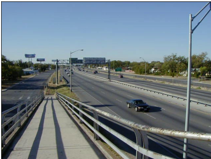
FIGURE 3-23 IH-35 South of the Second Pedestrian Overpass
