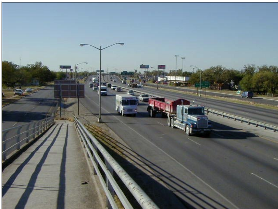
FIGURE 3-25 IH-35 South of the Third Pedestrian Overpass
