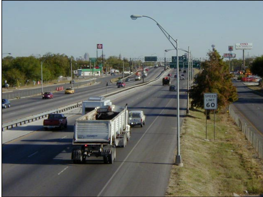
FIGURE 3-22 IH-35 North of the First Pedestrian Overpass
