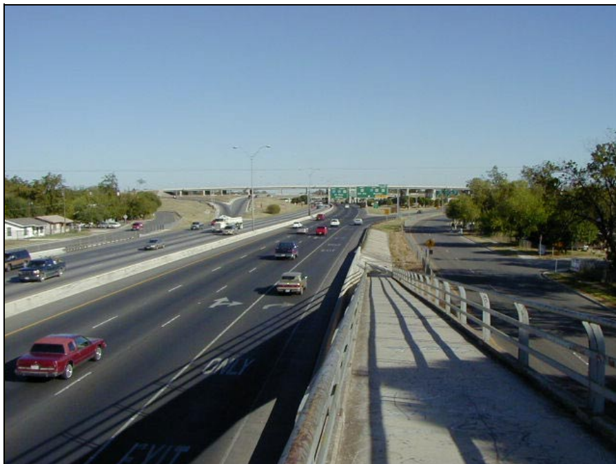
FIGURE 3-29 IH-35 North of the Fourth Pedestrian Overpass
