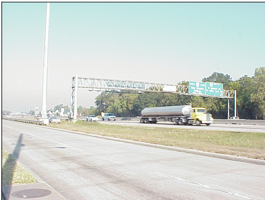
FIGURE 3-13 US 290 at the Third AVI Reader Taken to the West
