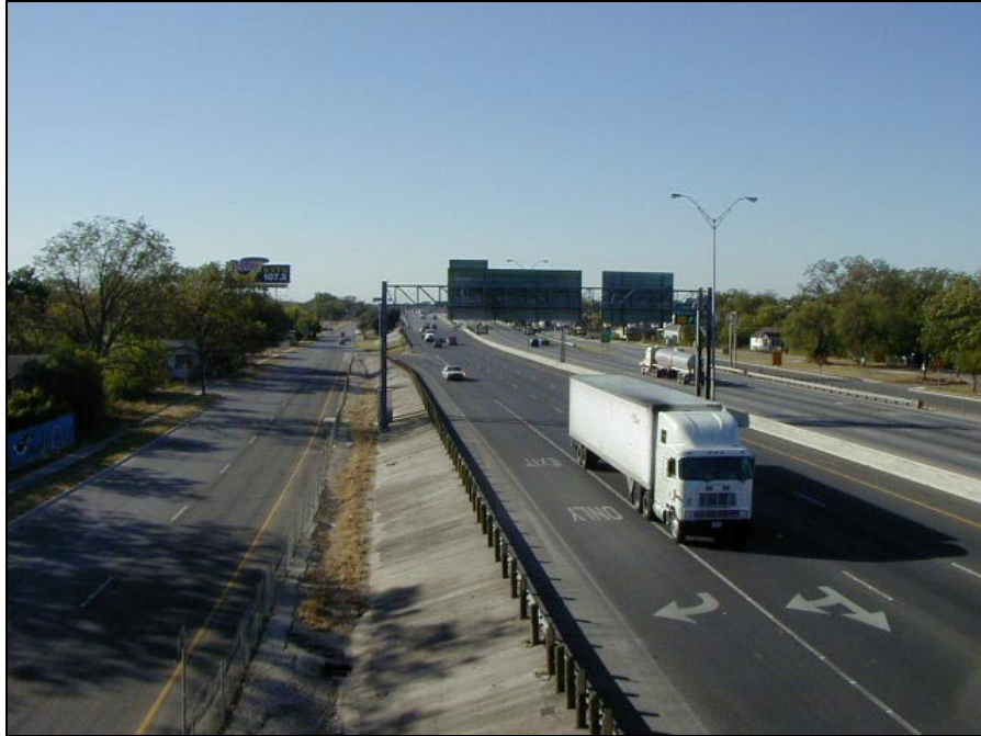
FIGURE 3-28 IH-35 South of the Fourth Pedestrian Overpass
