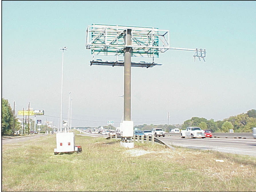
FIGURE 3-18 US 290 Taken Looking West Showing the Fifth AVI Station
