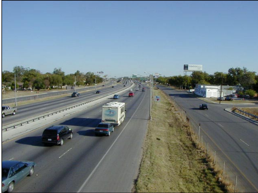
FIGURE 3-24 IH-35 North of the Second Pedestrian Overpass
