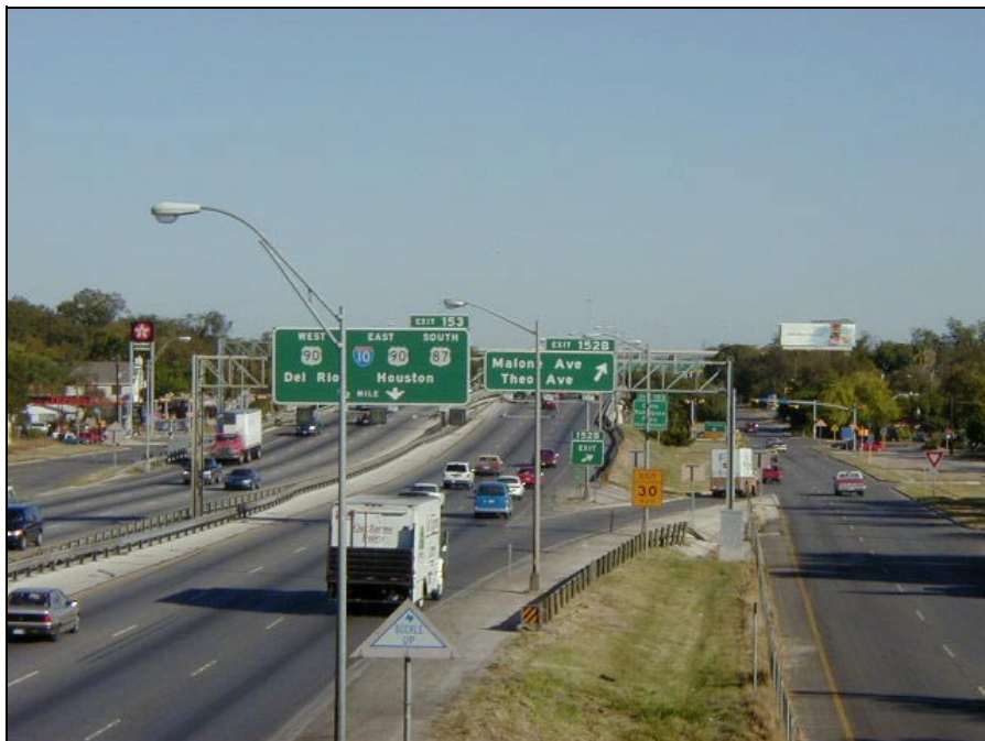
FIGURE 3-27 IH-35 North of the Third Pedestrian Overpass Showing the Malone Exit
