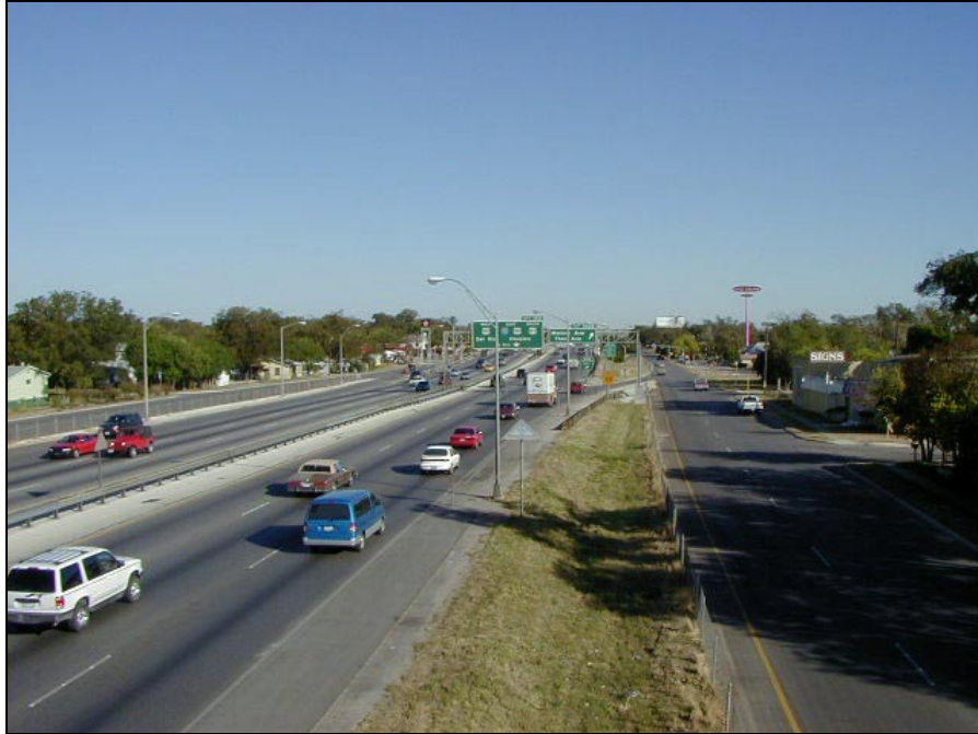
FIGURE 3-26 IH-35 North of the Third Pedestrian Overpass
