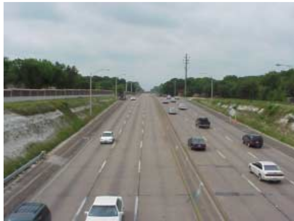
Figure 31. Dallas North Tollway at Meaders Lane (northbound lanes).
