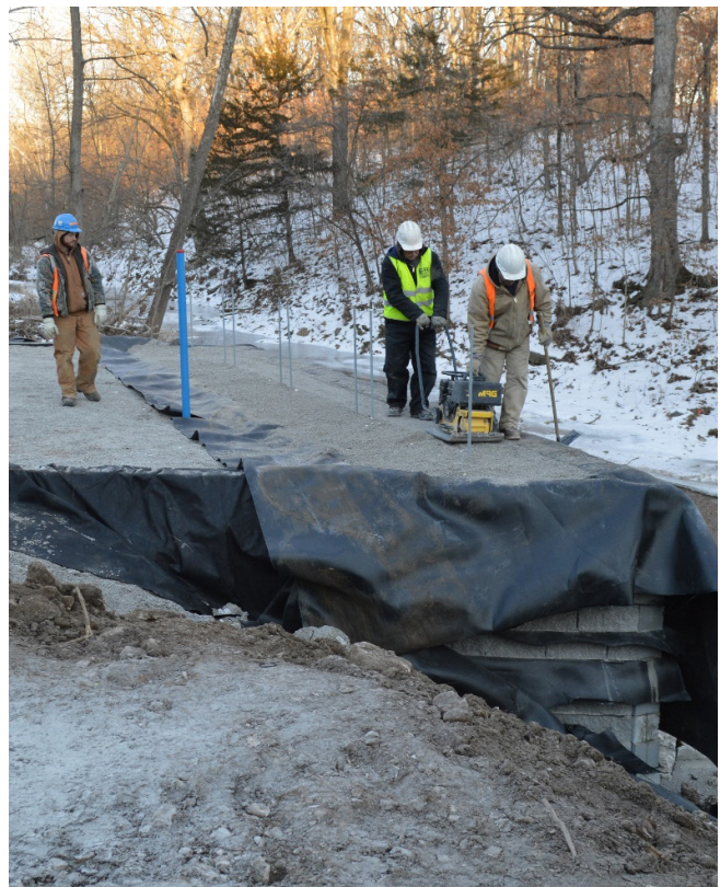
Compaction of second layer of beam seat
