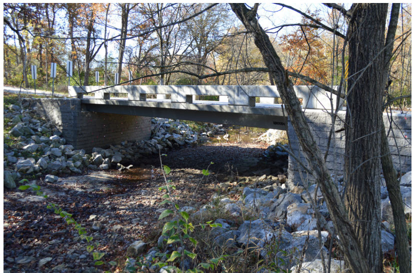
Completed Rustic Road GRS-IBS from the northeast
