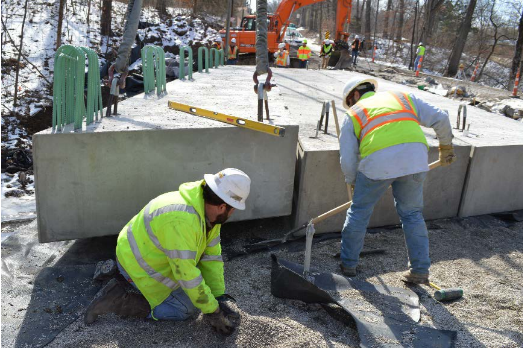
Figure 32. Crew places additional aggregate below first girder to achieve level surface
