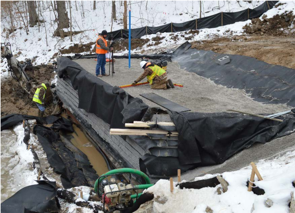
Figure 22. Surveying and leveling to place anchor plates for girders
