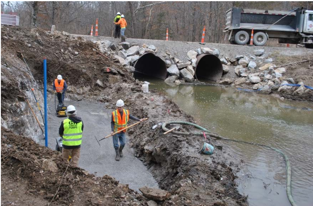
Figure 9. Compaction of reinforced soil foundation for south abutment
