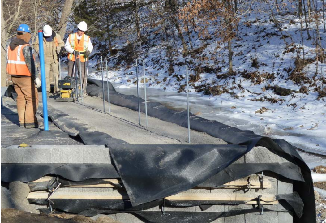
Figure 26. Compaction of first layer of beam seat for north abutment
