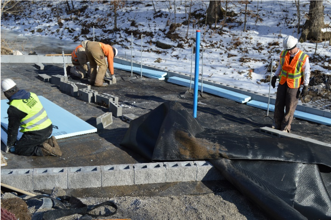
Figure 24. Preparation of the beam seat for north abutment
