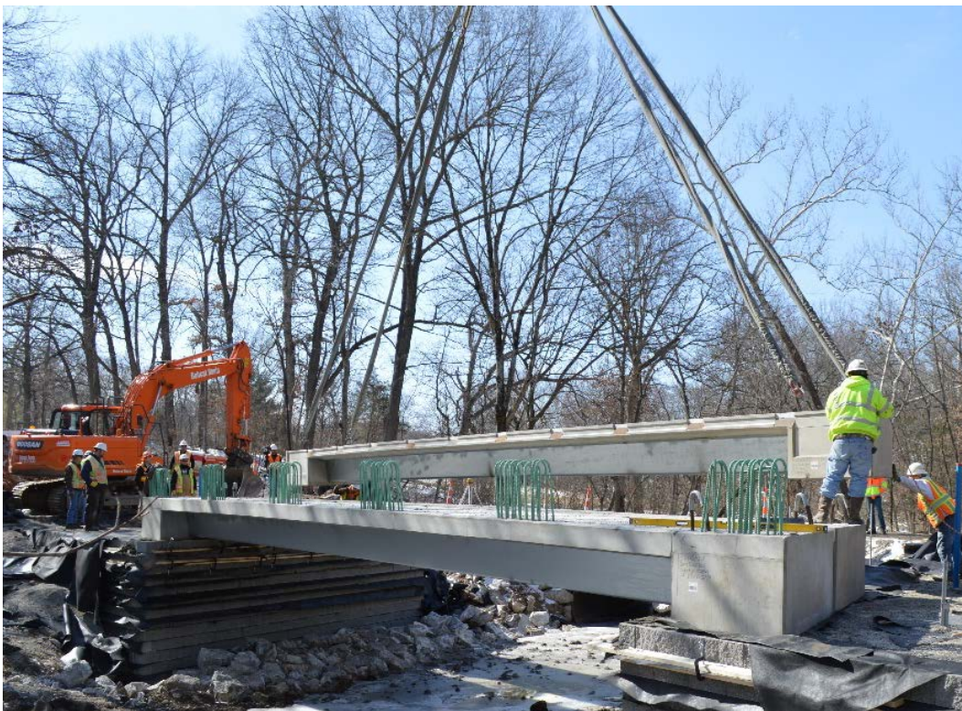
Figure 31. Placement of third girder
