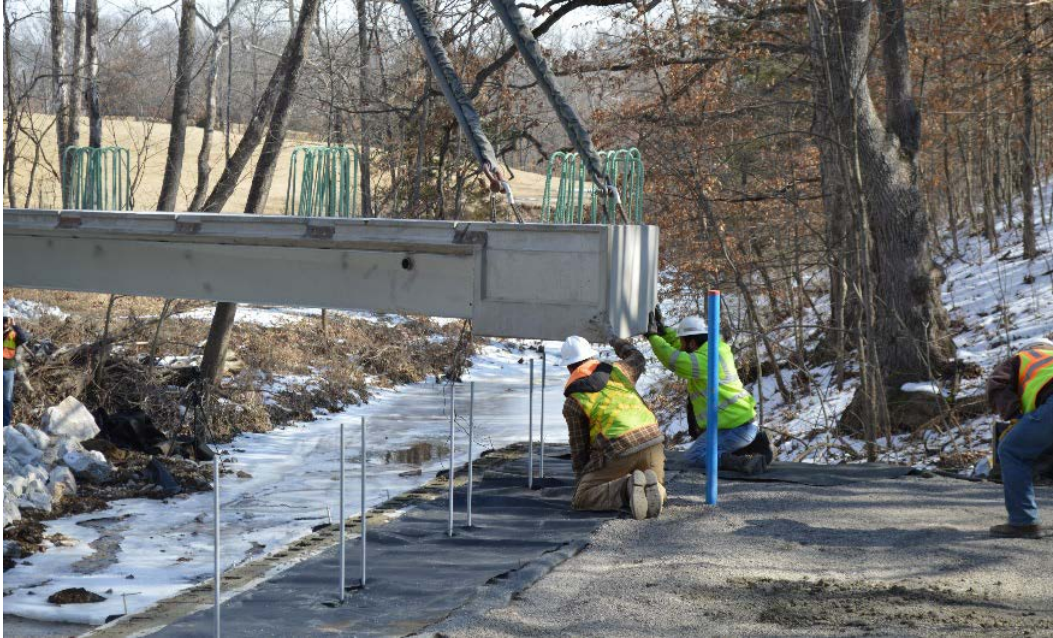
Figure 30. First girder being lowered into place
