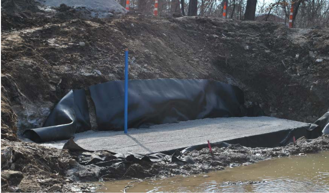
Figure 14. Completed third course of south abutment
