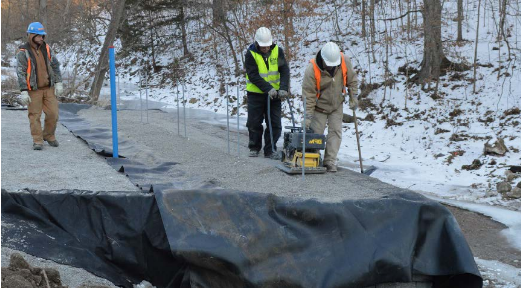
Figure 28. Compaction of second layer of beam seat
