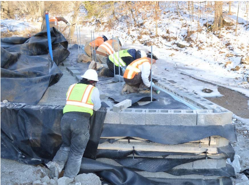
Figure 27. Preparation of second layer of beam seat for north abutment
