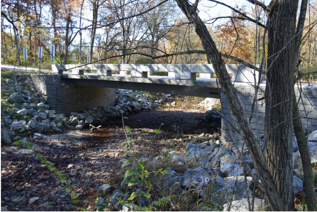
Figure 34. Rustic Road GRS-IBS from the northeast
