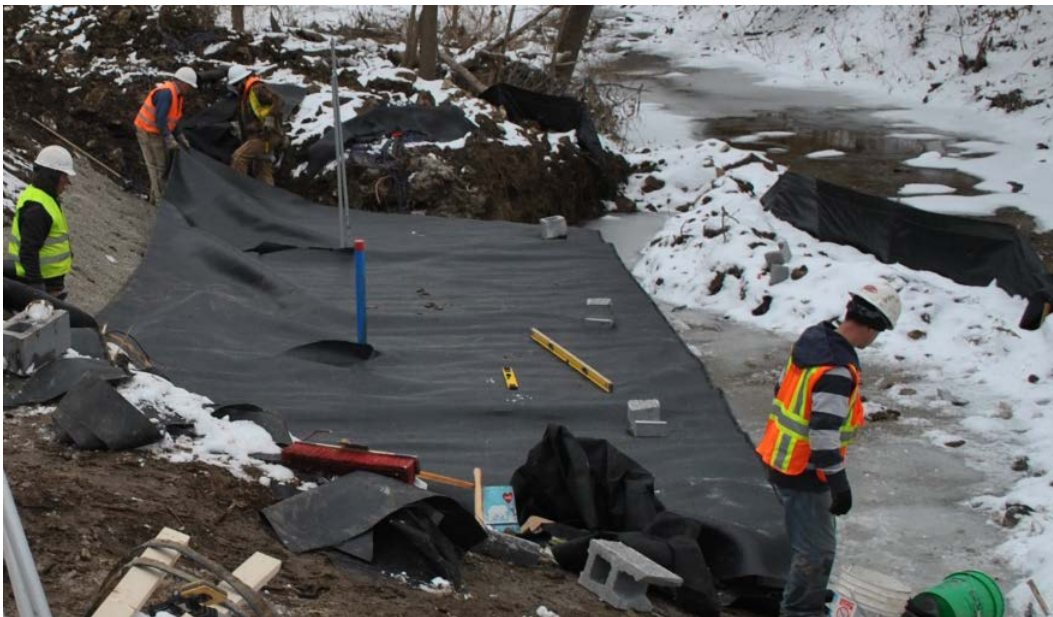
Figure 19. Completed tenth course of GRS of north abutment
