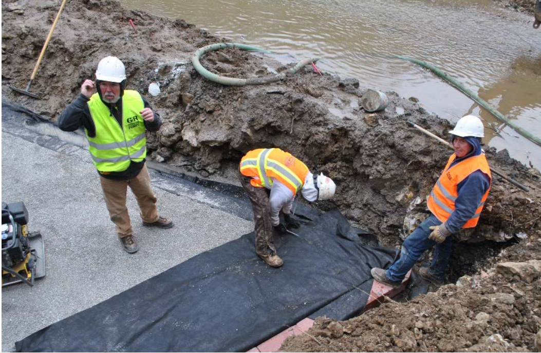
Figure 12. Wrapping separation geotextile around second GRS course of south abutment
