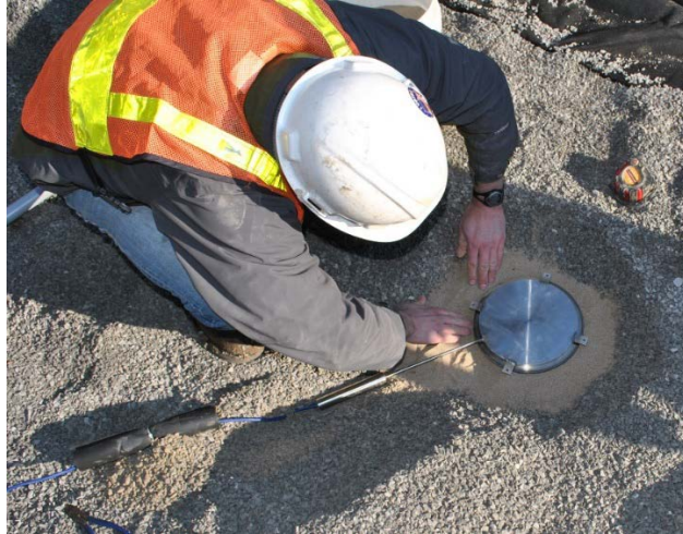
Figure 38. Installation of EPC-1 near bottom of north abutment
