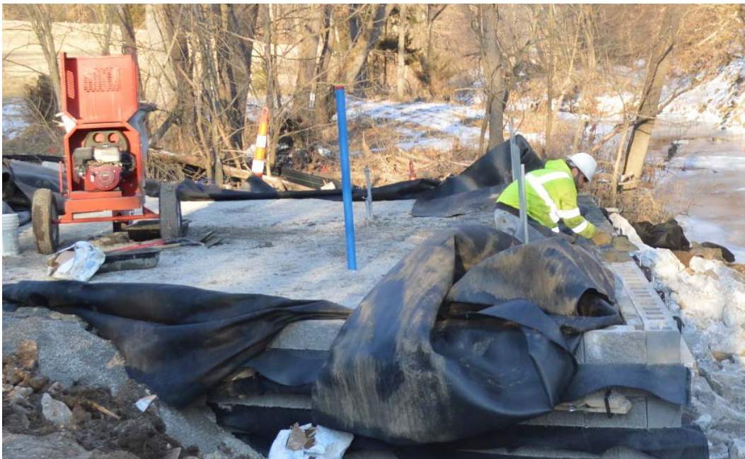
Figure 29. Grouting CMU block openings of top layer of abutment
