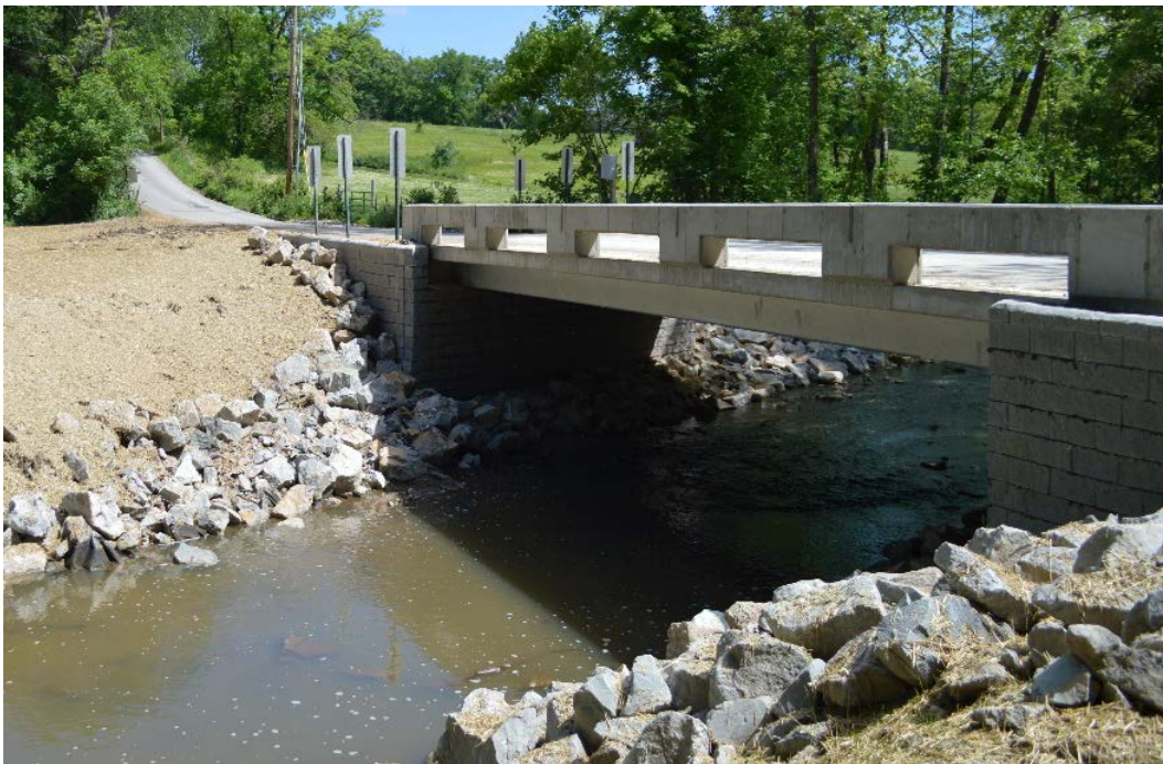
Figure 33. Rustic Road GRS-IBS from the southwest
