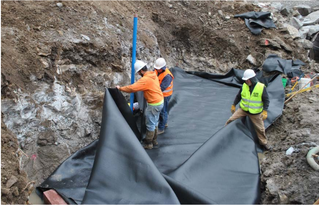
Figure 13. Placement of reinforcement between second and third courses of south abutment
