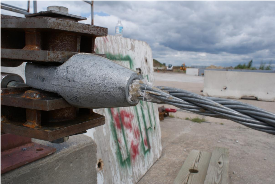
Figure 119. Impact Head Damage and Wire Rope Pull-Through, Test No. DBC-1
