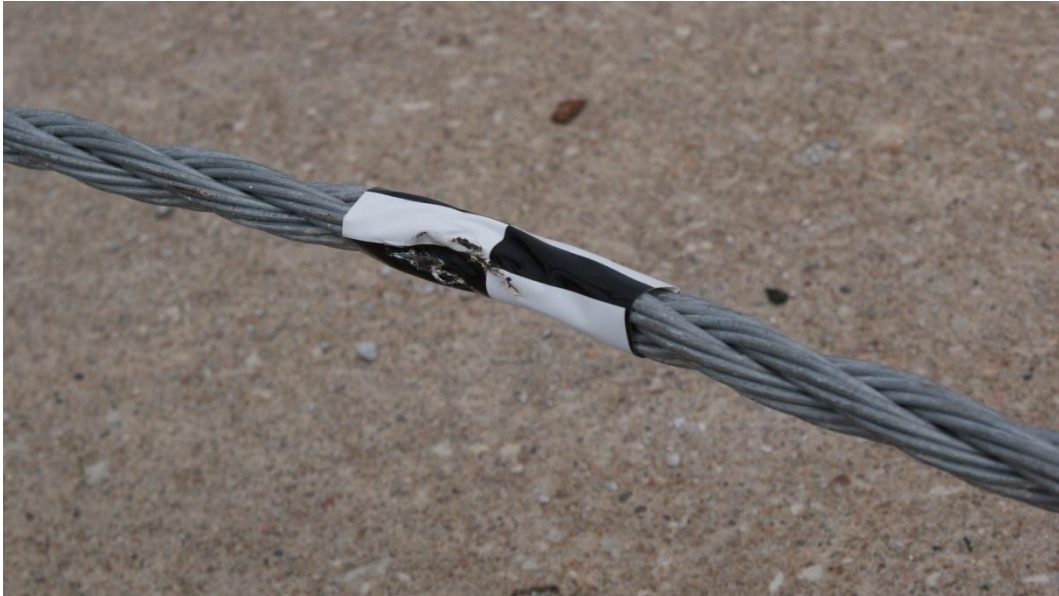
Figure 117. Wire Rope Damage, Test No. DBC-1
