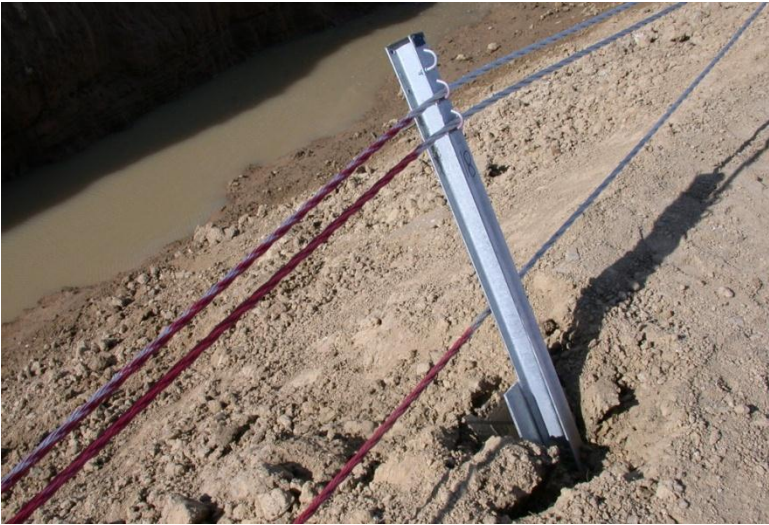
Figure 206. System Damage, Test No. CS-1
