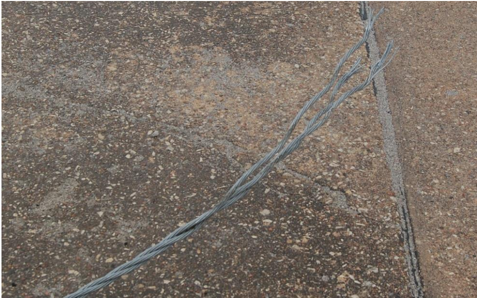
Figure 146. Wire Rope Damage, Test No. DBC-6
