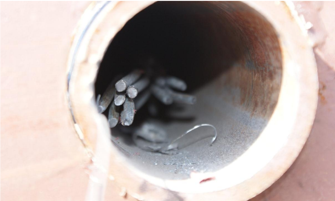
Figure 57. Upstream Wire Rope Damage, Test No. DTC-1
