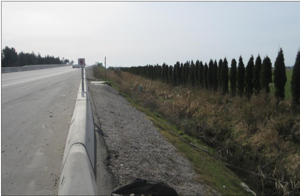
Figure 37. Photo of Vegetation (Cedars) Designed to Reduce Barn Owl-Vehicle Collisions along SFPR in British Columbia
