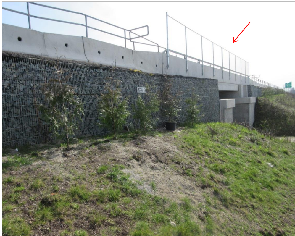
Figure 38. Photo of Chain-Link Fencing (indicated with arrow) to Prevent Low Flight by Barn Owls near an Overpass along SFPR
