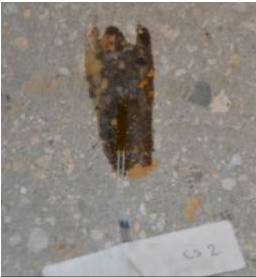
Figure 5.17 Strain Gage Attached to Top of Slab
