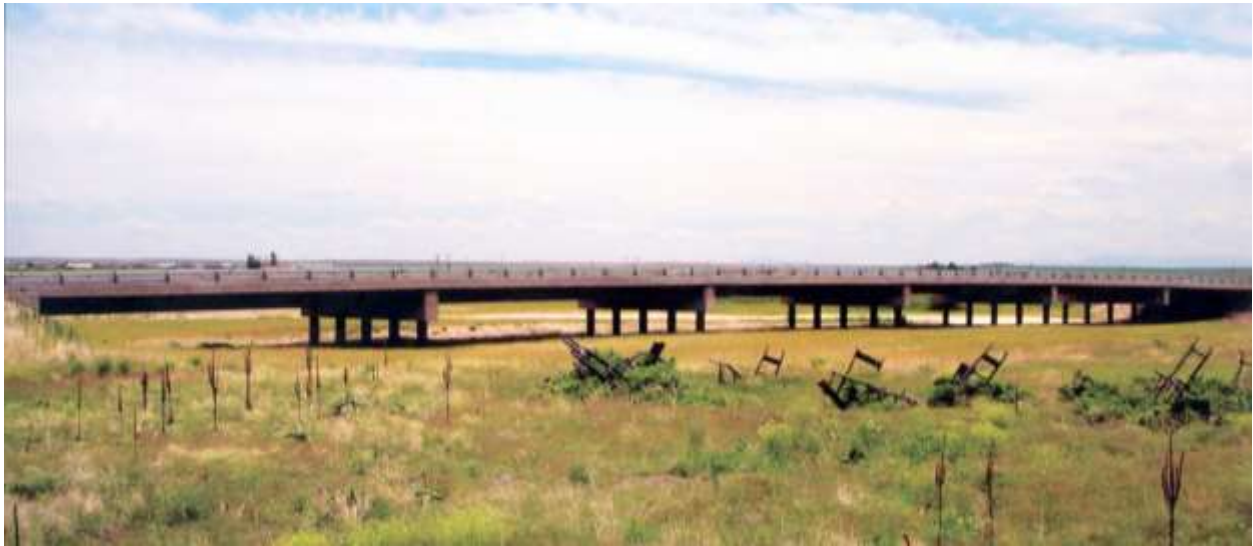
Figure 3.1 SH 36 Over Box Elder Creek (reprinted courtesy of AISC)
