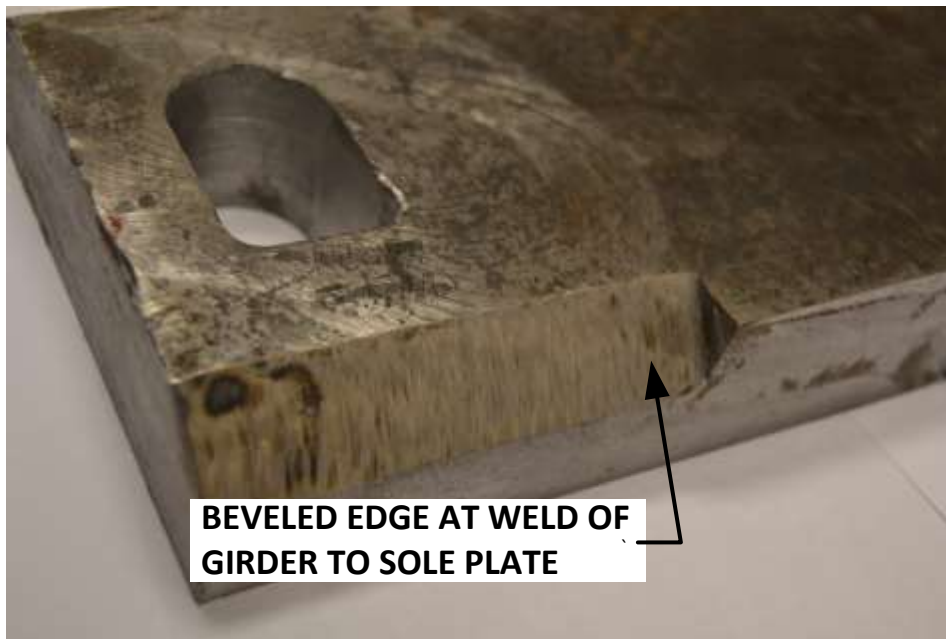
Figure 5.43 Detail of Sole Plate Showing Bevel at Weld
