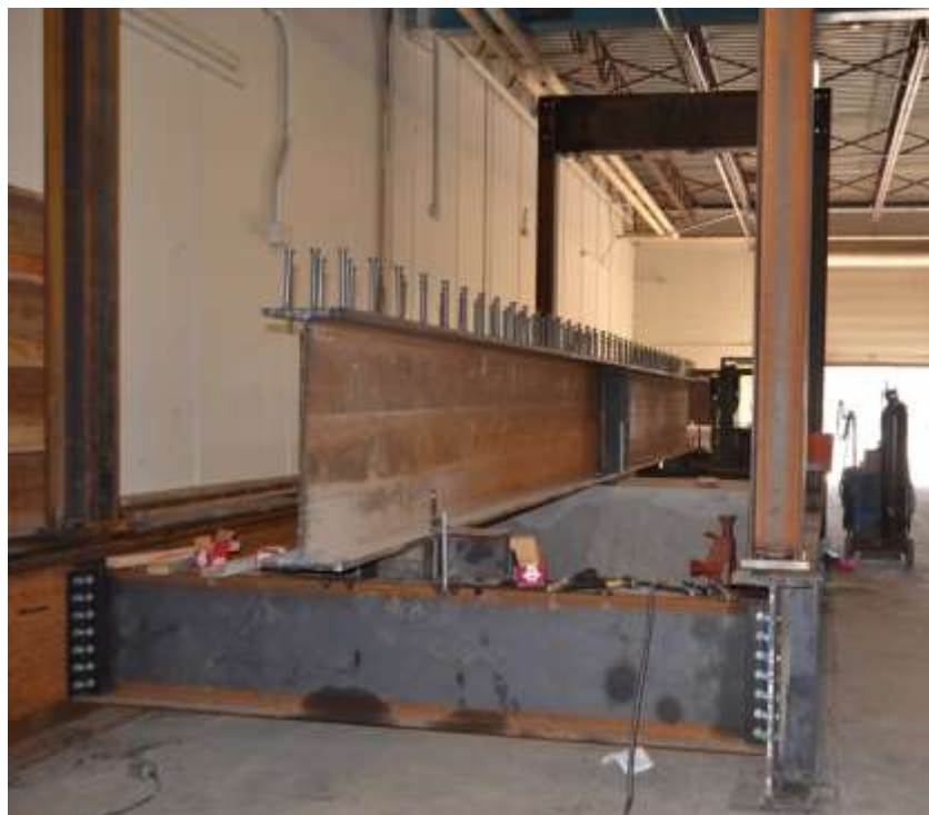
Figure 5.4 Bridge Girders with Studs
