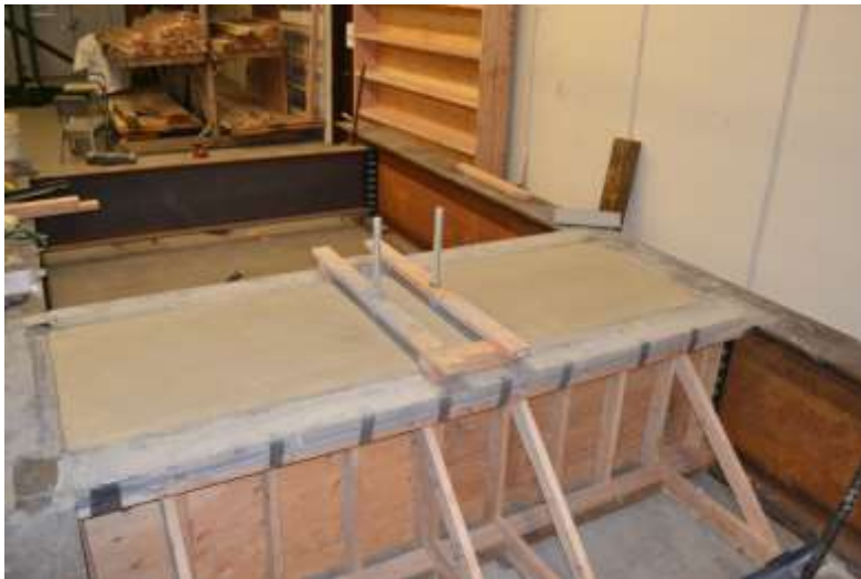
Figure 5.2 Self-Reacting Load Frame - Finished Concrete Support Pier
