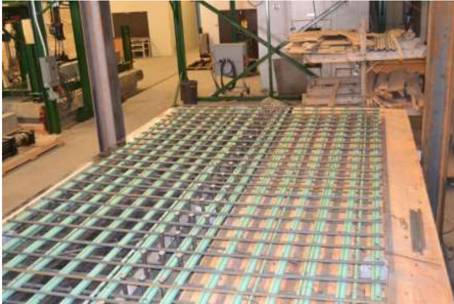
Figure 5.7 Slab Reinforcing Placement
