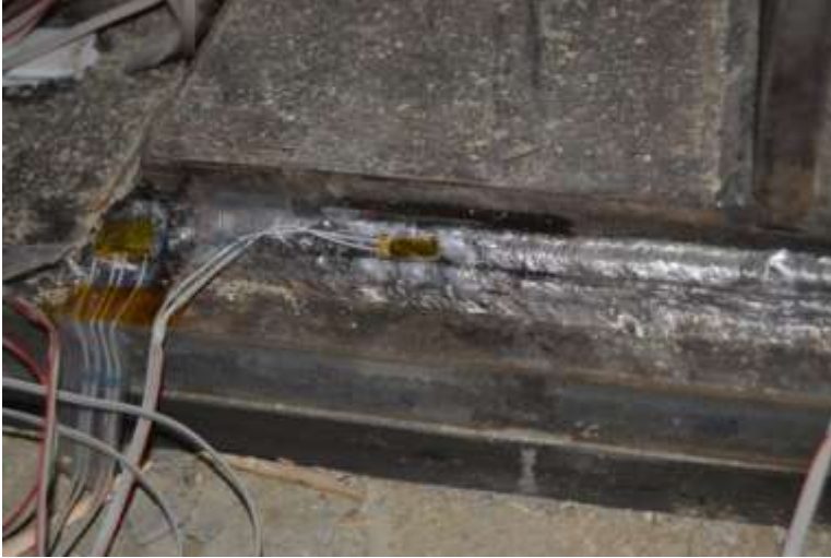
Figure 5.16 Gage Placement at 5/8" Sole Plate Fillet Weld
