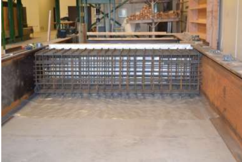
Figure 5.1 Self-Reacting Load Frame - Concrete Support Pier Reinforcing
