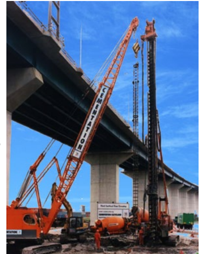
ACIP piles at a bridge interchange.
