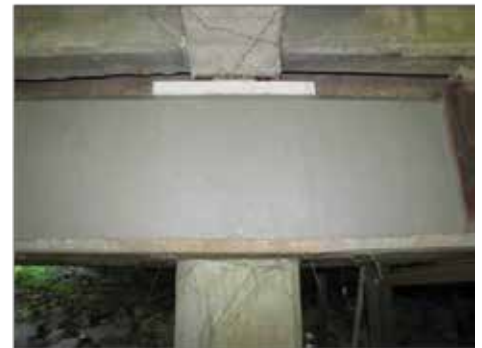
Pile cap repaired with high-strength composites.
