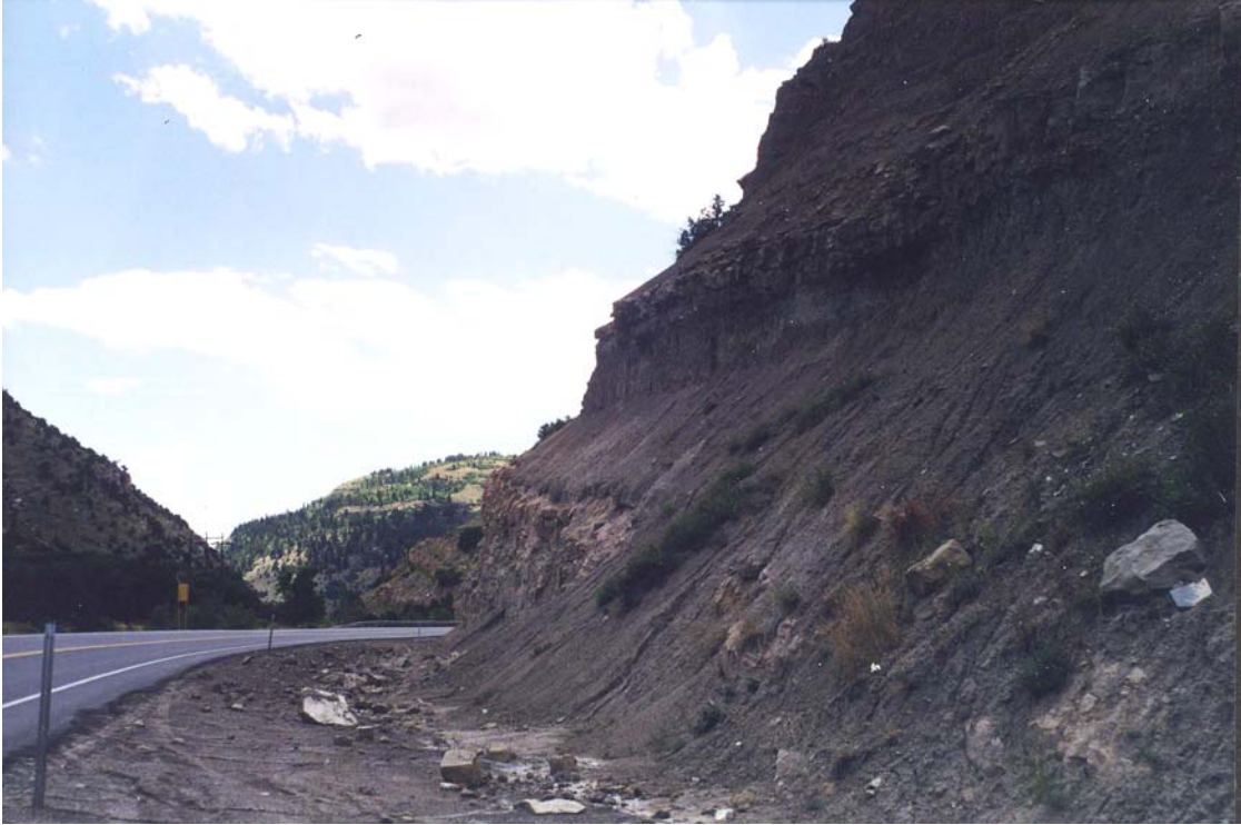
Figure 5. B-rated slope near Colton, Utah.
