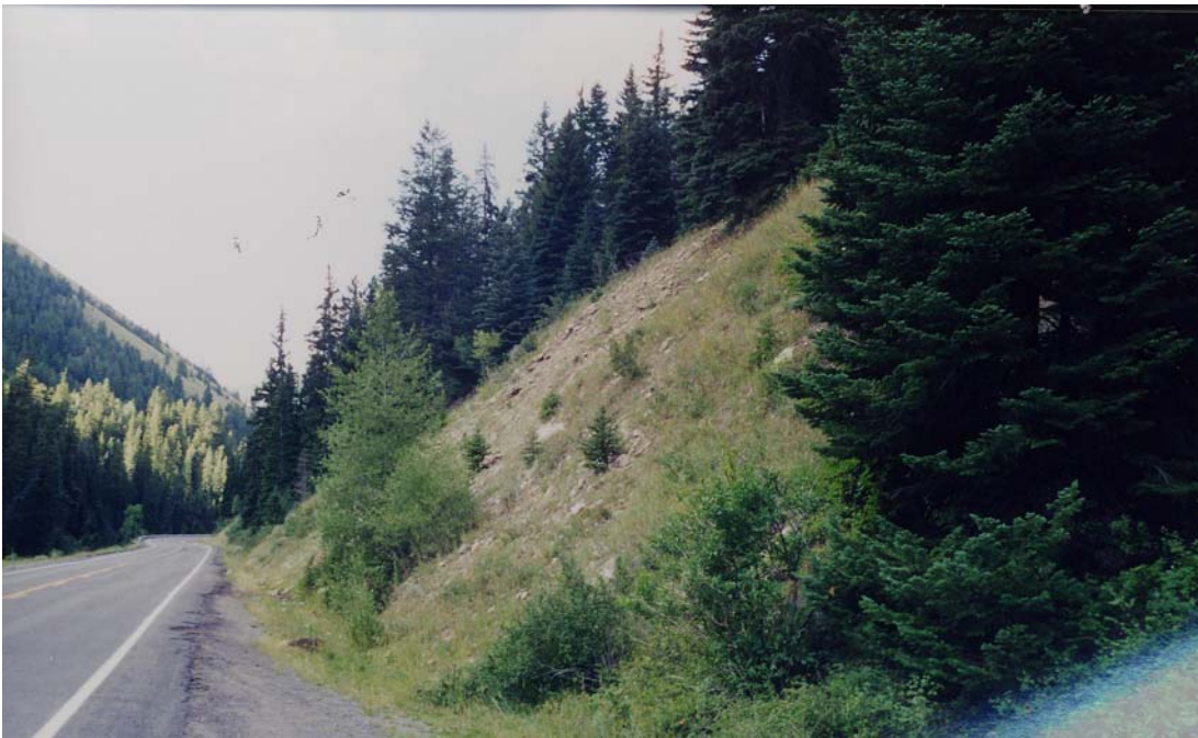
Figure 4. B-rated slope near Huntington, Utah.
