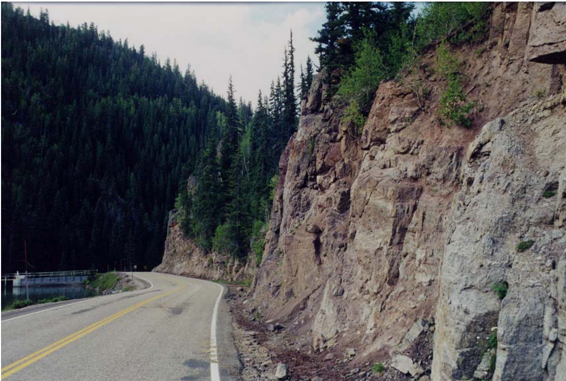
Figure 6. Near-vertical A-rated rock cut in the Beaver Maintenance Station.
