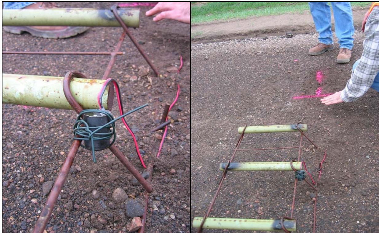
FIGURE C6 Pictures of sensor installation on Unweave the Weave project.
