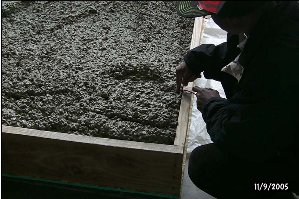
FIGURE B9 Placement of edge maturity meter in MnROAD trial slab.
