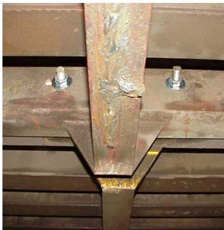
c. Threaded rod on both sides of the transverse member
