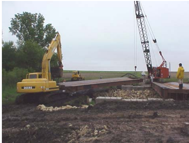
b. Flatcar placement on the cap beams
