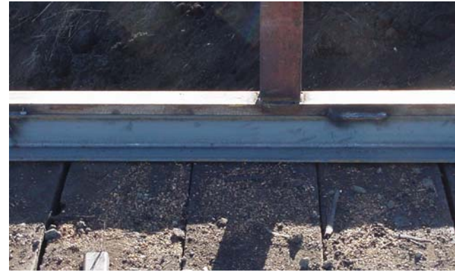
f. Angles welded on the exterior girders
