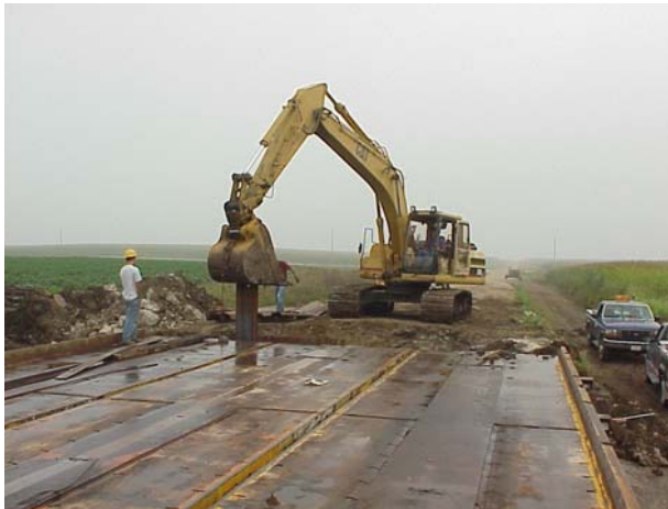
g. Driving sheet piling with a backhoe
