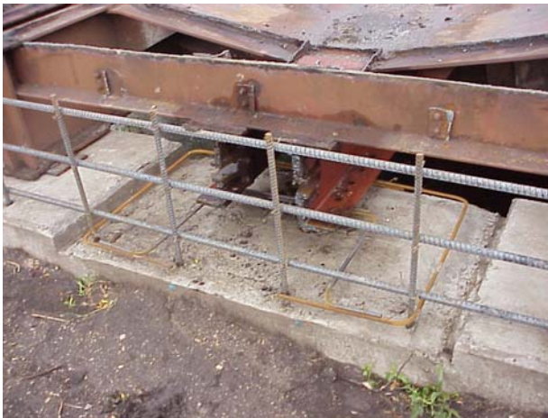
c. Backwall and interior girder seat reinforcement
