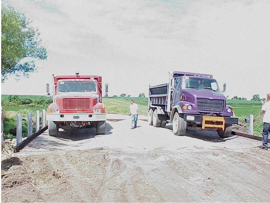
a. Testing prior to placement of the driving surface
