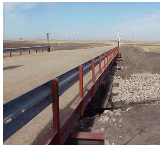
b. Installation of the thrie beam
