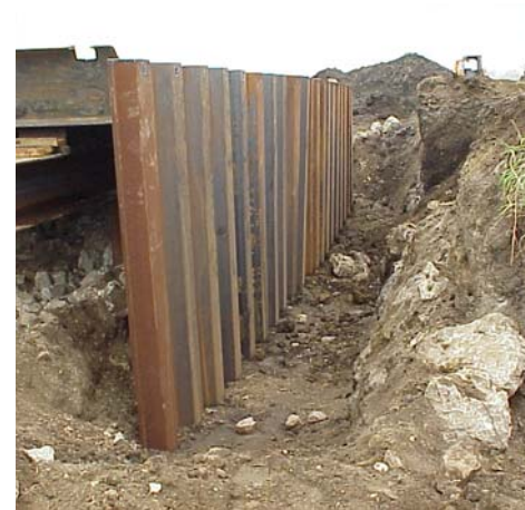
h. Completed sheeting wall
