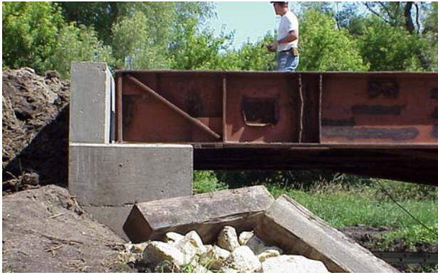
d. Completed abutment backwall
