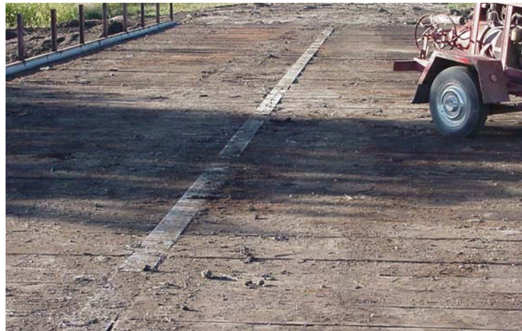
g. Placement of the recycled, transverse timber planks
