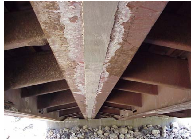
d. Connection after concrete placement
