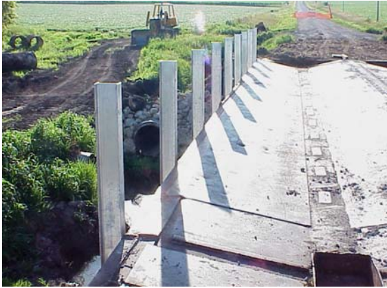
a. Guardrail posts welded on the BCB
