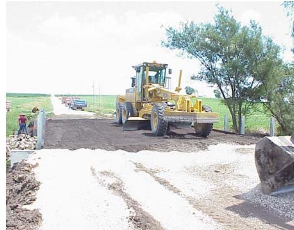
d. Blading the asphalt milling driving surface
