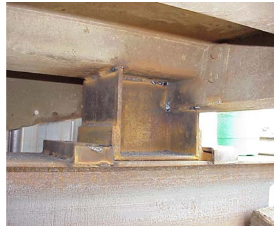
d. Exterior girder support in place at the north abutment
