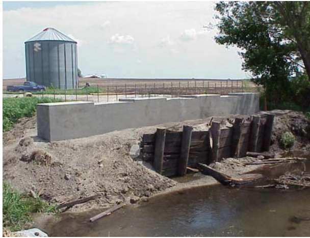
a. Concrete cap beam prior to RRFC placement
