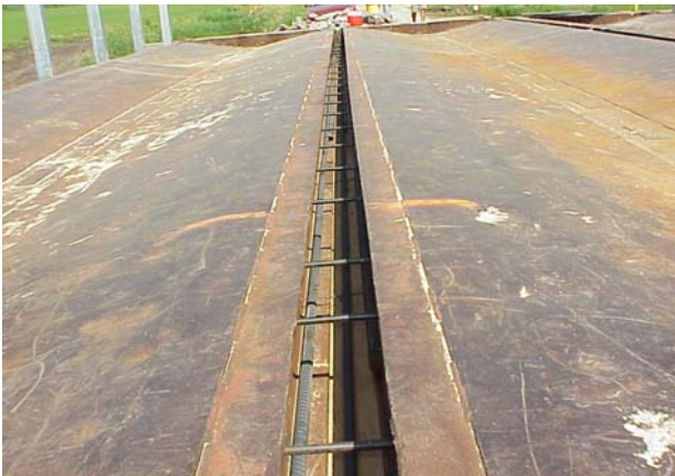
c. Threaded rod and longitudinal reinforcement
