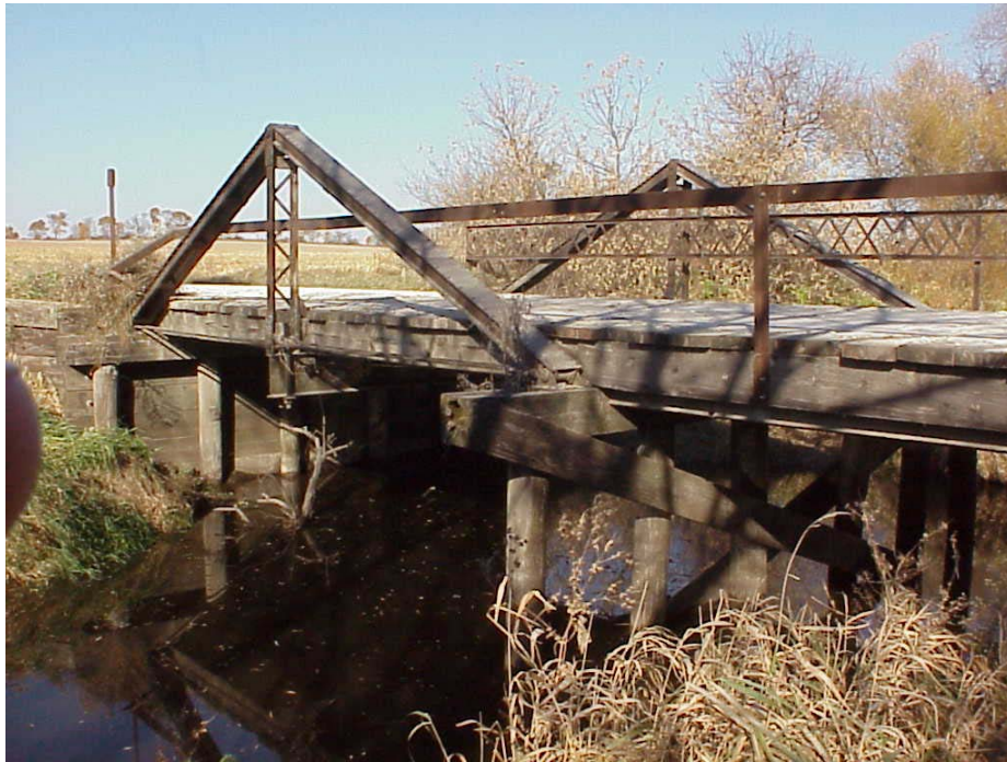
b. Photograph of the original bridge
