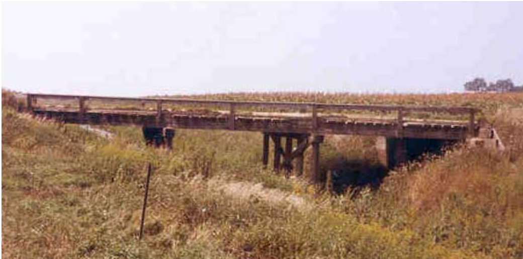
b. Photograph of the original bridge
