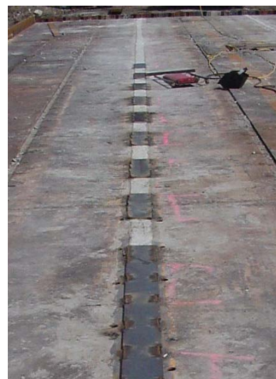
d. Top connection plates after concrete placement
