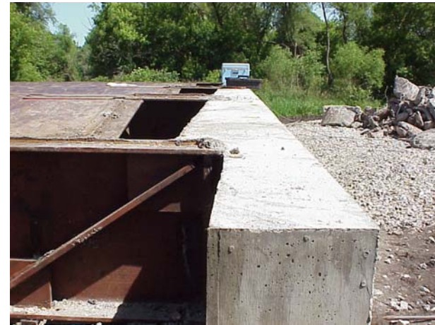
g. Integral east abutment
