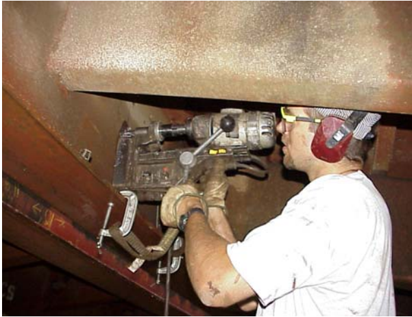
a. Drilling holes for the transverse threaded rod
