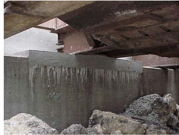
e. Completed interior girder seat
