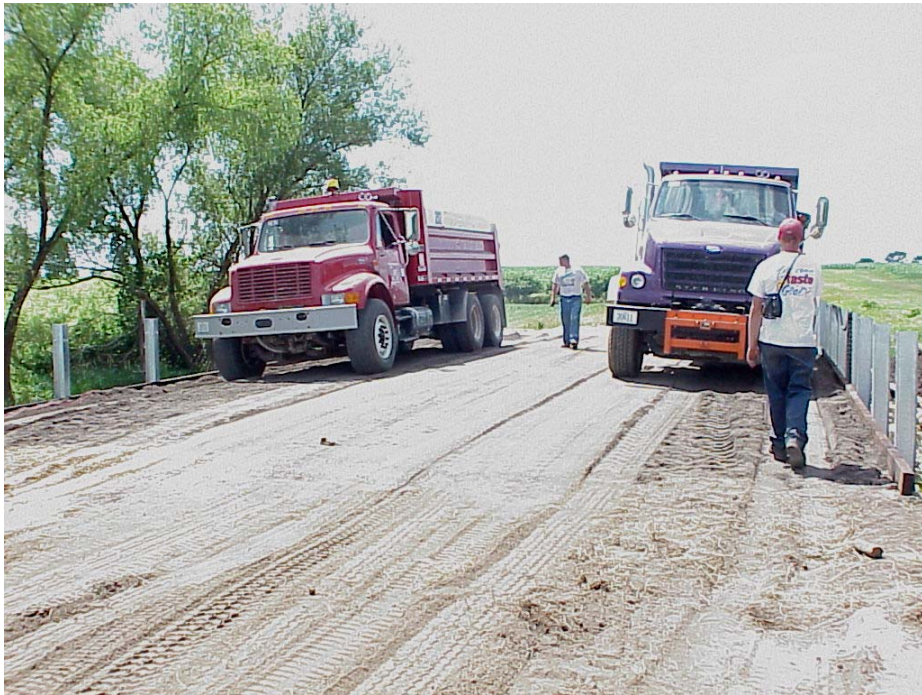
b. Testing after placement of the driving surface
