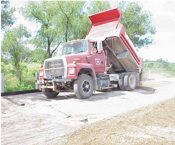
c. Laying pea gravel
