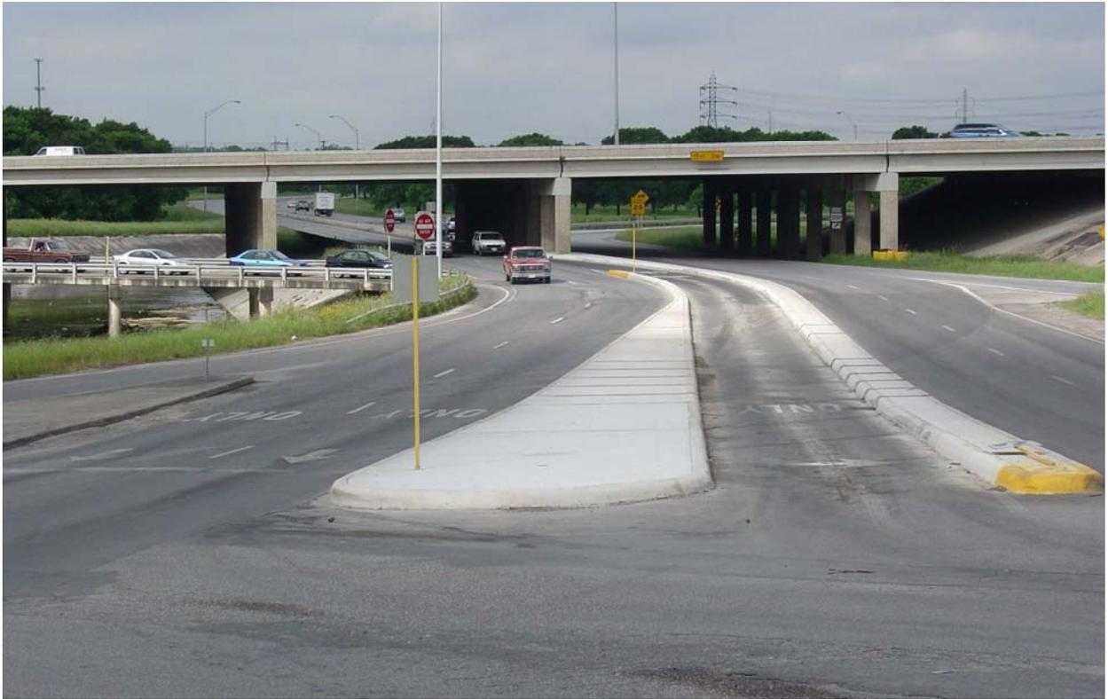
Figure 11-8. Median Added to Limit Left Turns by Traffic from Ramp.
