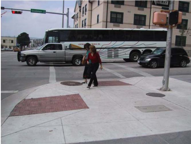
Figure 7-3. Photo of Perpendicular Curb Ramps.
