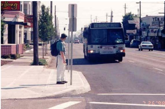
Figure 5-23. Example of Bus Bulb.
