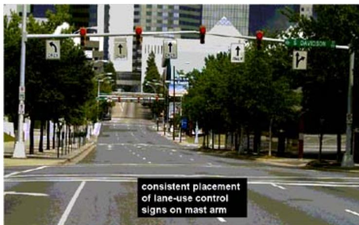
Figure 10-18. Placement of Overhead Lane-Use Control Signs.<sup>8</sup>
