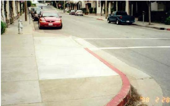
*Figure 5-21. Example of a Curb Extension.*
