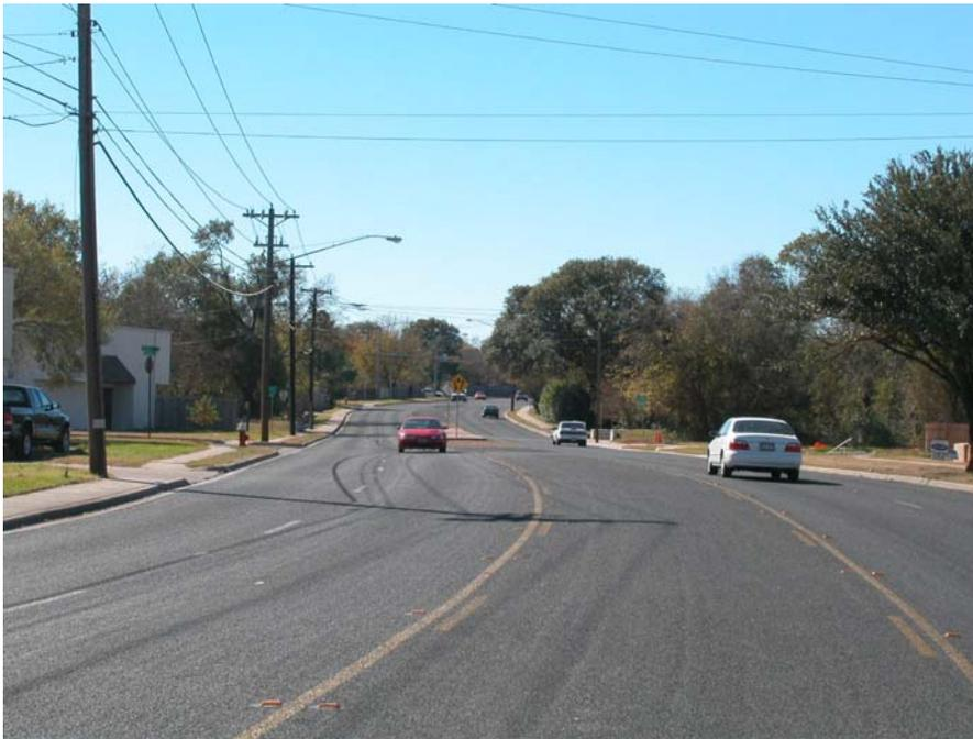
Figure 9-1. Example of Longitudinal Pavement Markings.
