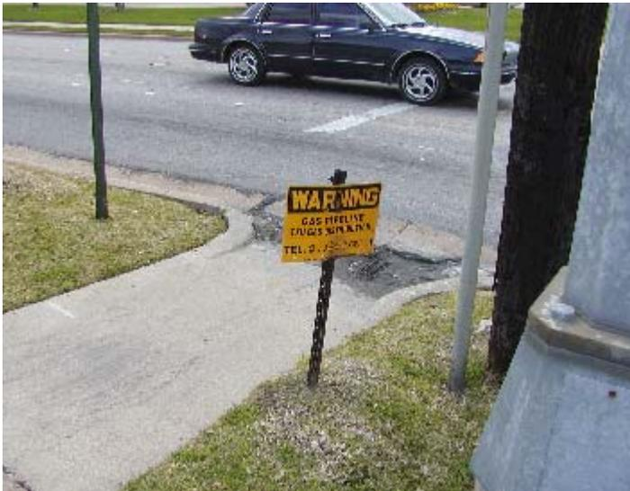
*Figure 5-32. Example of Utility Marker at Intersection.*
