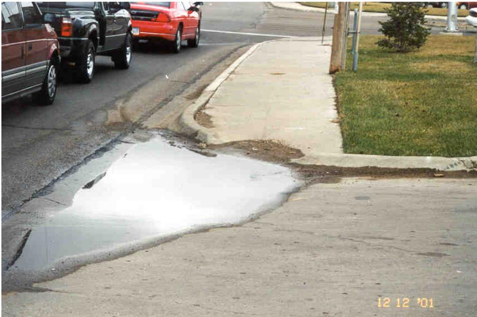
Figure 6-17. Ponding at Curb Ramp (Older, Non-Compliant Curb Ramp).
