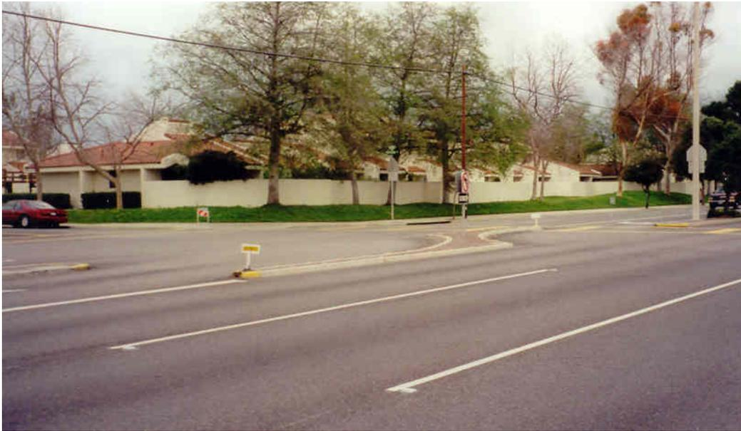
Figure 11-11. Channelized Median Opening to Restrict through Movements.
