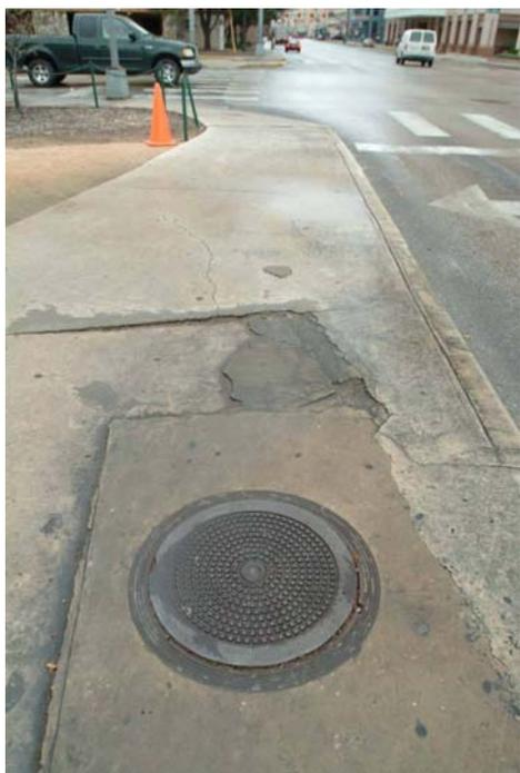
Figure 7-14. Utility Cover in the Pedestrian Path at Southeast Corner.
