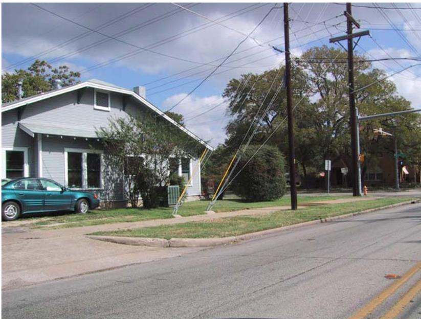
*Figure 5-29. Guy Wire Parallel to Sidewalk.*
