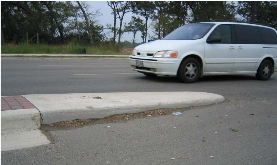
Figure 4-22. Ramped Down Median Nose.
