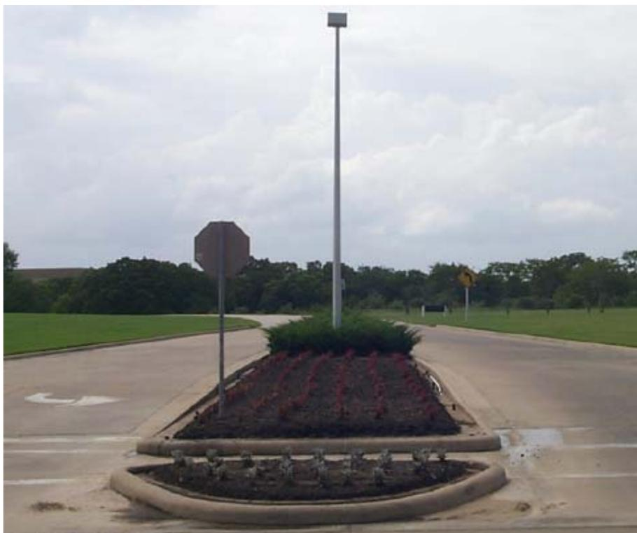
Figure 4-20. Example of Median Nose.
