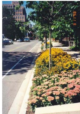
*Figure 5-12. Example of Continuous Landscaping to Encourage Lower Operating Speeds.*
