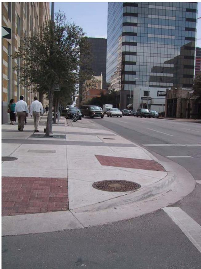
Figure 5-31. Example of Manhole Outside Pedestrian Access Route.
