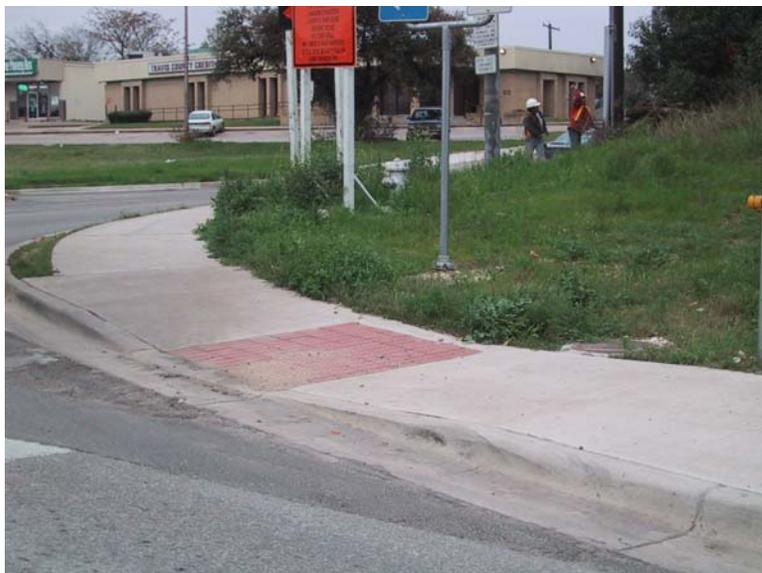
Figure 7-5. Photo of Parallel Curb Ramp.
