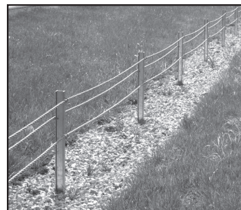
Left: A standard three-strand cable median barrier is shown. Below: A high-tension four-strand cable median barrier is shown.
