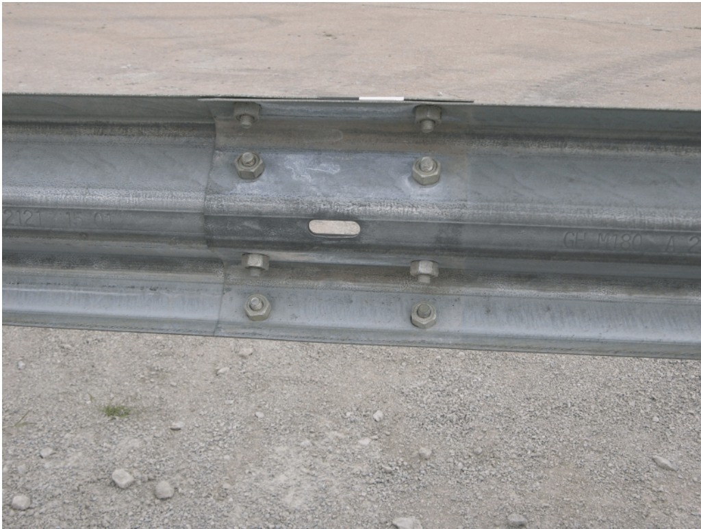
Figure 53. Splice Details, Design No. 2
