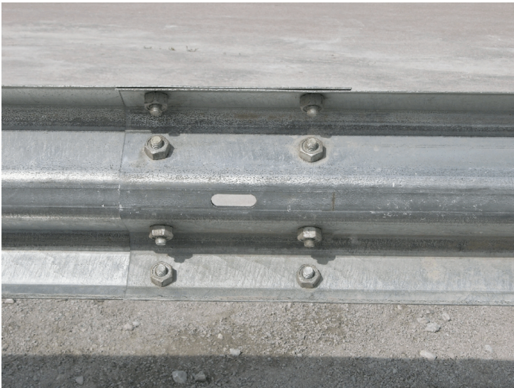
Figure 30. Splice Details, Design No. 1
