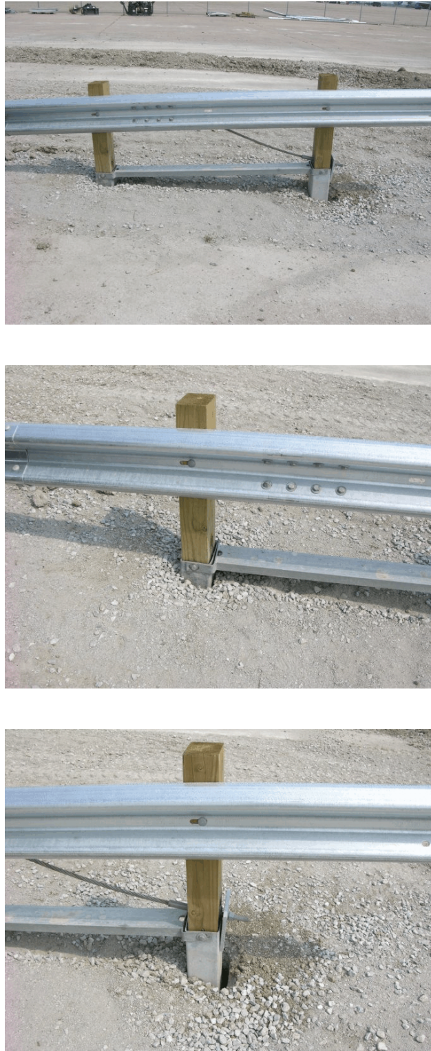
Figure 41. Downstream Anchorage Damage, Test No. MGS221-1
