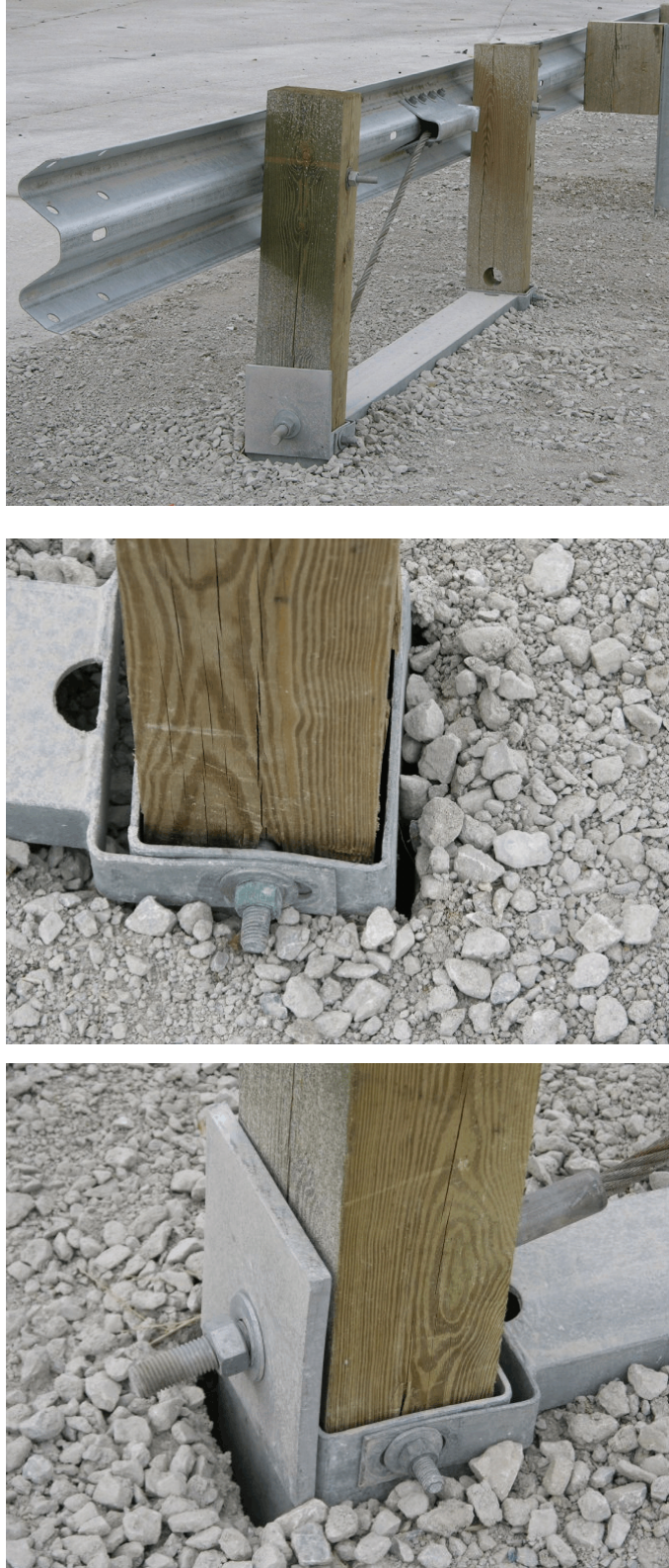
Figure 64. Downstream Anchorage Damage, Test No. MGS221-2
