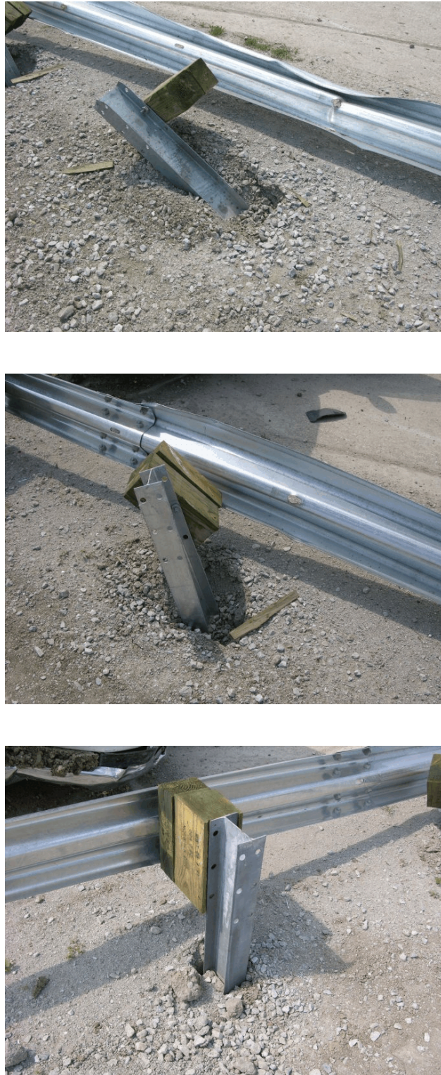
Figure 39. Post Nos. 25 through 27 Damage, Test No. MGS221-1
