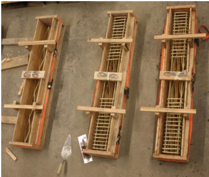
Figure 3.39 Specimen forms assembled with reinforcement in place for pour B
