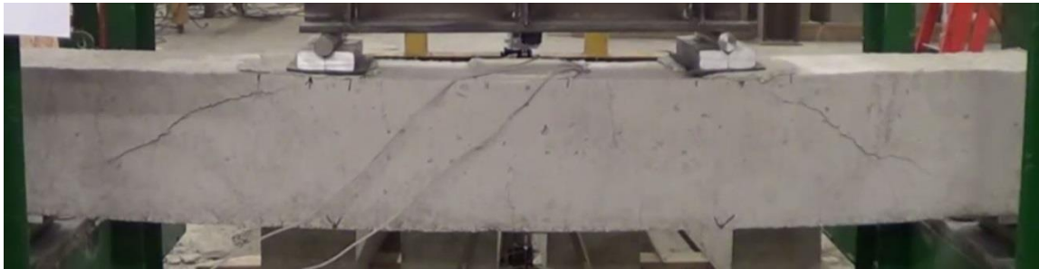
Figure 4.18 IIb-1 shear cracking before collapse event
