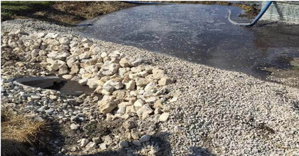
Figure 4.17 Flooding observed during testing at around 5 minutes.
