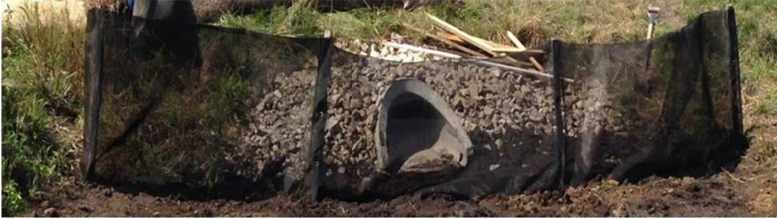
Figure 4.3 Silt fence (woven monofilament).
