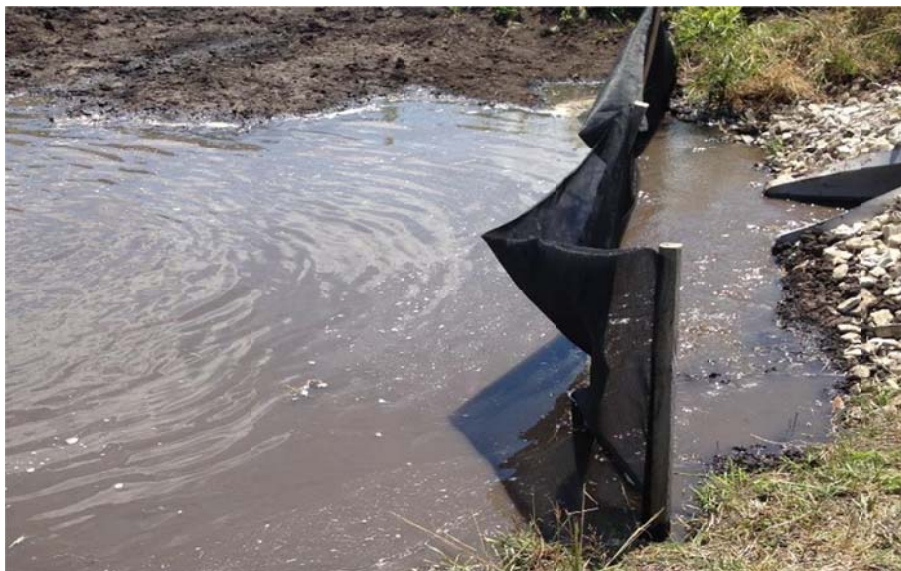
Figure 4.5 Flow through the silt fence (woven monofilament) during the test.
