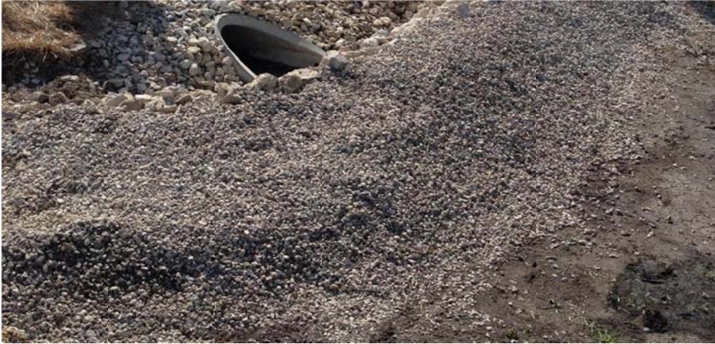
Figure 3.5 Flared-end inlet protection using stone.
