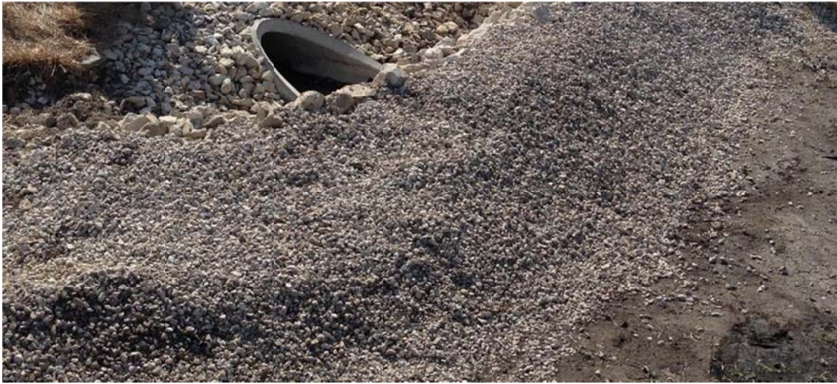
Figure 4.16 Stone check dam.
