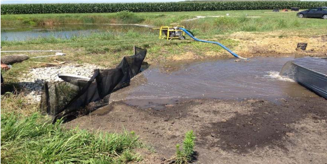
Figure 4.4 Silt fence (woven monofilament) at 158 gpm (10 L/s) flow rate.
