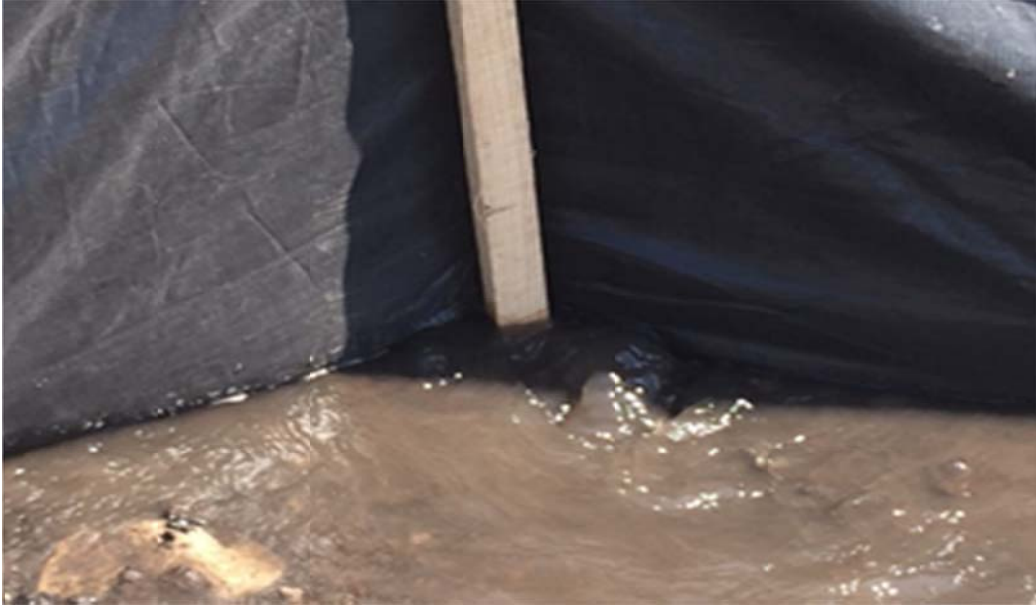
Figure 4.10 Product undercutting (silt fence with IDOT-approved fabric).
