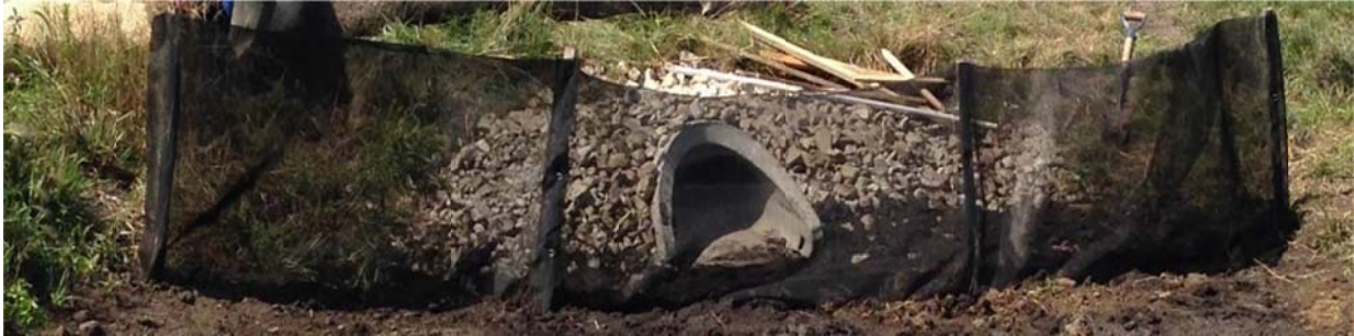
Figure 3.2 Silt fence with woven monofilament.
