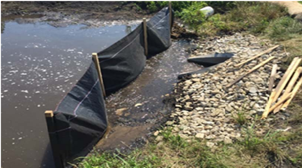
Figure 4.9 Water pressure stressing the silt fence with IDOT-approved fabric.
