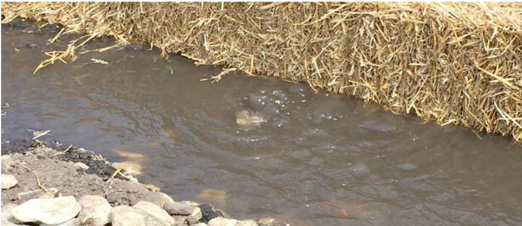
Figure 4.12 Product undercutting.
