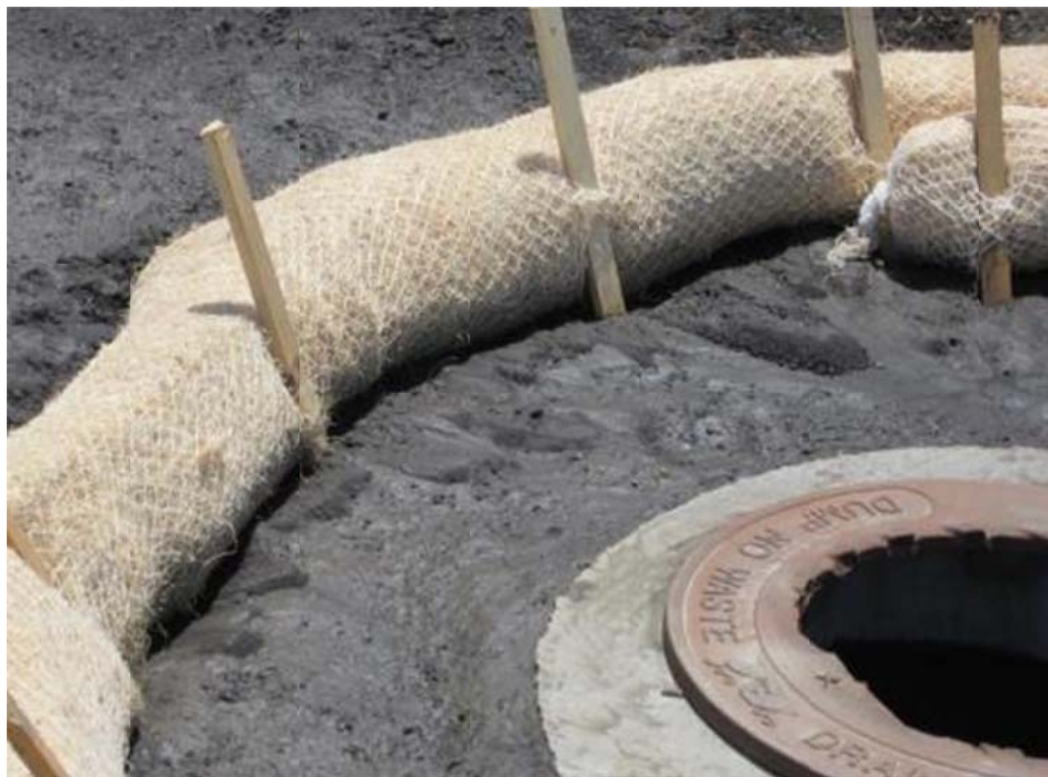
Figure A.6 Sediment log installation.
