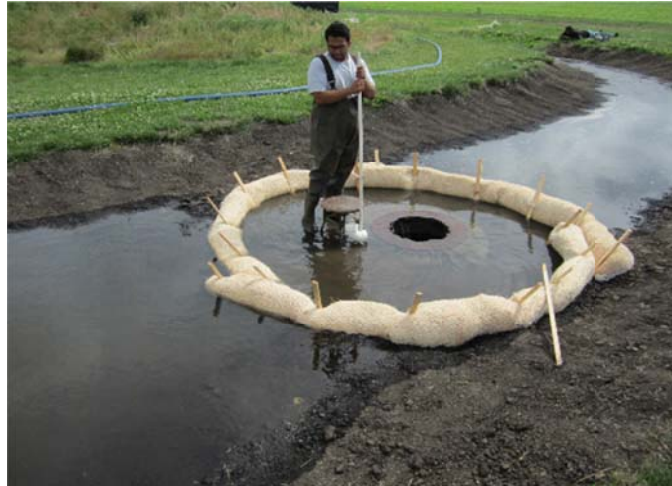
Figure 4.5 Sediment log without erosion control blanket, under 79 gpm (5 L/s) flow rate.
