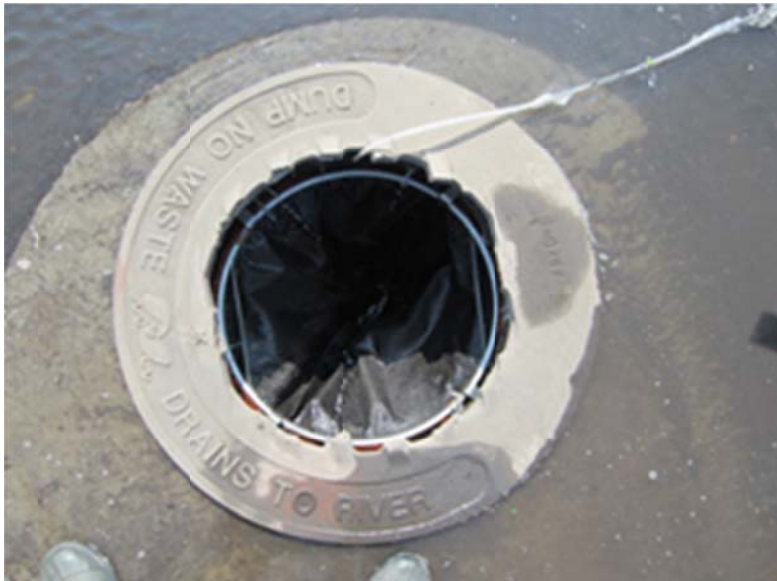
Figure 4.13 Filter bag at 79 gpm (5 L/s) flow rate, inside.
