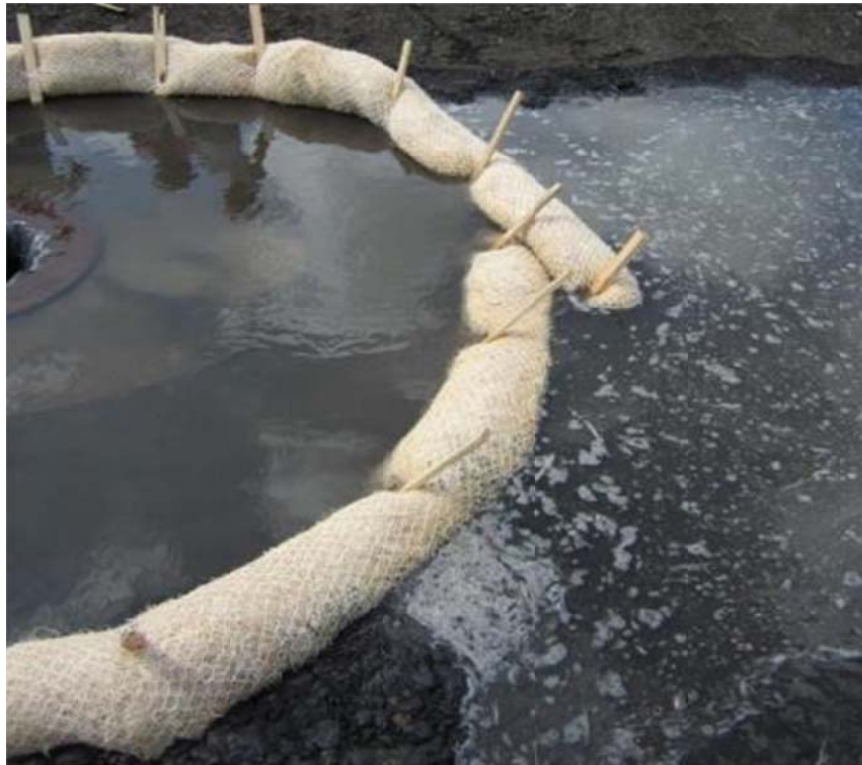
Figure A.8 Sediment log water accumulation.
