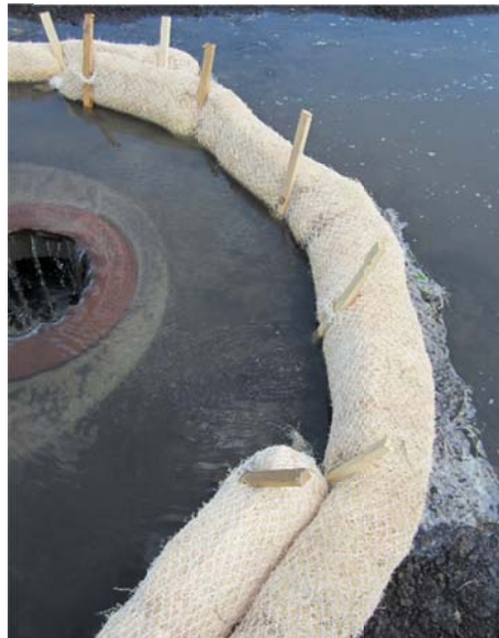
Figure 4.6 sediment settling on the concrete pad of the inlet.
