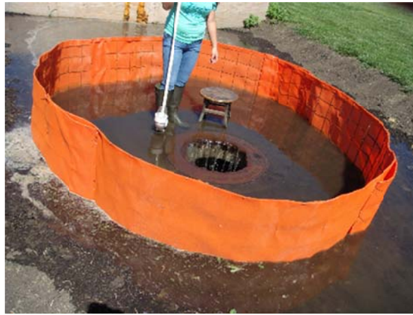
Figure 4.3 Welded-wire woven monofilament with 2 foot gap under 79 gpm (5 L/s) flow rate.
