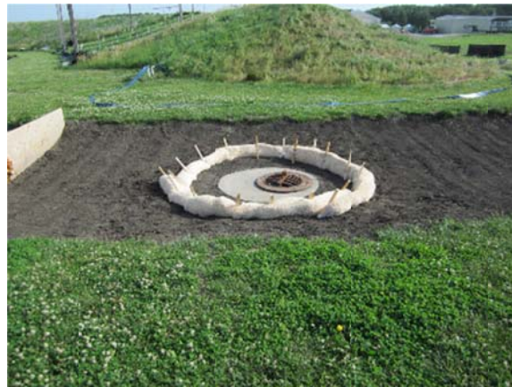
Figure 3.3 Sediment log with no erosion control blanket.
