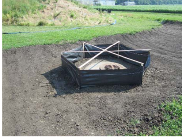
Figure 3.8 Silt fence with 2 foot gap.
