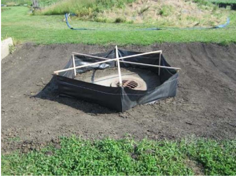
Figure A.17 Silt fence (2 foot gap), pre-testing.
