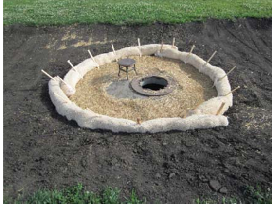
Figure 3.4 Sediment log with erosion control blanket.
