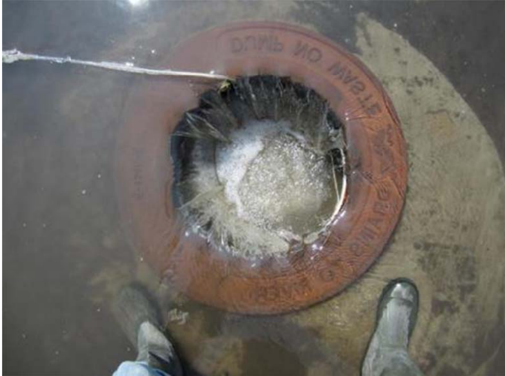
Figure A.15 Drop filter bag, with water overflowing product.
