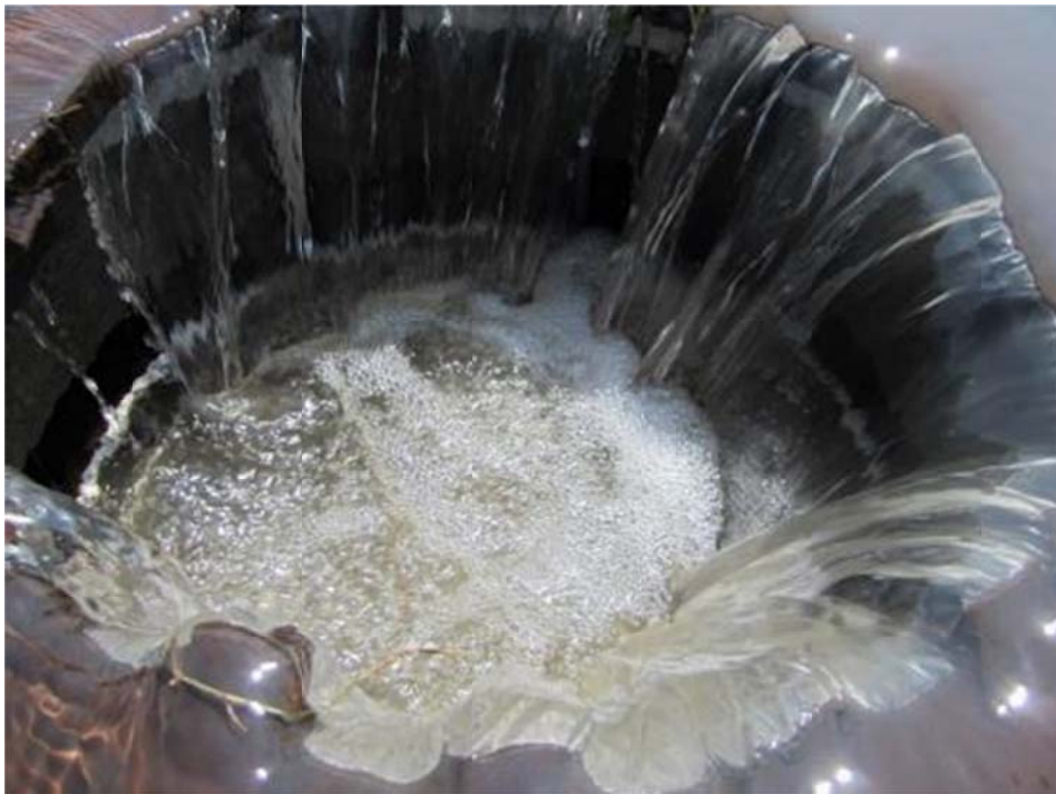
Figure A.16 Drop filter bag overflowing manhole.
