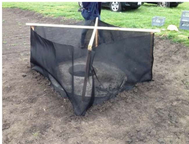
Figure 3.9 Silt fence with woven monofilament fabric.
