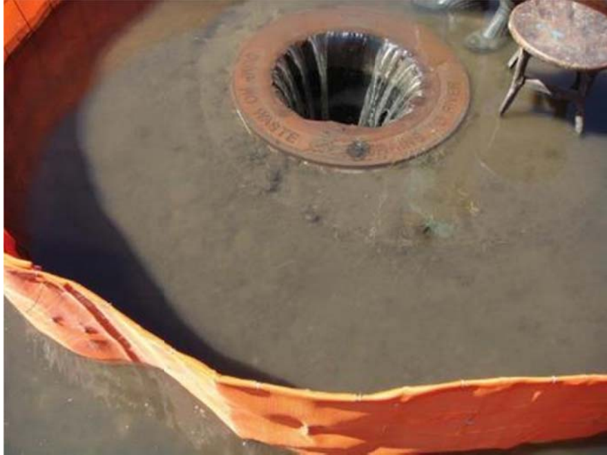
Figure A.3 Welded-wire woven monofilament fabric entering manhole.
