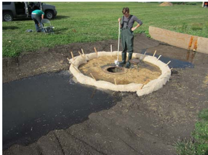
Figure 4.8 Sediment log with erosion control blanket, at 79 gpm (5 L/s) flow rate, with water not flowing around it.
