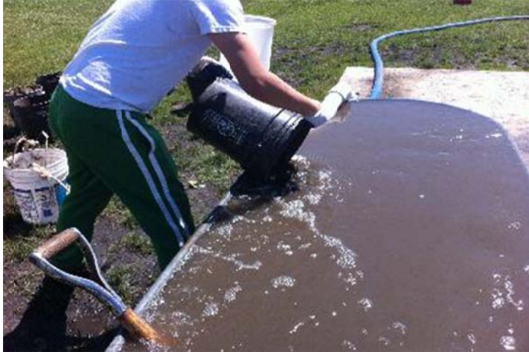
Figure 3.14 Adding clay soil.
