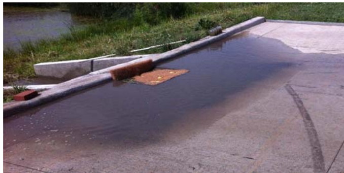
Figure 4.16 Ponding around the SediGuard.
