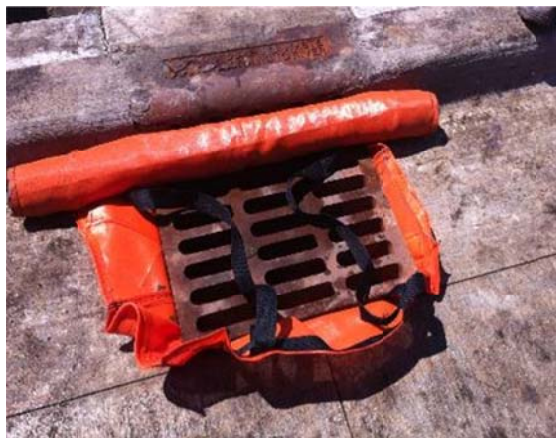
Figure 3.3 Outside view of installed Dandy curb sack product.
