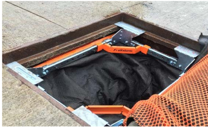
Figure 4.1 Frame installed under a grate.
