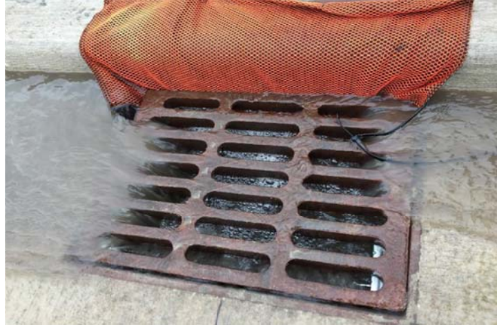
Figure 4.3 Frame and grate overflow protection.
