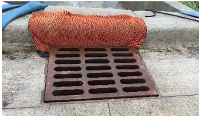
Figure 3.1 Outside view of installed frame and grate product.
