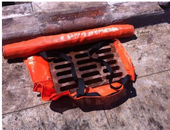
Figure 4.4 Dandy curb sack (installed).
