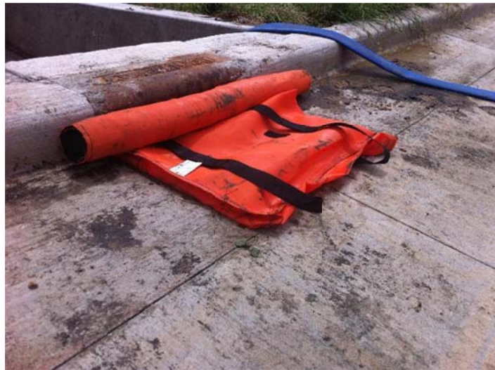
Figure 4.6 Dandy curb bag (installed).
