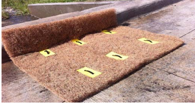
Figure 4.14 SediGuard (installed).
