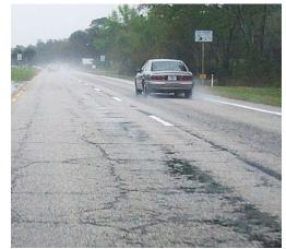
Note the extensive cracking in this roadway, both along and across its length. On the right, cracking has resulted in spalling and a significant loss of pavement integrity.
