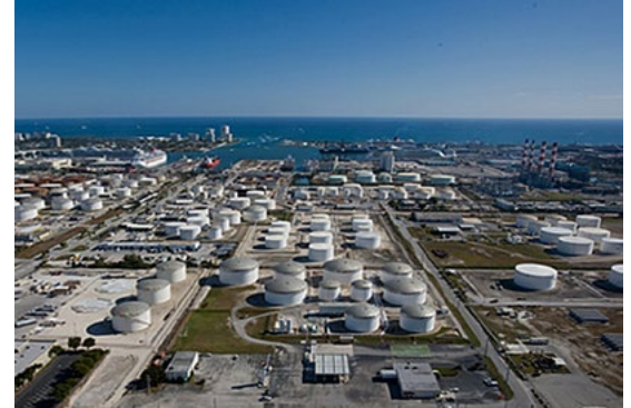
Fuel storage tanks at Port Everglades.
