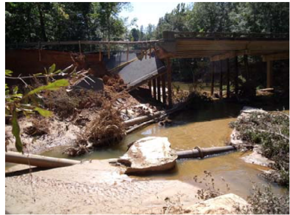
Figure 2.1. Repairable abutment damage in GA flood of 2009. Figure 2.2 Abutment failure in GA flood of 2009.
