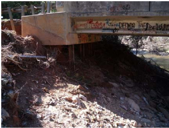
Figure 2.1. Repairable abutment damage in GA flood of 2009. Figure 2.2 Abutment failure in GA flood of 2009.
