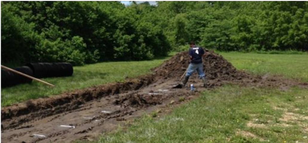
Figure 3.3: Topsoil Source Area
