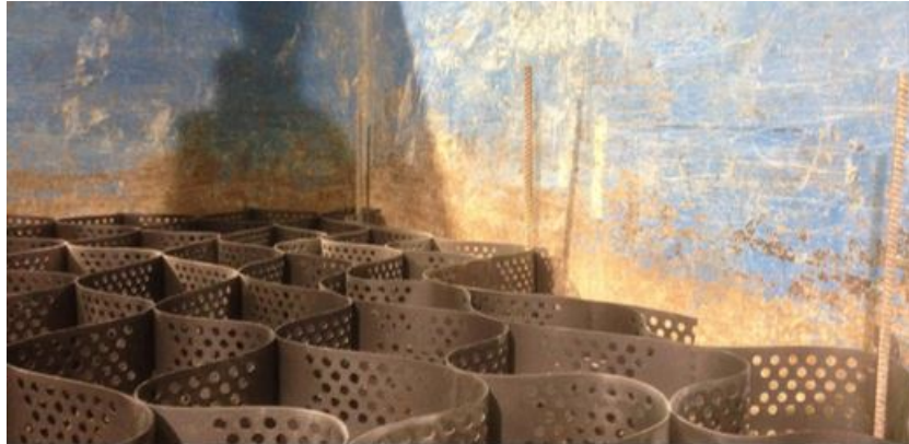
Figure 5.6: Placement of Geocell
