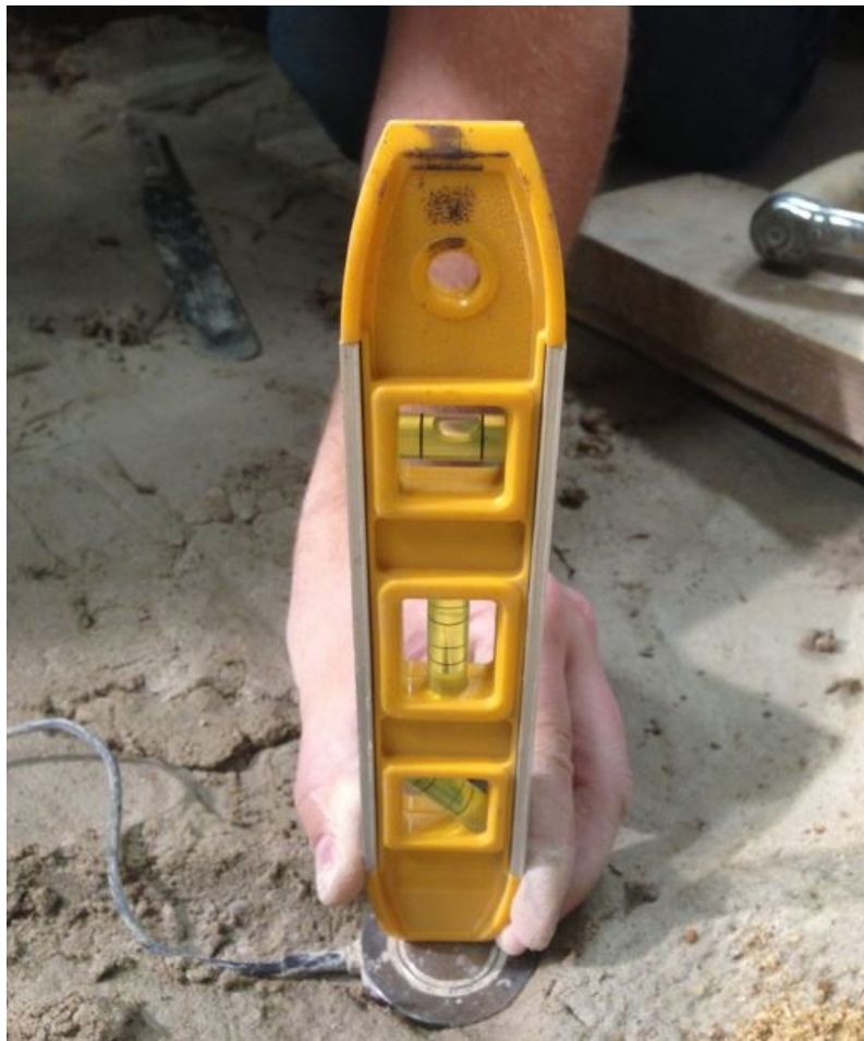
Figure 5.5: Installation of Earth Pressure Cell
