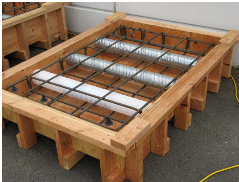
Figure 3 – Typical specimen formwork with post-tensioning ducts and rebar cage
