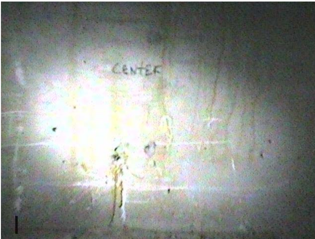
Figure 41 – Photo of Heating Location # 1
