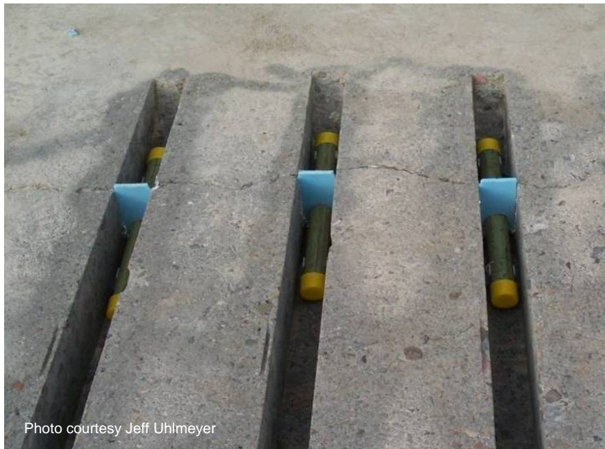
Figure 56 Dowel bar retrofit assembly at a transverse crack.
