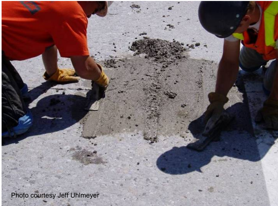
Figure 70 Finishing patching material.
