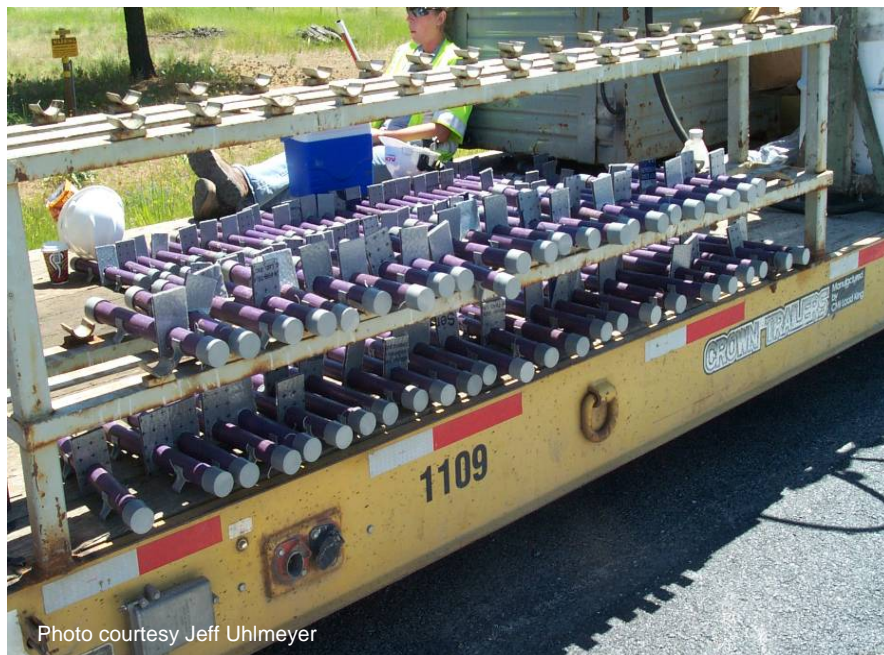
Figure 51 Dowel bar retrofit assemblies.
