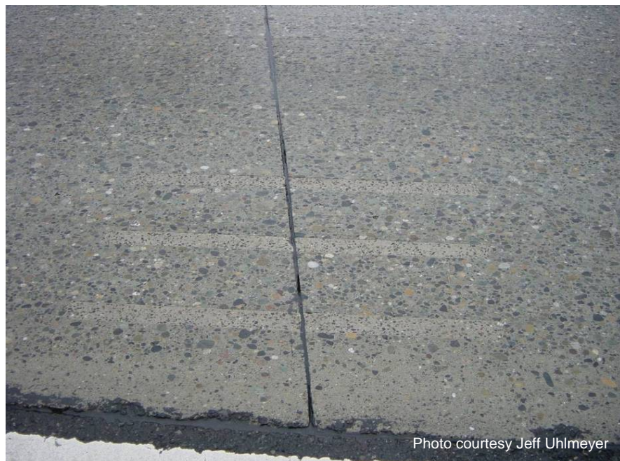
Figure 84 Close-up of completed dowel bar retrofit.
