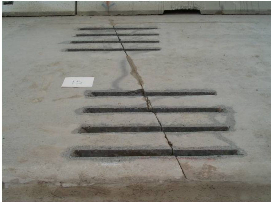
Figure 13 Dowel bar slots on a skewed transverse joint.
