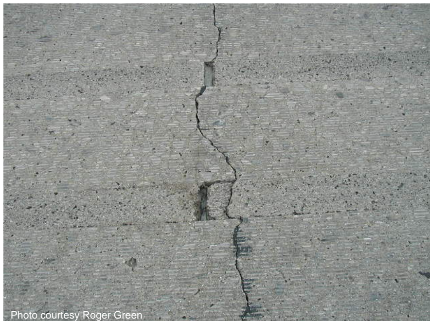
Figure 66 Misaligned foam core board.
