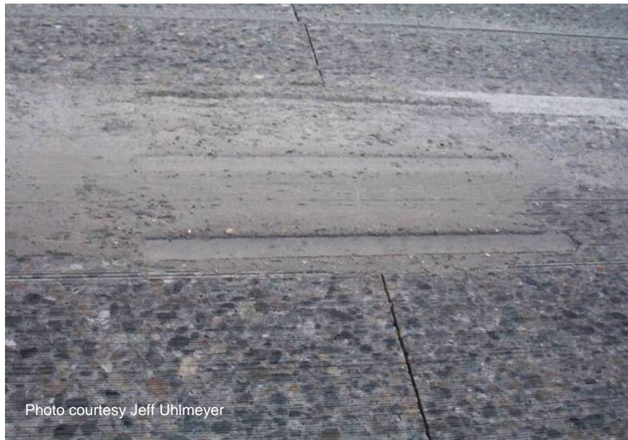
Figure 77 Mechanical sweeping prior to patching material reaching strength.
