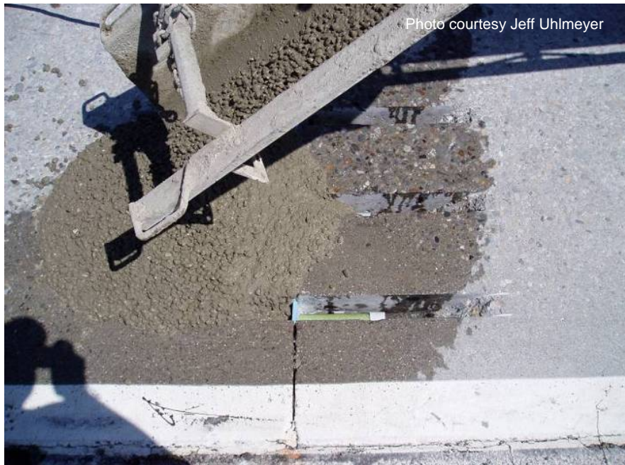
Figure 63 Placing patching material adjacent to dowel bar slots.
