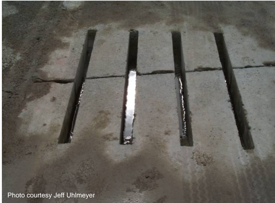
Figure 42 Water must be removed prior to placement of patching material.
