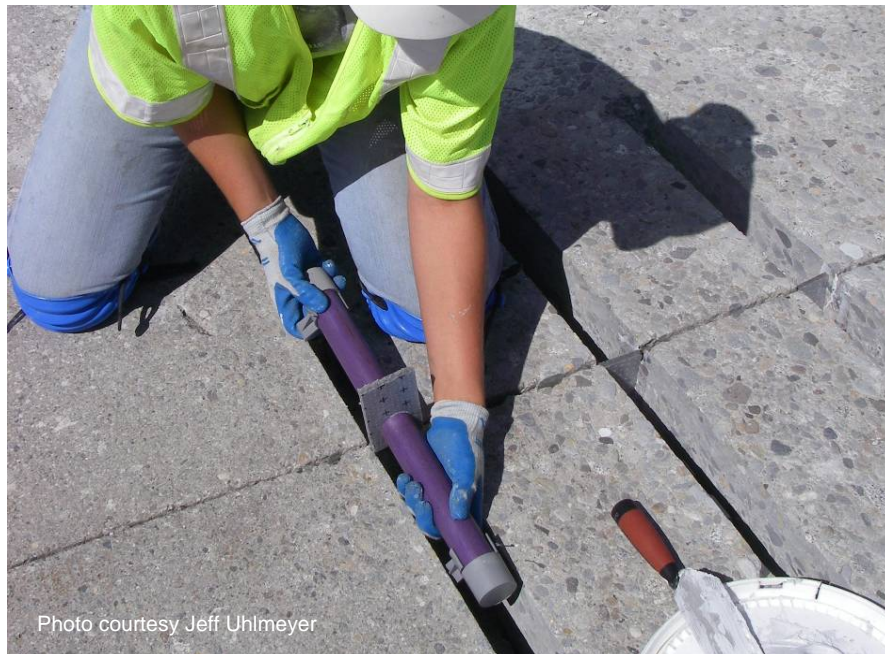
Figure 54 Inserting dowel bar retrofit assemblies into dowel bar slots.
