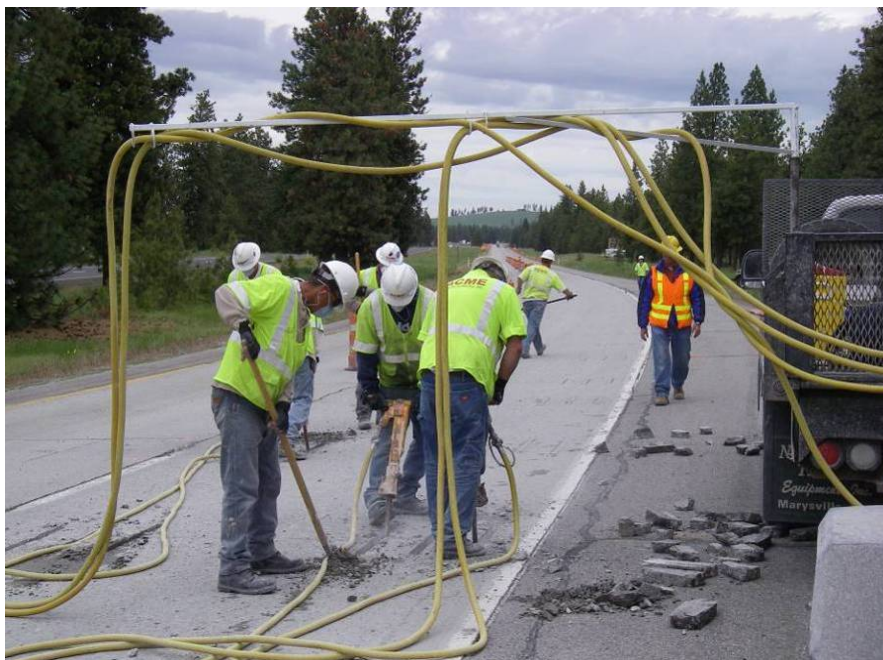
Figure 23 Jackhammer operation.
