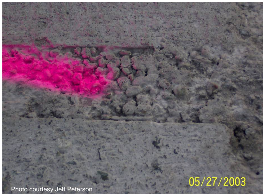
Figure 46 Insufficient consolidation of patching material.
