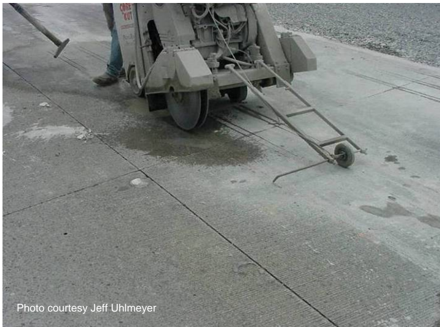
Figure 11 Cutting equipment for one dowel bar slot at a time.
