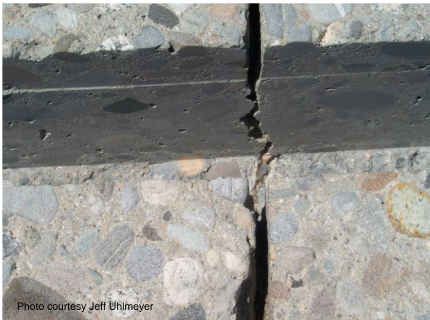
Figure 41 Cleaned dowel bar slot.
