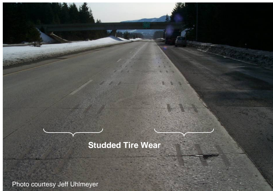
Figure 78 Wear due to studded tires.
