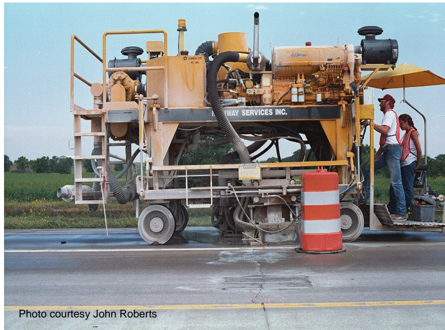
Figure 8 Cutting equipment for six dowel bar slots per joint.
