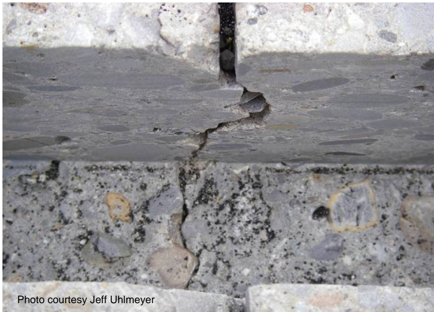
Figure 37 Dowel bar slot after shot blasting.
