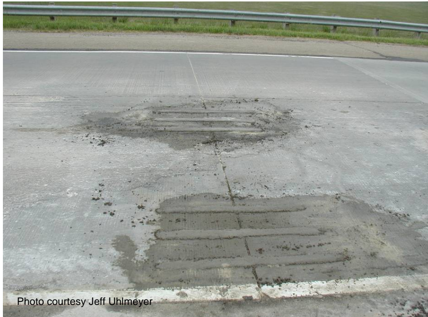
Figure 72 Patching material should be left high to prevent overworking
