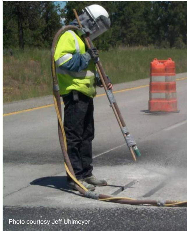
Figure 36 Cleaning dowel bar slot by shot blasting.
