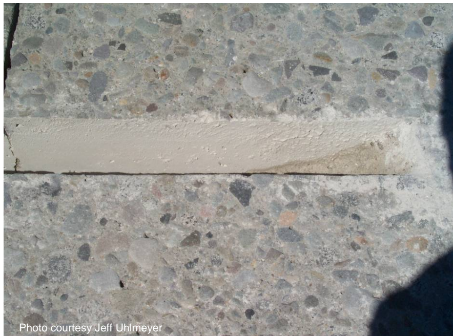
Figure 35 Sawcut blade residue on slot walls.
