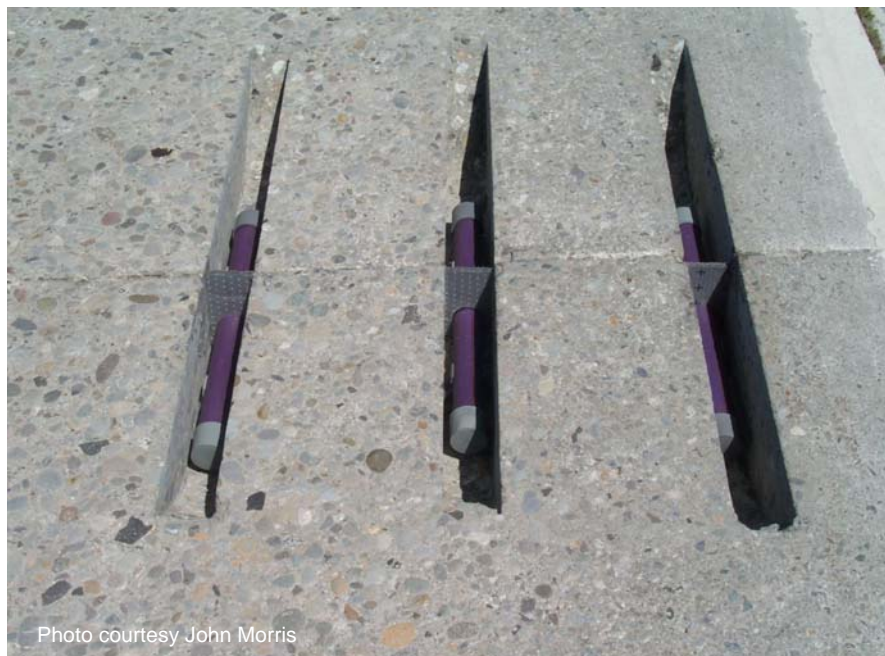
Figure 55 Dowel bar retrofit assembly at a transverse joint.
