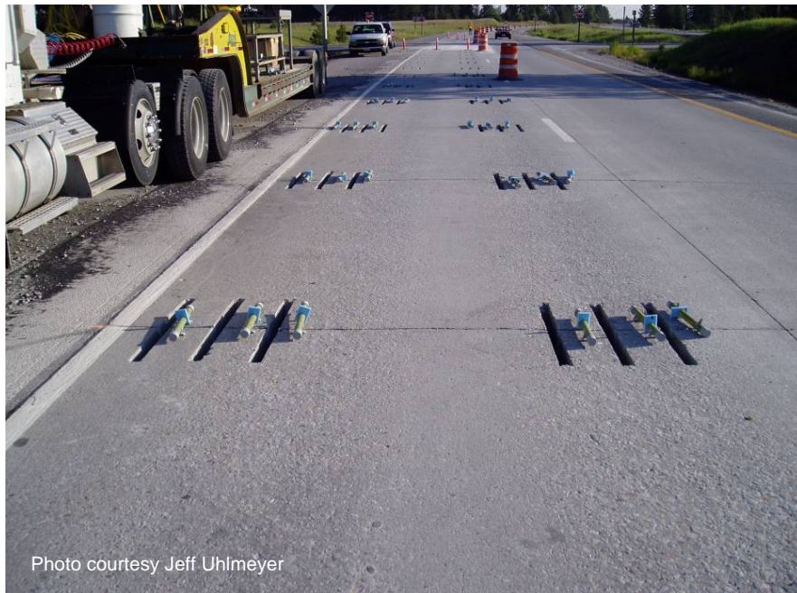
Figure 52 Dowel bar retrofit assemblies ready for installation.
