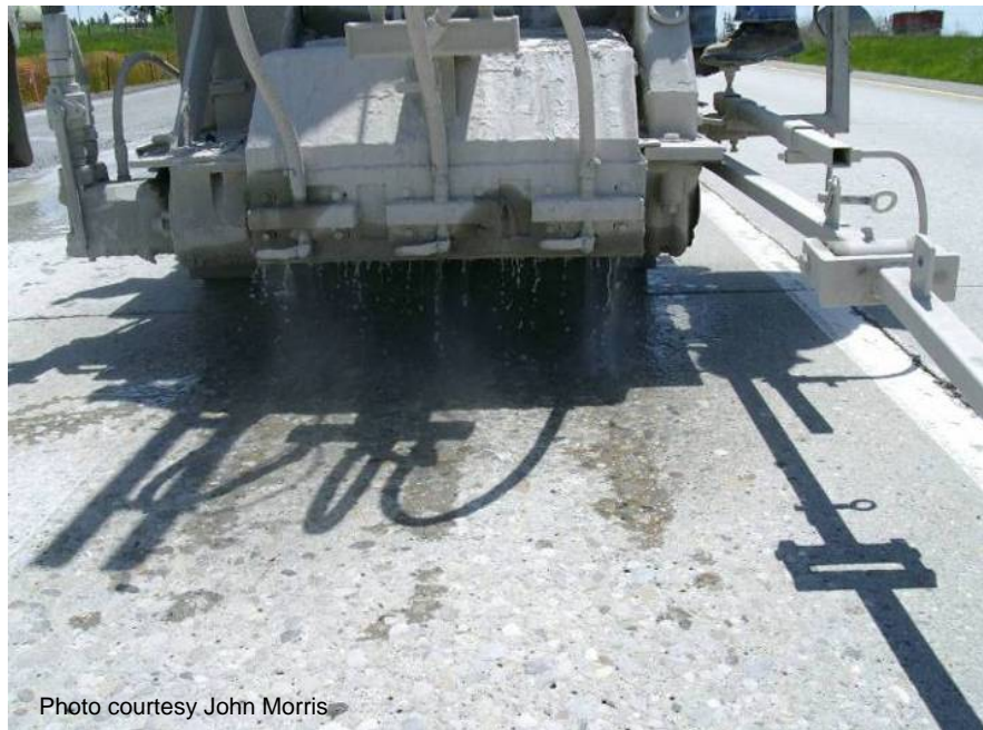
Figure 9 Cutting equipment for three dowel bar slots per wheelpath.
