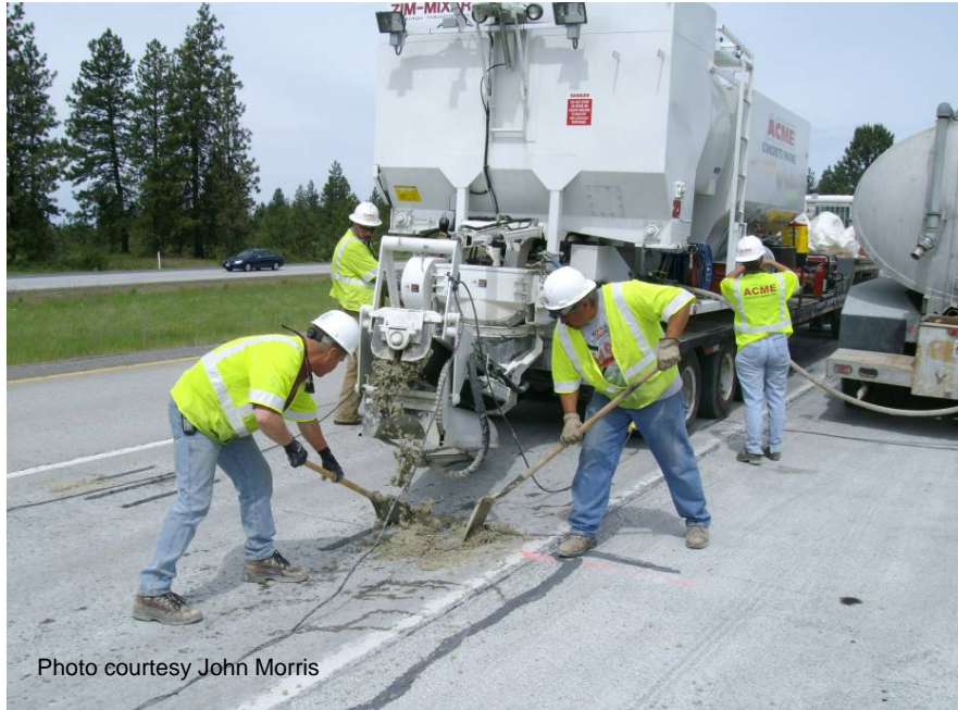
Figure 62 Placement of patching material.
