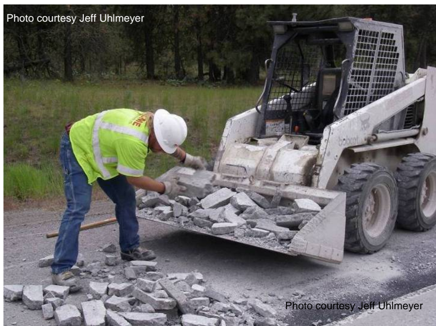
Figure 32 Debris removal.
