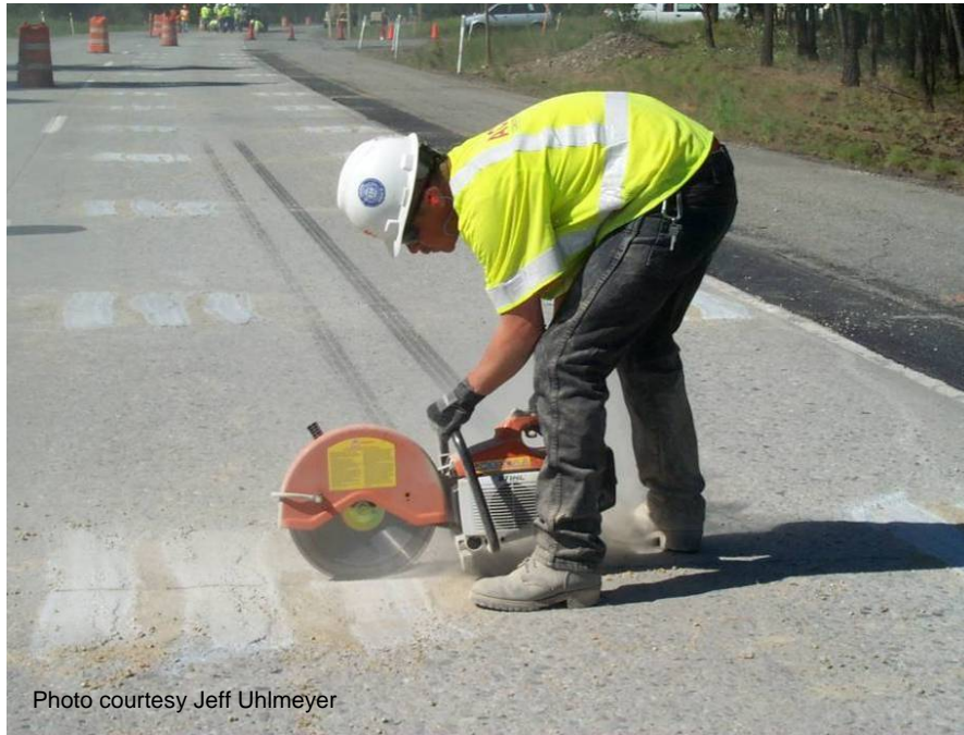
Figure 75 Establishing joint in patching material.
