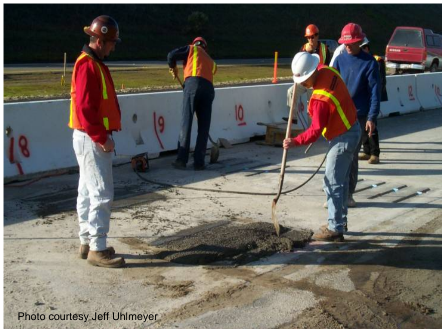
Figure 64 Moving patching material into dowel bar slots.
