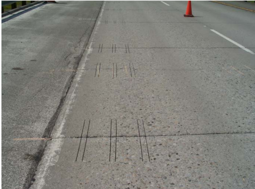
Figure 12 Cut dowel bar slots on non-skewed transverse joint.
