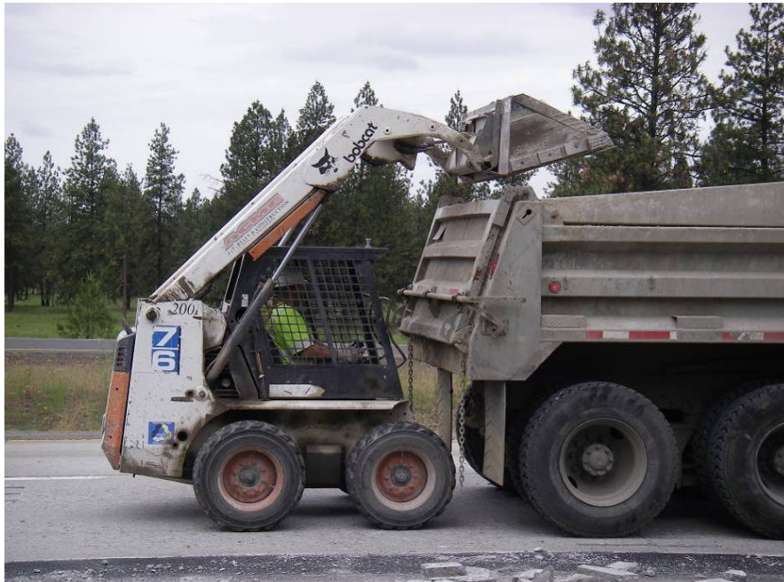
Figure 33 Loading debris into dump truck.
