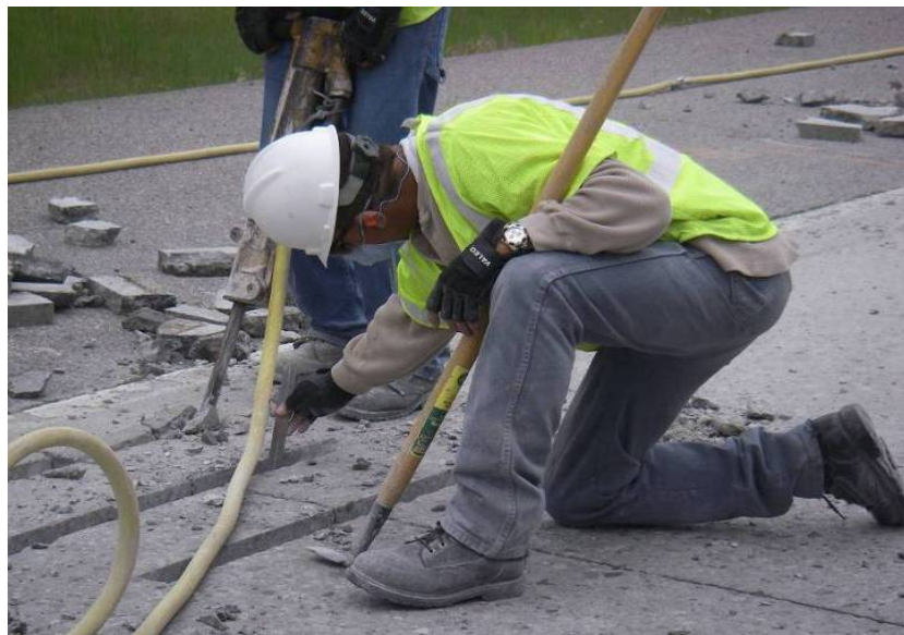
Figure 16 Check depth of dowel bar slot.
