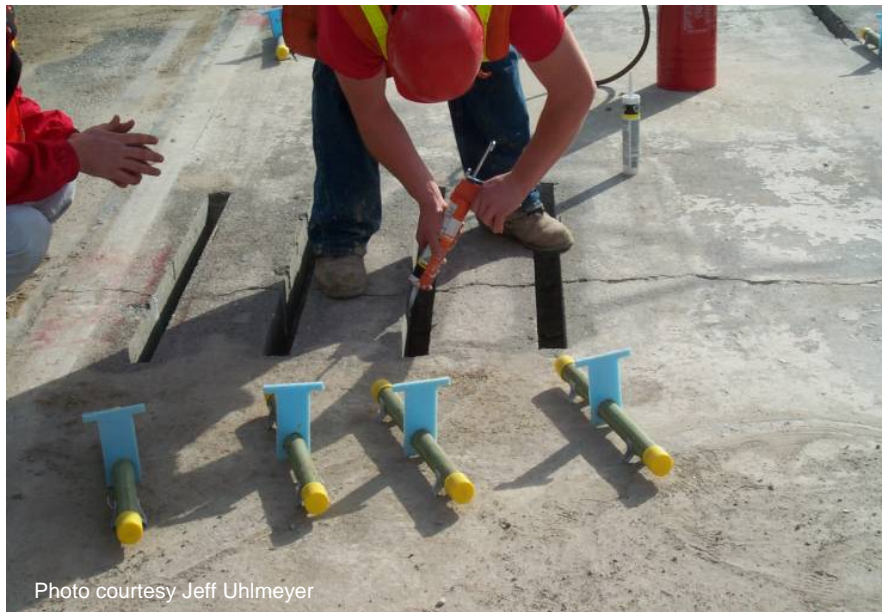
Figure 49 Caulking dowel bar slot sides and bottom.
