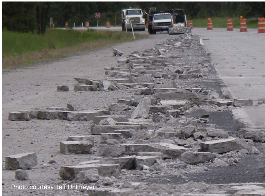
Figure 31 Debris from the jackhammering process.
