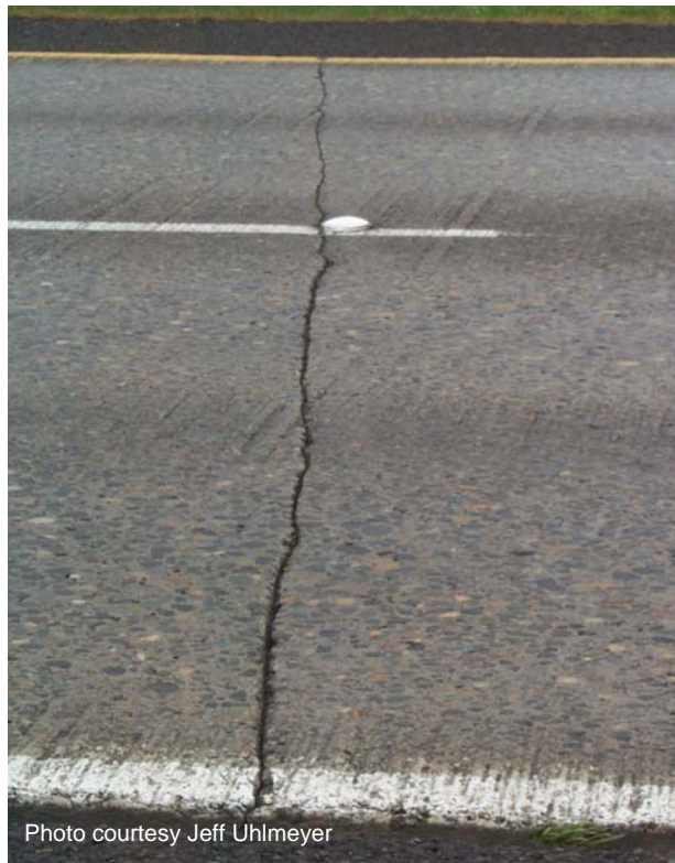
Figure 76 Transverse tape joint (original construction).
