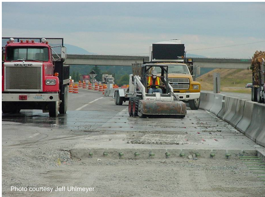
Figure 34 Sweeping debris from roadway.
