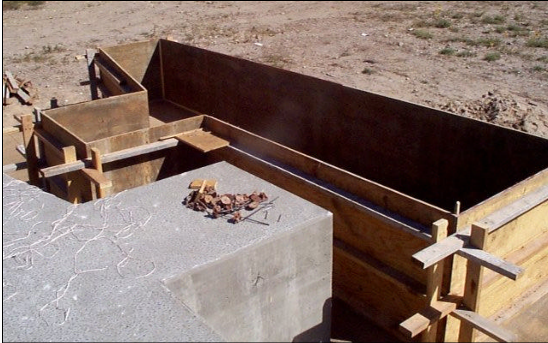
Figure 3.2 – Forms for new bent being cast on its side.
