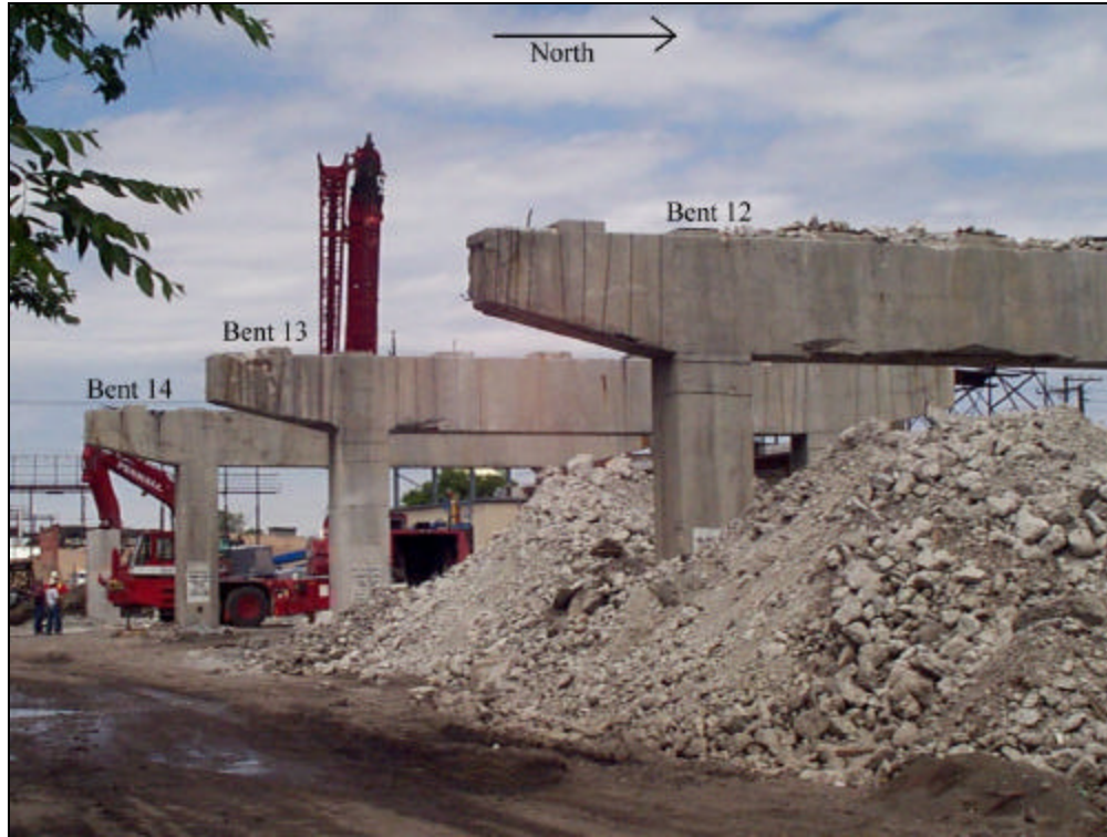
Figure 1.1 – Bent Caps 12, 13, and 14.
