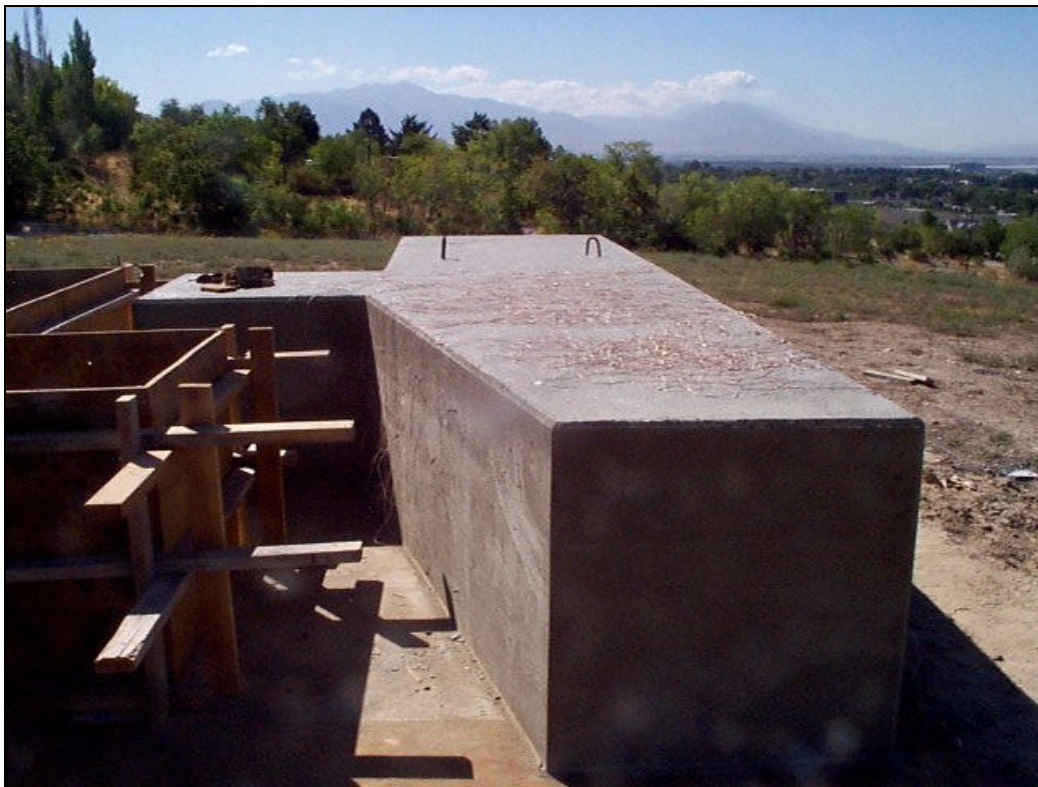
Figure 3.3 – New bent after removal of the forms.
