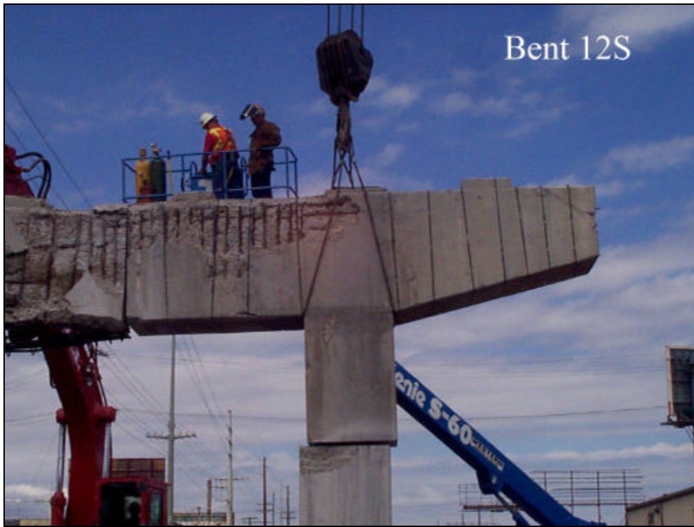
Figure 1.2 – Cantilever Portion of Bent 12.
