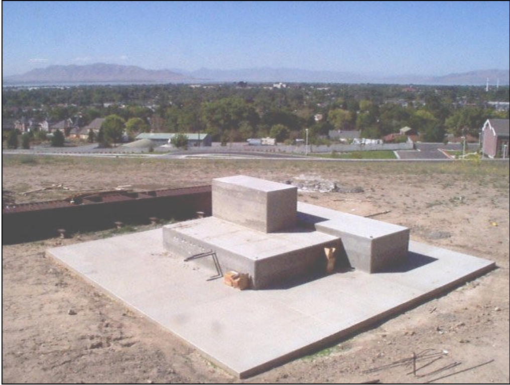
Figure 4.5 – Constructed test pad
