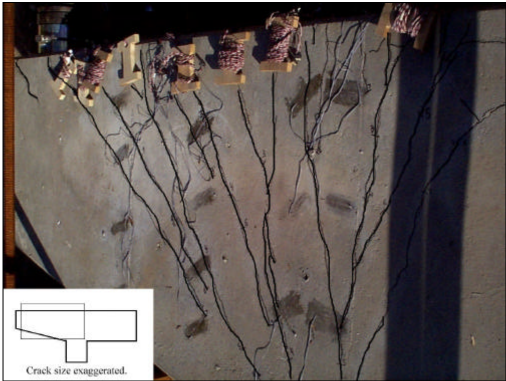
Figure 5.39 – Bent 1N, cracks on cycle 8.
