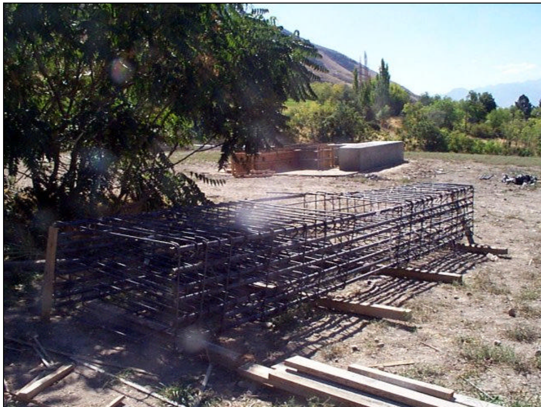
Figure 3.1 – Reinforcement cage for new bent.
