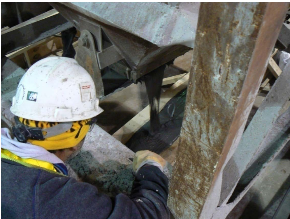
Figure 4.18. Beginning of first pour of UHPC units
