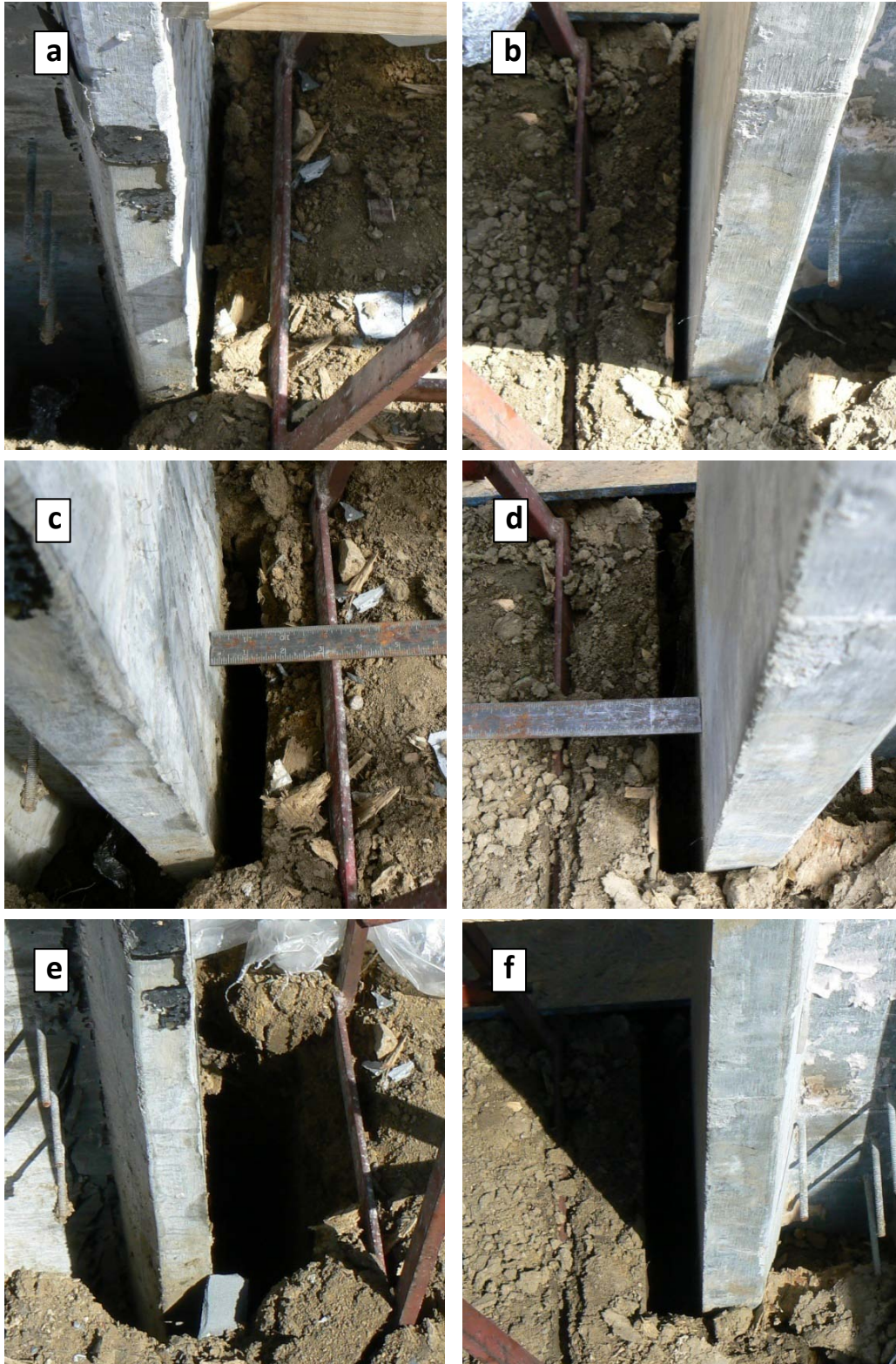
Figure 5.35. Soil gaps due to lateral pile movement next to a) P1 and b) P2 early in the test, c) P1 and d) P2 midway through the test, and e) P1 and f) P2 after the shear failure of pile P1
