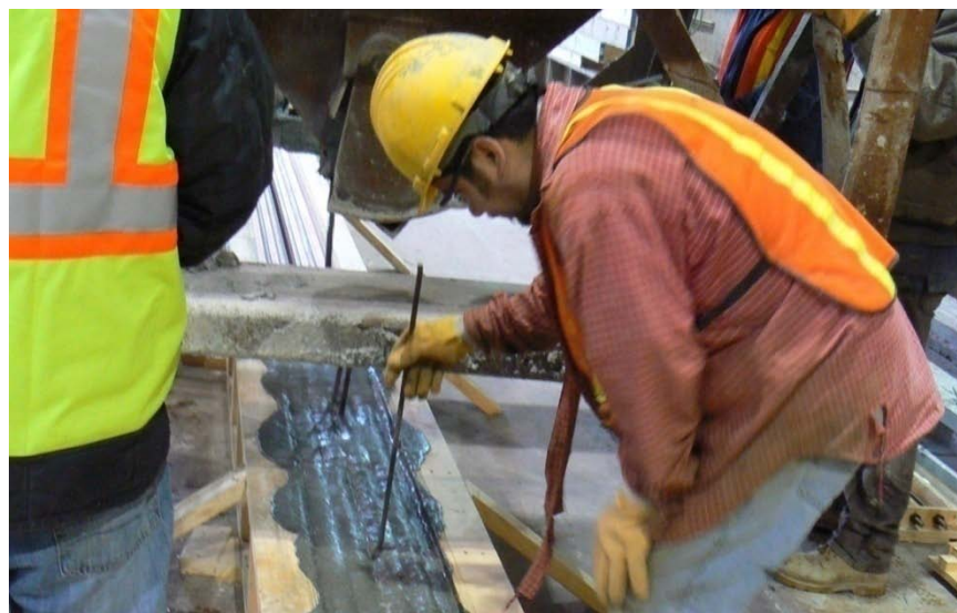
Figure 4.24. “Rodding” through the web of UHPC to eliminate formation of possible air pockets
