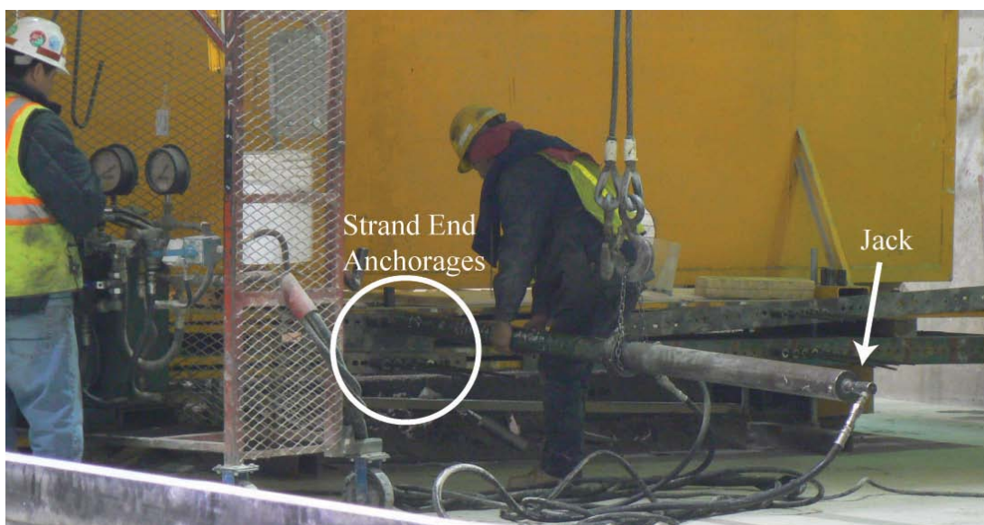
Figure 4.12. Stressing of prestressing strands for UHPC pile P1
