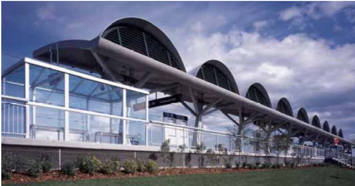
Figure 2.34. Shawnessy LRT station with UHPC canopies (Perry 2006)
