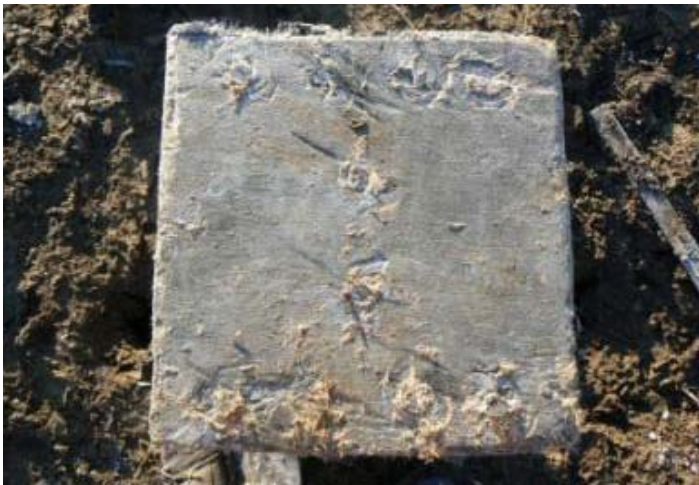
Figure 5.12. Condition of pile head at the end of driving pile P2
