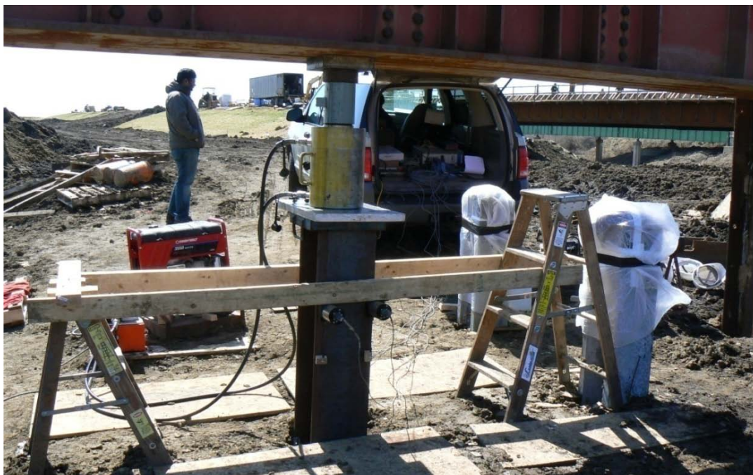
Figure 5.19. Wooden reference beams supported by ladders (steel pile)
