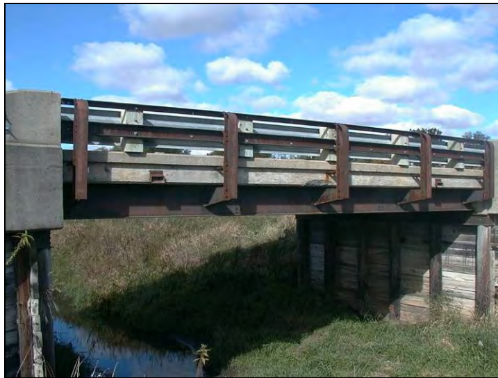
Figure 10.1. Side view of the bridge looking northwest (Bridge No. 094680 Carroll County – May 16 2006)
