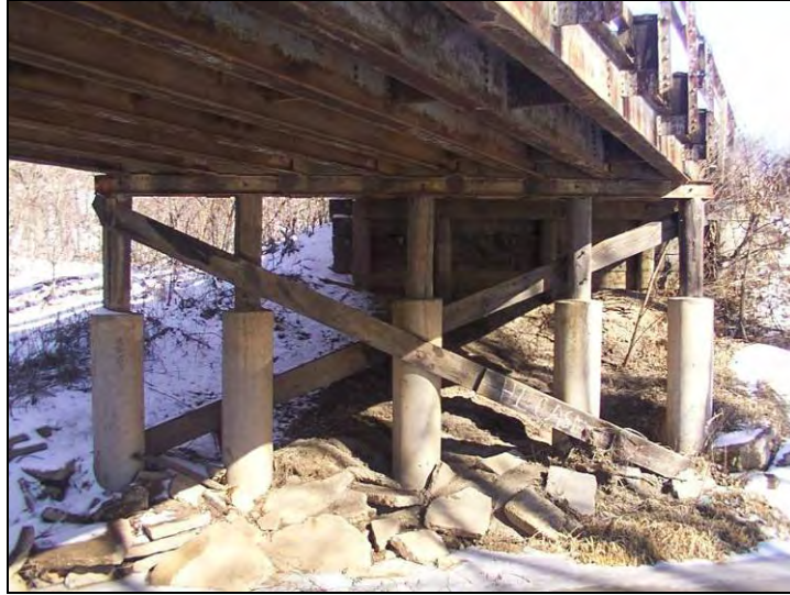
Figure 4.8. Encasing the center piers with concrete for pile restoration (Bridge No. 149 Boone County – February 11 2005)
