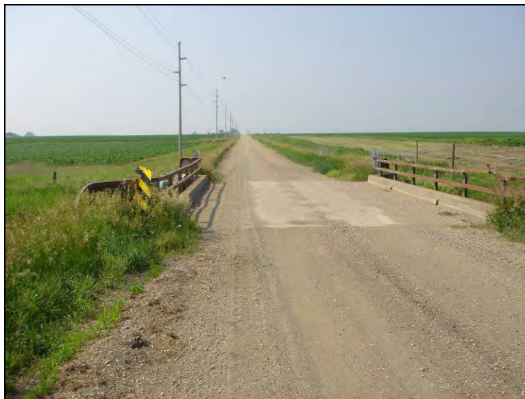
Figure 7.1. Bridge No. 7710 Boone County – looking south (June 24 2005)
