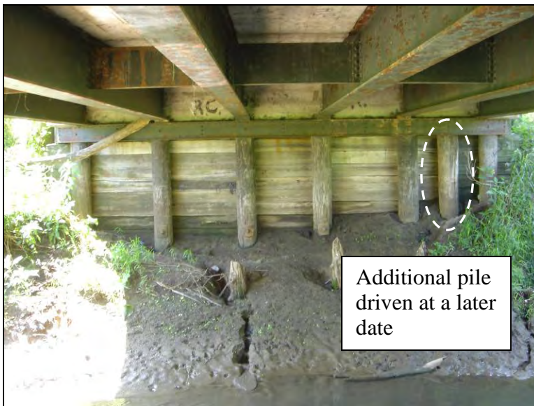
Figure 8.4. South abutment (Bridge No. 243470 Marshall County – July 22 2005)
