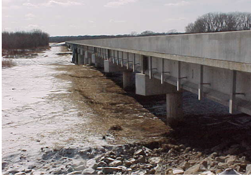
Figure 5.5 - Bridge A6031, Livingston County Rte. 36.
