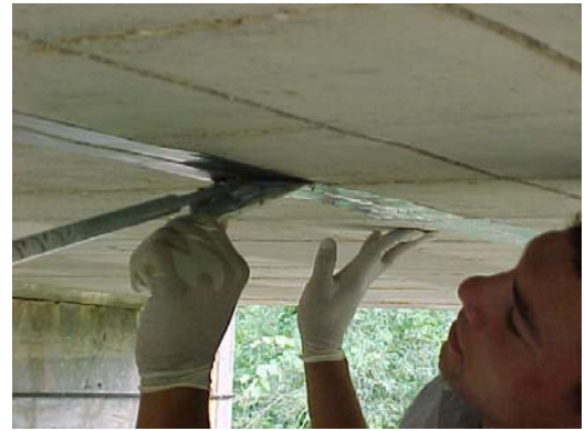
b) Inserting Epoxy Paste into the Groove
