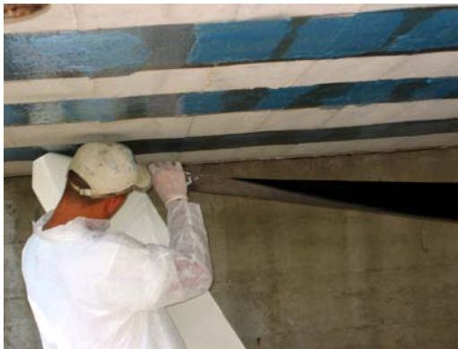
c) Application of CFRP Laminates
