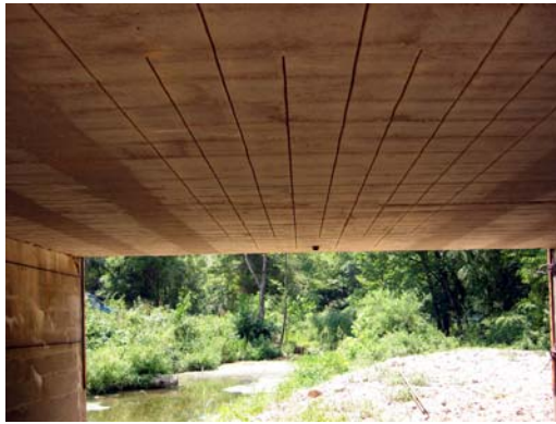
a) Grooves Prepared as per Design Geometry
