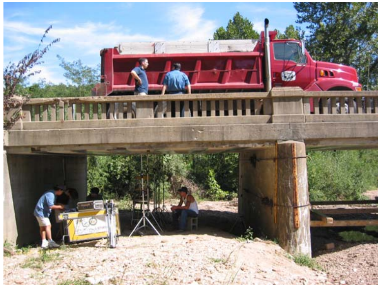
Figure 4-1 – Load Test with H20 Truck
