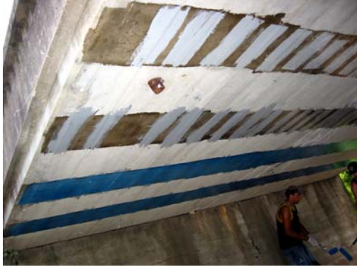
a) Surface Preparation with Primer and Putty
