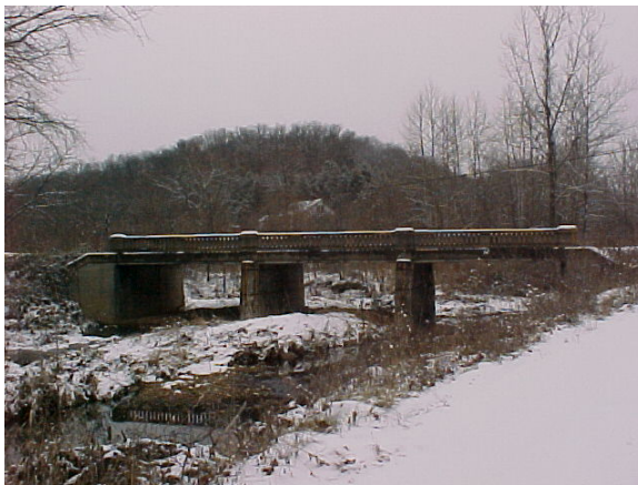
a) Side-view of the Bridge
