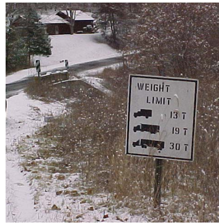
b) Load Posting Prior to Strengthening
