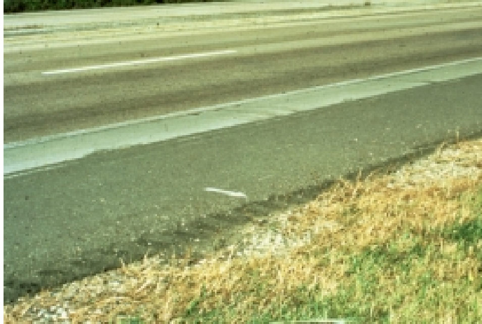
Figure 6.6. Painted arrow as a reference marker (Baumgardner, 2002).
