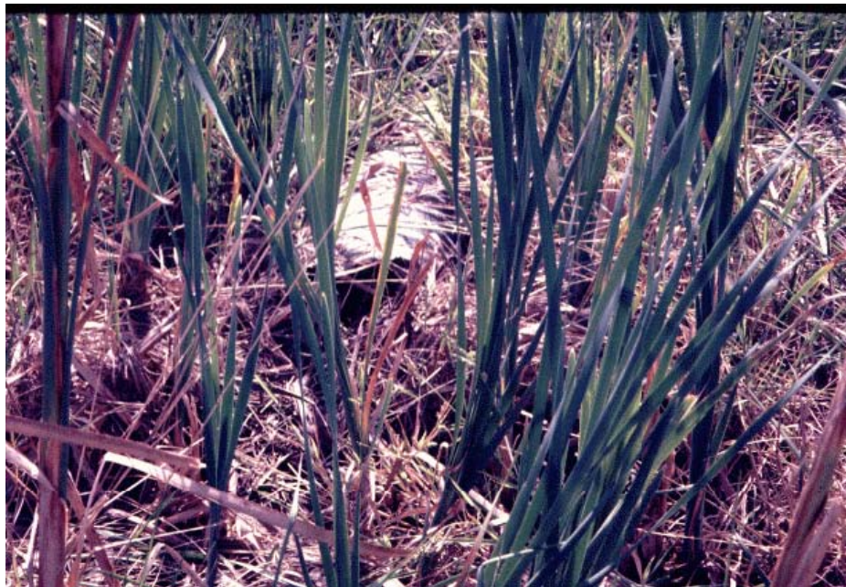
Figure 6.5. Hidden outlet pipe (Baumgardner, 2002).
