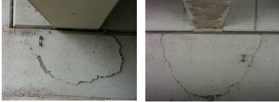
Figure 5-22. Abutment D-cracking
